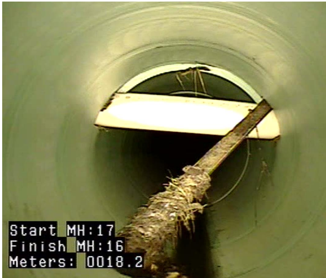
Figure 5-9: Second Pipe Intercepting the Storm Sewer on 1 st Ave N
