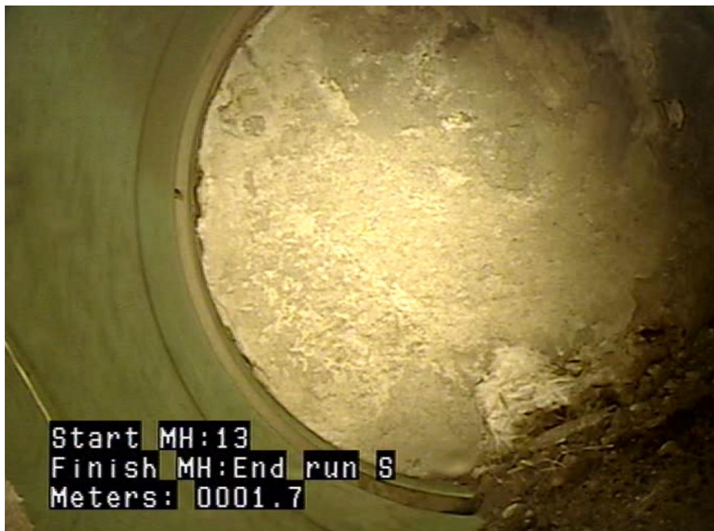
Figure 5-10: Concrete Blockage in the Storm Sewer Along 1 st St NE
