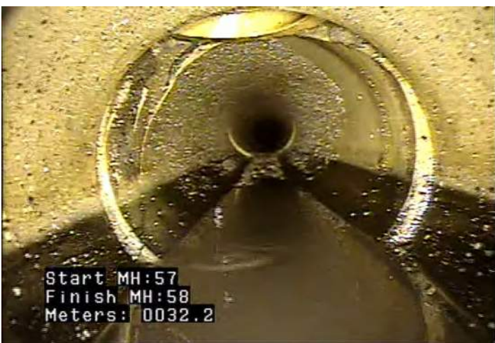
FM - Fracture Multiple @ 32.2 m.
