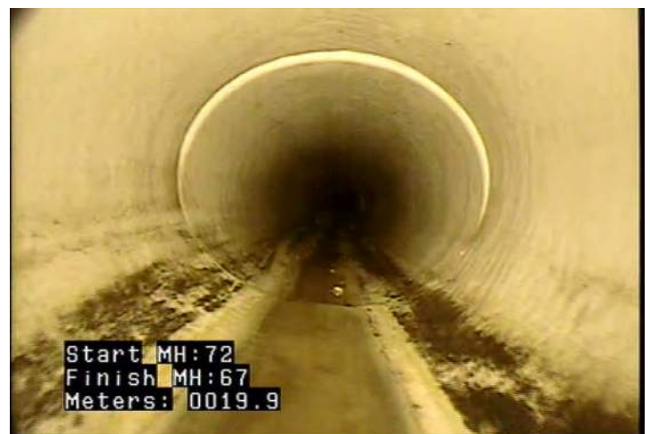
D - Pipe Deformed @ 19.9 m.
