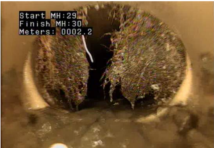
ID - Infiltration - Dripper @ 2.2 m.
