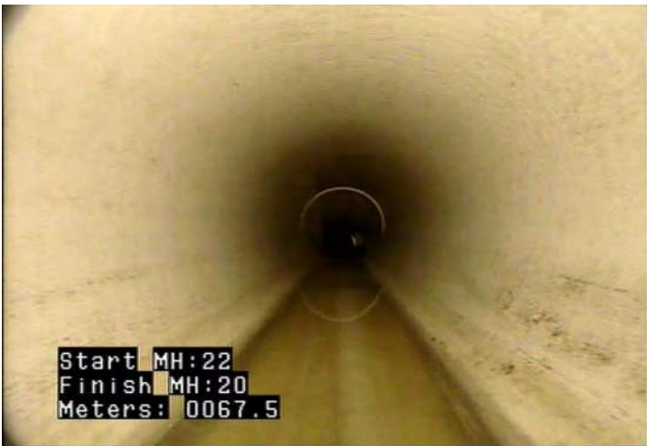
MWLS - Water Level: Sag @ 67.5 m.
