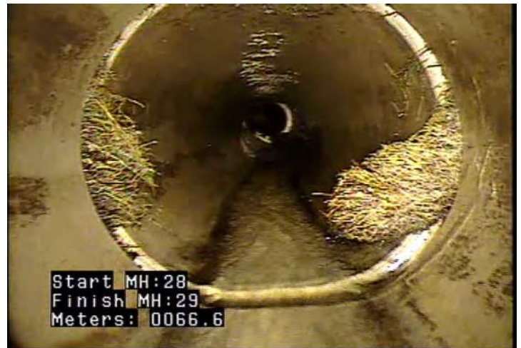
RMJ - Roots, Medium, Joint @ 66.6 m.
