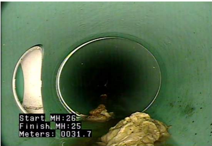
D - Pipe Deformed @ 31.7 m. Oval
