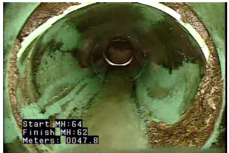
JSM - Joint Separated (open): Medium @ 47.8 m.
