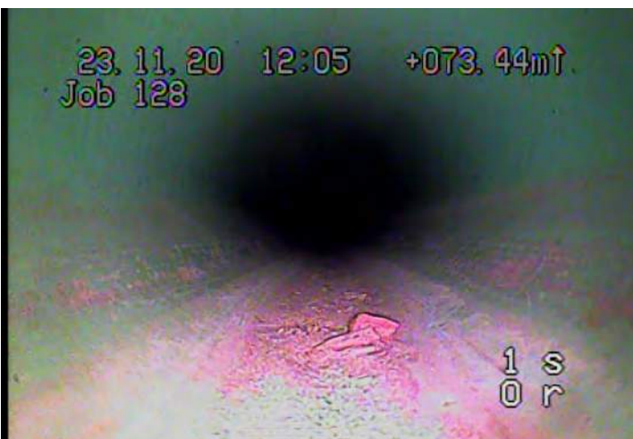
DSGV - Deposits Settled: Gravel @ 73.0 m.
