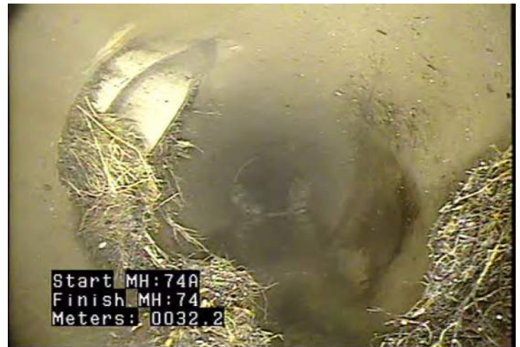
RMC - Roots, Medium: Connection @ 32.2 m.
