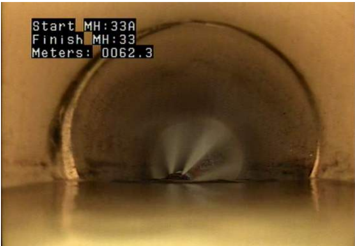
DAE - Deposits Attached: Encrustation @ 62.3 m.
