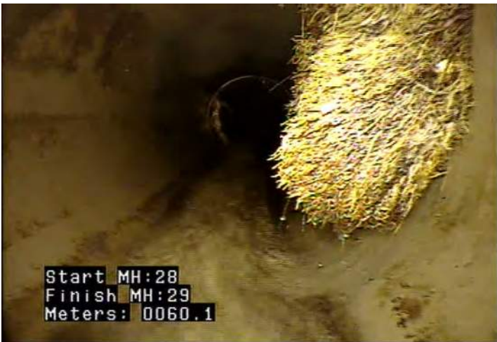
RMB - Roots, Medium: Barrel @ 60.1 m. Possible hole in pipe at this spot.
