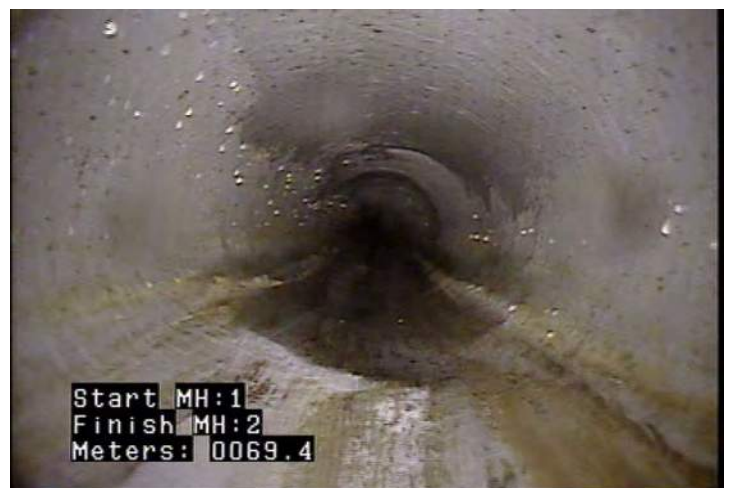
D - Pipe Deformed @ 69.4 m.
