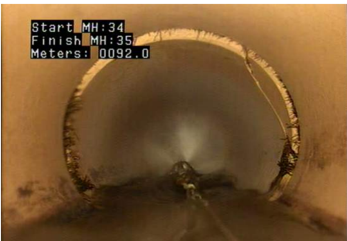
FC - Fracture Circumferential @ 92.0 m.
