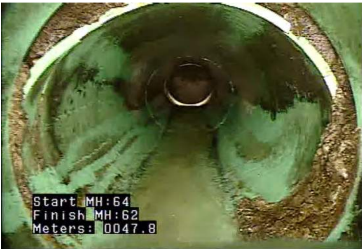
D - Pipe Deformed @ 47.8 m.
