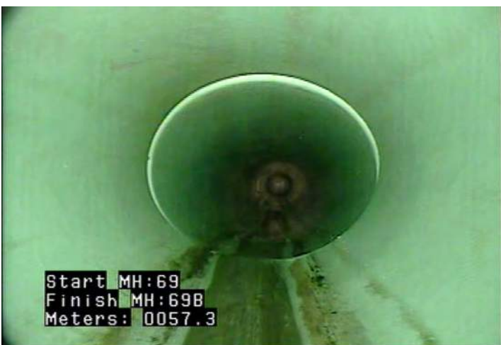
D - Pipe Deformed @ 57.3 m. Oval
