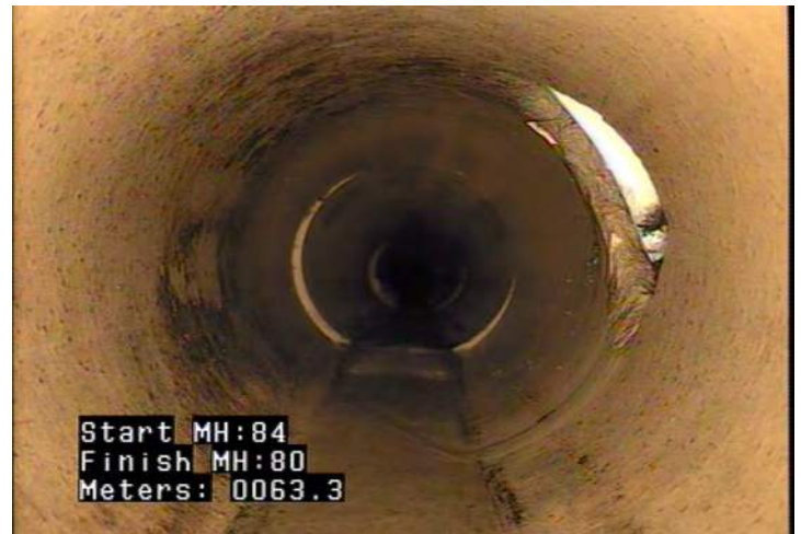
TB - Tap, Break-in / Hammer @ 63.3 m.
