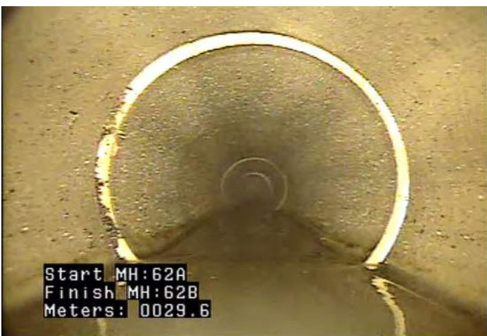
MWLS - Water Level: Sag @ 29.6 m.
