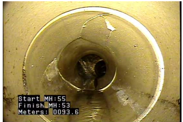
B - Pipe Broken @ 93.6 m.
