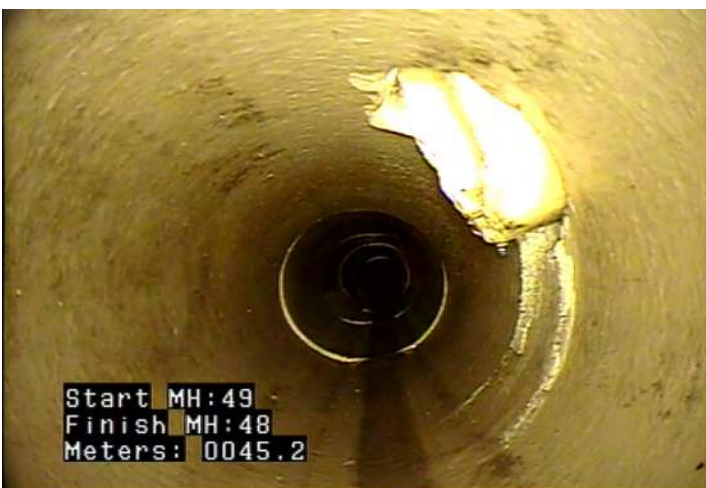
TBI - Tap, Break-in / Hammer: Intruding @ 45.2 m.
