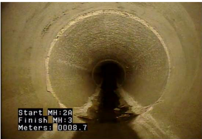
MGO - General Observation @ 8.9 m. Chipped joint 9:00
