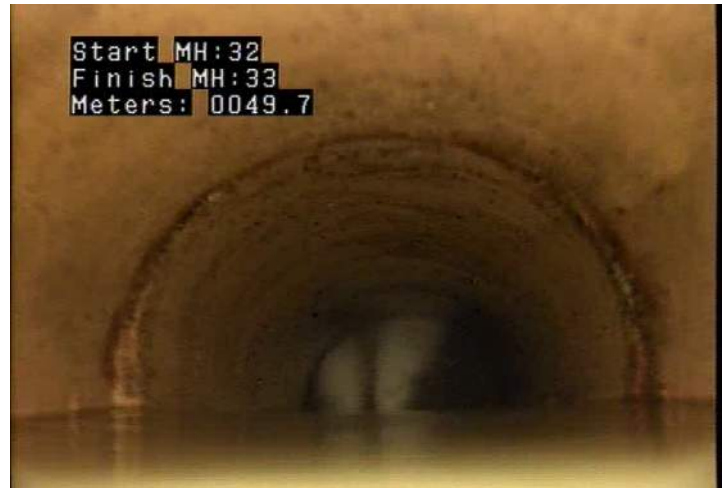
DAE - Deposits Attached: Encrustation @ 49.7 m.
