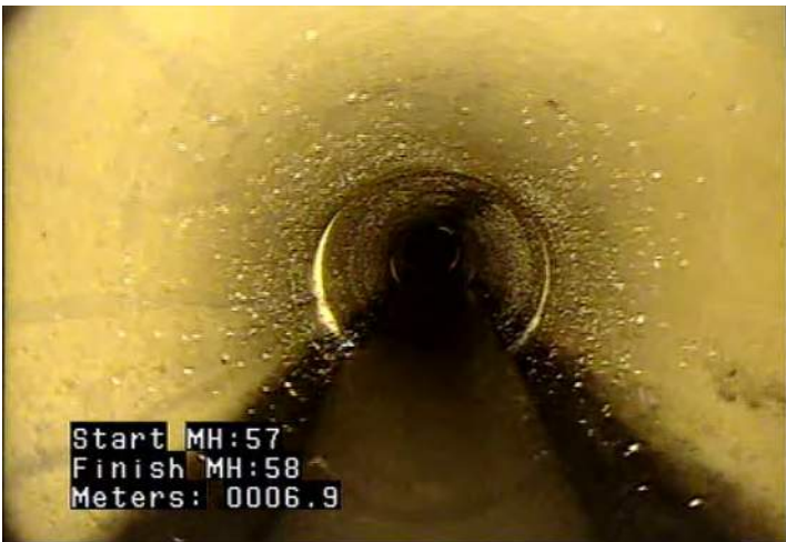
MWLS - Water Level: Sag @ 6.9 m.
