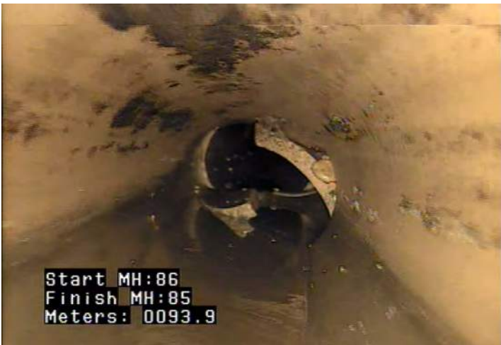
MWLS - Water Level: Sag @ 93.9 m.
