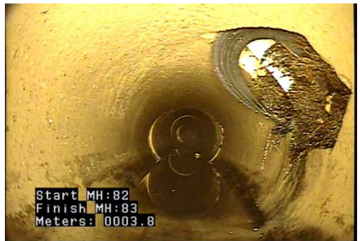
TBD - Tap, Break-in / Hammer: Defective @ 3.8 m. Gasket off
