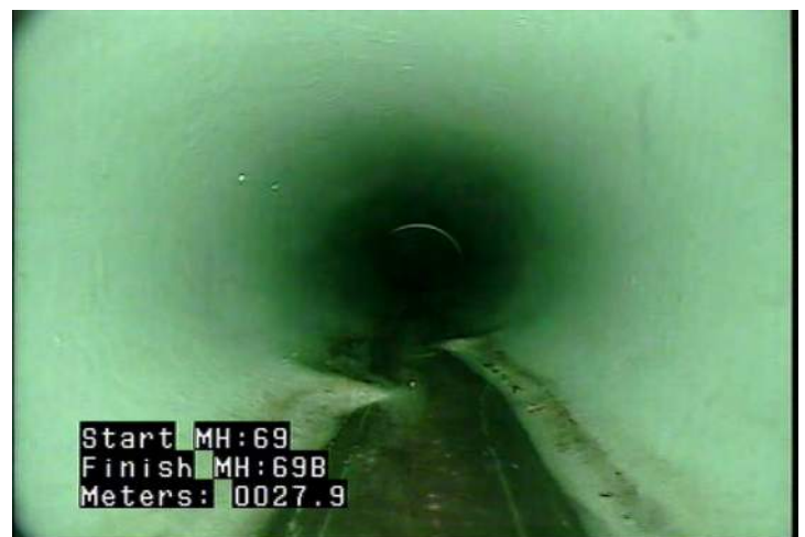
D - Pipe Deformed @ 27.9 m.
