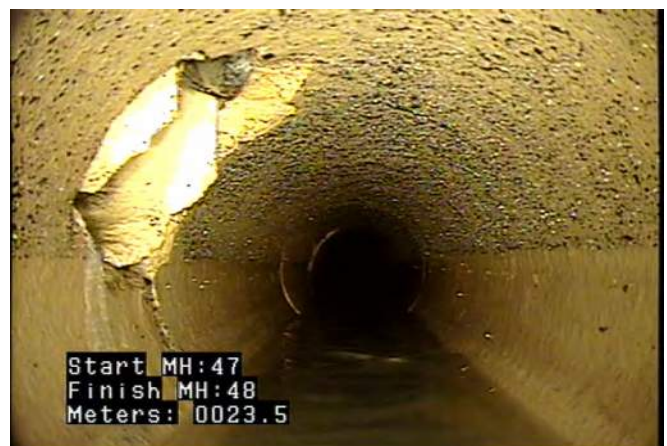
TBD - Tap, Break-in / Hammer: Defective @ 23.5 m. Plastic intruding from top of service.
