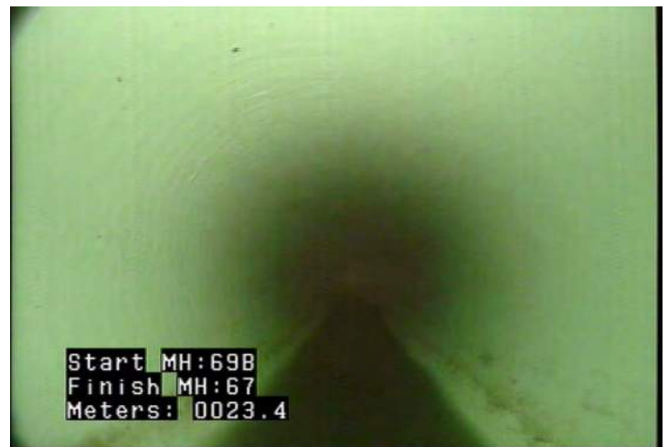
MWLS - Water Level: Sag @ 23.4 m.
