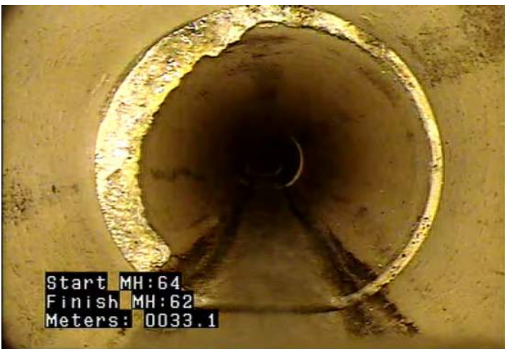
DAE - Deposits Attached: Encrustation @ 33.1 m.
