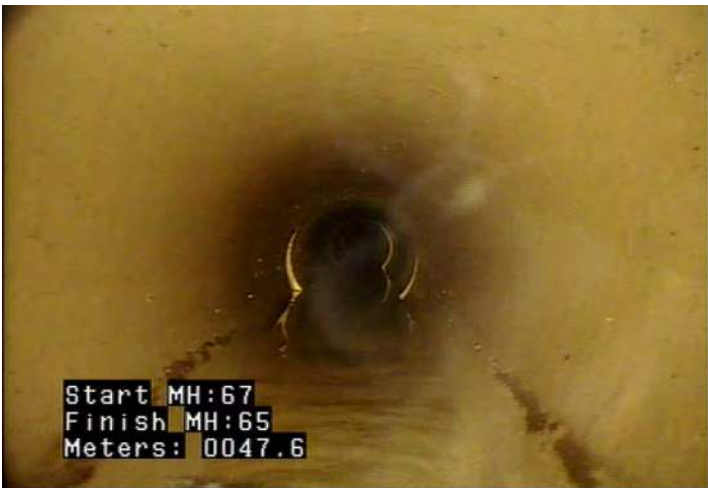
MWLS - Water Level: Sag @ 47.6 m.
