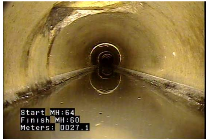
TB - Tap, Break-in / Hammer @ 27.1 m.
