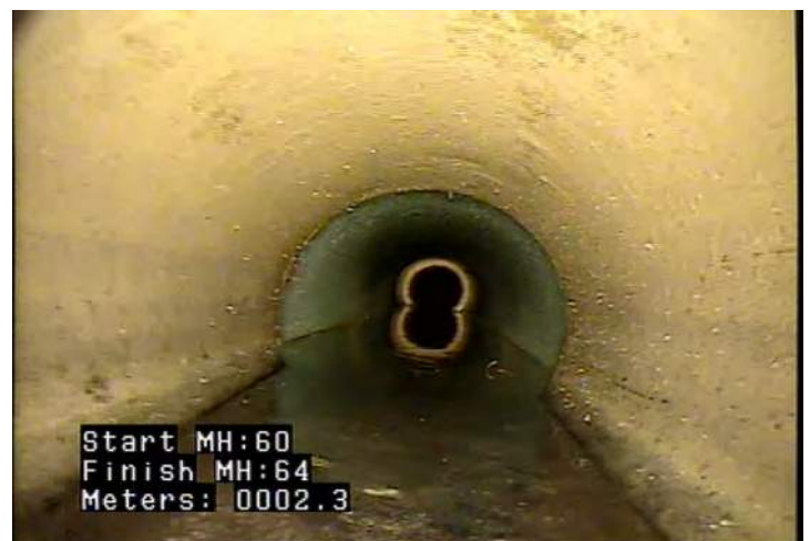
MWLS - Water Level: Sag @ 2.3 m.
