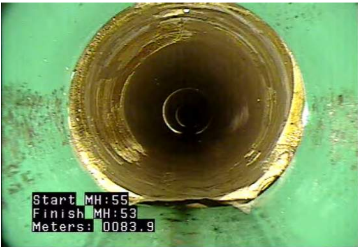
FS - Fracture Spiral @ 84.0 m.
