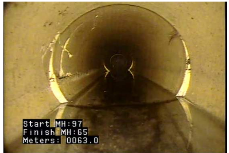
FM - Fracture Multiple @ 63.0 m.
