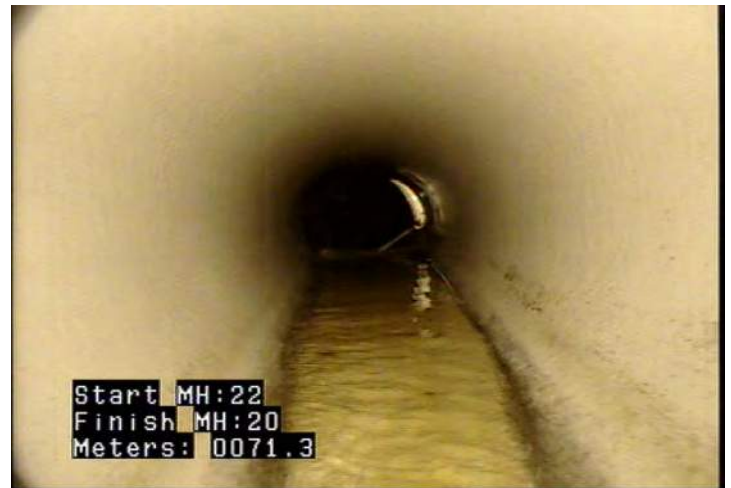
MWLS - Water Level: Sag @ 71.3 m.
