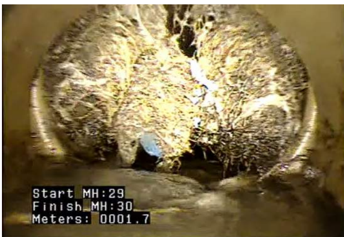
JOL - Joint Offset (displaced): Large @ 1.7 m.
