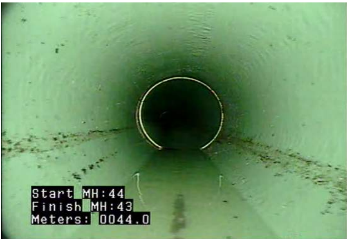
MWLS - Water Level: Sag @ 44.0 m.
