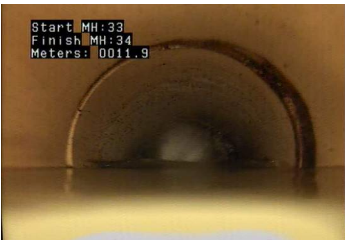
DAE - Deposits Attached: Encrustation @ 11.9 m.
