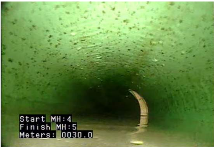
MWLS - Water Level: Sag @ 30.0 m.
