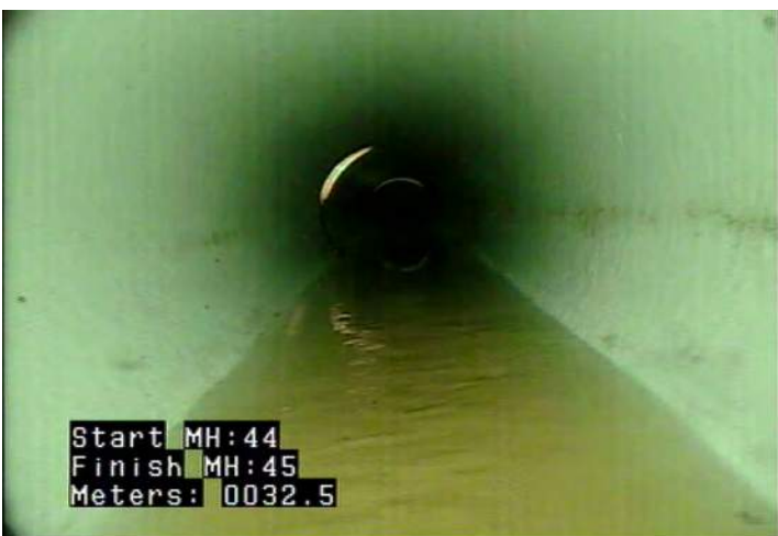
MWLS - Water Level: Sag @ 32.5 m.
