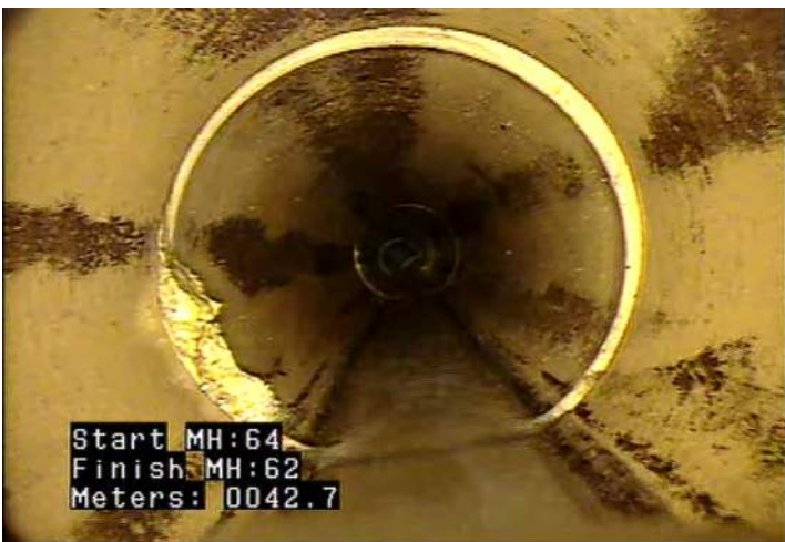
DAE - Deposits Attached: Encrustation @ 42.7 m.
