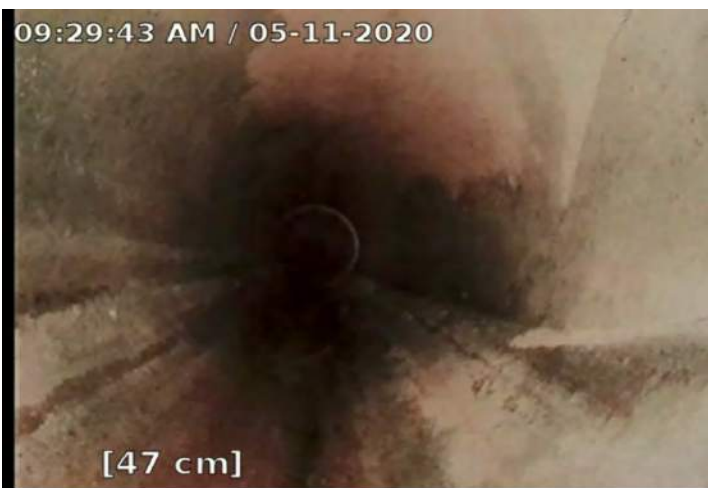
CC - Crack Circumferential @ 0.5 m.
