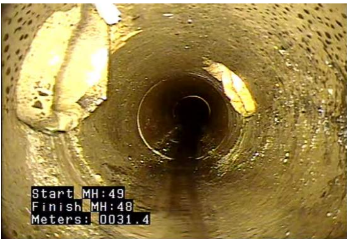
TBI - Tap, Break-in / Hammer: Intruding @ 31.4 m.
