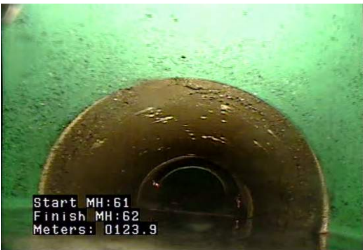
MMC - Material Change @ 123.9 m. PVC to Clay tile
