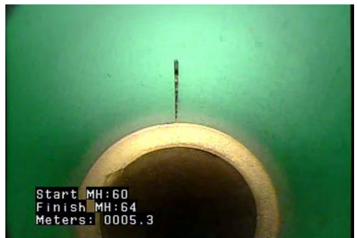
RPR - Point Repair - Pipe Replaced @ 2.6 m. PVC MSC - Dimension/Shape Change @ 5.3 m.
