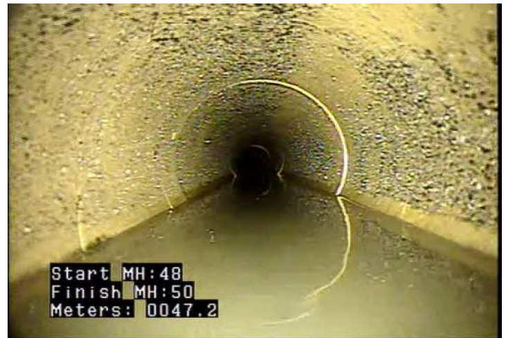
CM - Crack Multiple @ 47.2 m.
