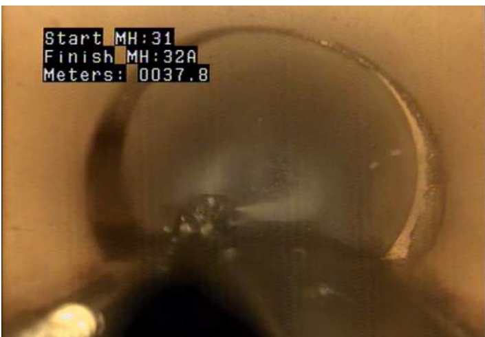
DAE - Deposits Attached: Encrustation @ 37.8 m.
