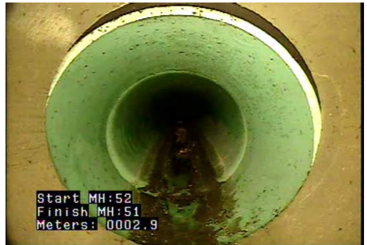
MMC - Material Change @ 2.9 m. Clay tile to PVC
