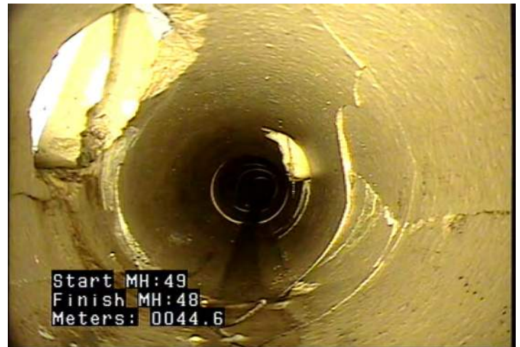
TB - Tap, Break-in / Hammer @ 44.6 m.
