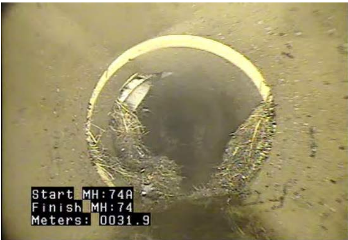
RMJ - Roots, Medium, Joint @ 31.9 m.
