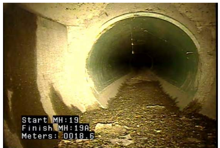
DSGV - Deposits Settled: Gravel @ 18.6 m.
