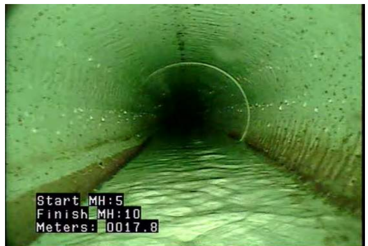
MWLS - Water Level: Sag @ 17.8 m.
