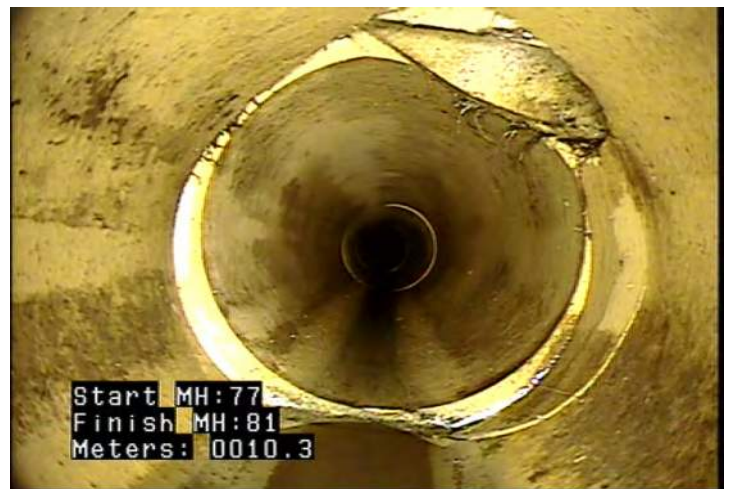
FS - Fracture Spiral @ 10.4 m.
