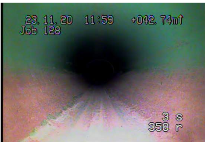
DSGV - Deposits Settled: Gravel @ 41.1 m.
