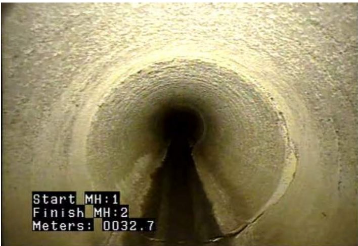
MGO - General Observation @ 32.7 m. Chip at joint
