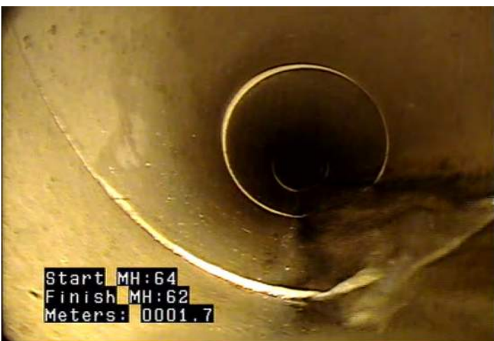
FC - Fracture Circumferential @ 0.5 m.
