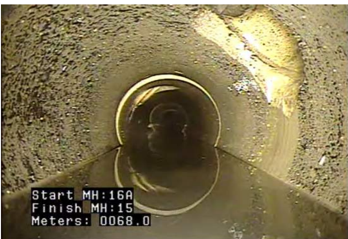
TB - Tap, Break-in / Hammer @ 68.0 m.
