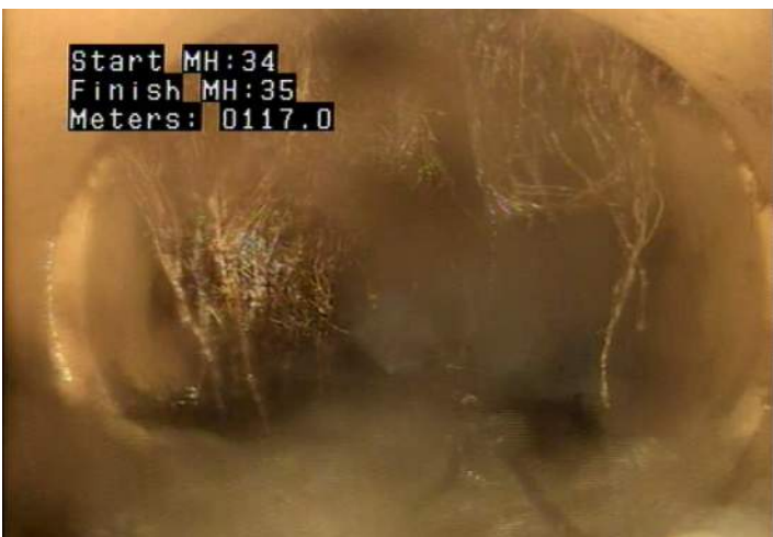
RMJ - Roots, Medium, Joint @ 117.0 m.
