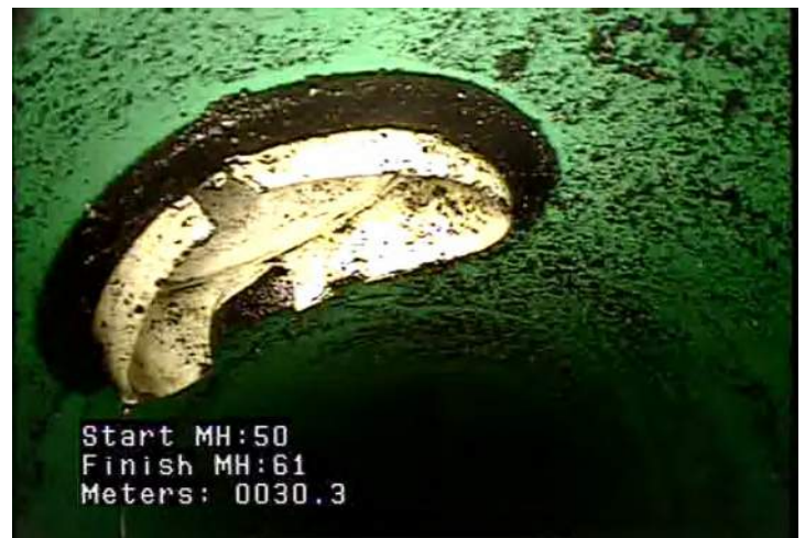
TSD - Tap, Saddle: Defective @ 30.3 m. Chipped
