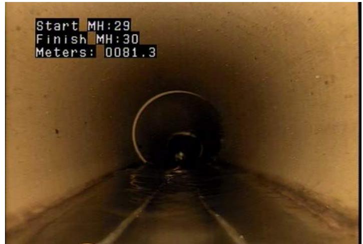
MWLS - Water Level: Sag @ 81.3 m.
