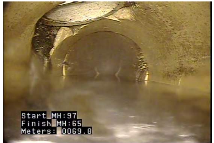
H - Hole in Pipe @ 69.8 m. Under service.
