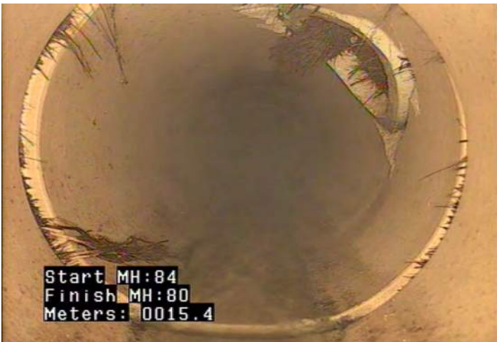
TBD - Tap, Break-in / Hammer: Defective @ 15.4 m. Roots
