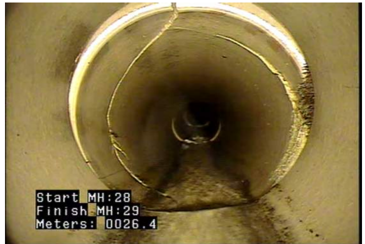
FM - Fracture Multiple @ 26.4 m.
