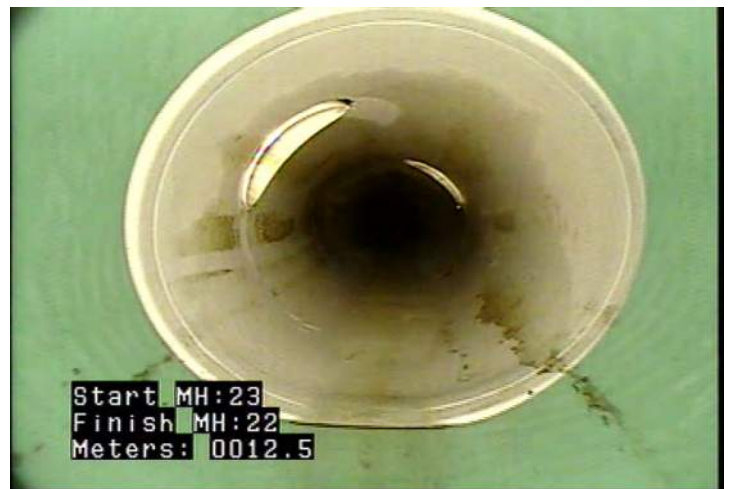
MMC - Material Change @ 12.5 m. Blue to White PVC
