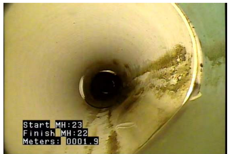
MMC - Material Change @ 1.9 m. Blue to White PVC
