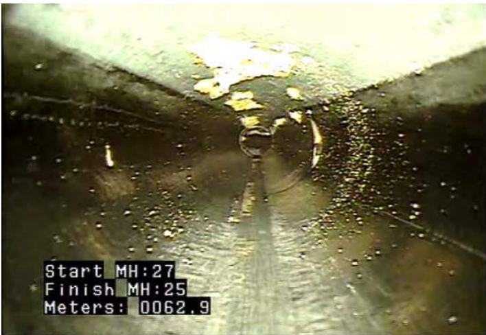
DAGS - Deposits Attached: Grease @ 62.9 m.
