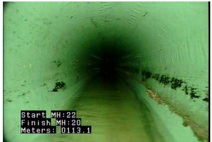
MWLS - Water Level: Sag @ 113.1 m.
