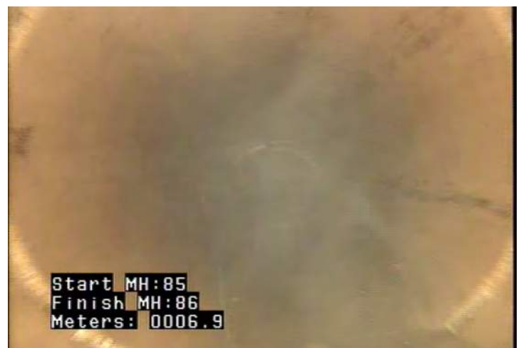
MWLS - Water Level: Sag @ 6.9 m.
