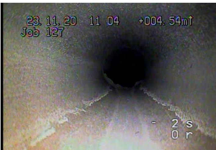
ISGT - Intruding Seal Material - Grout @ 2.9 m.
