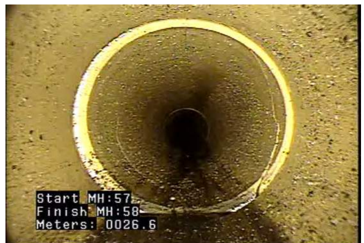
FM - Fracture Multiple @ 26.6 m.
