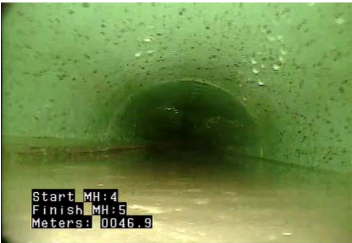
MWLS - Water Level: Sag @ 46.9 m.
