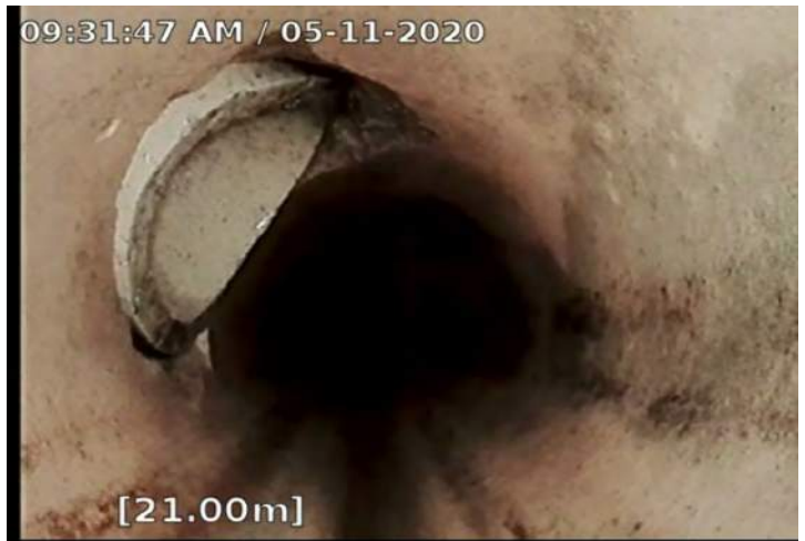
TB - Tap, Break-in / Hammer @ 21.0 m.
