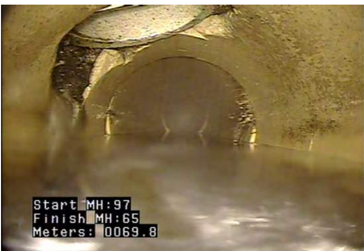
TB - Tap, Break-in / Hammer @ 69.8 m.
