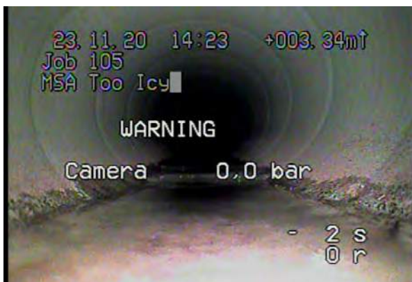
MSA - Survey Abandoned @ 3.3 m. Unable to crawl due to icy conditions. Unable to go downstream due to ST MH 16 being buried.
