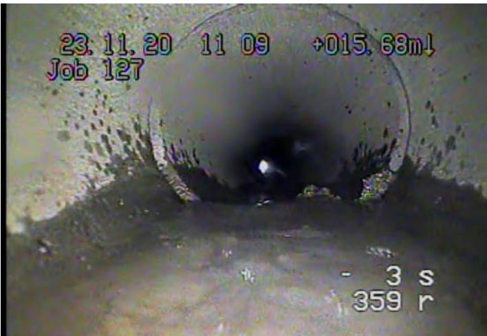
ISGT - Intruding Seal Material - Grout @ 17.1 m.
