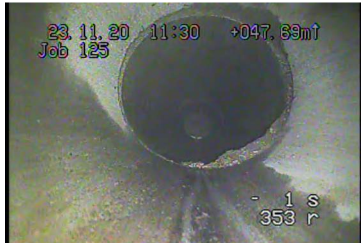
ISGT - Intruding Seal Material - Grout @ 47.9 m.
