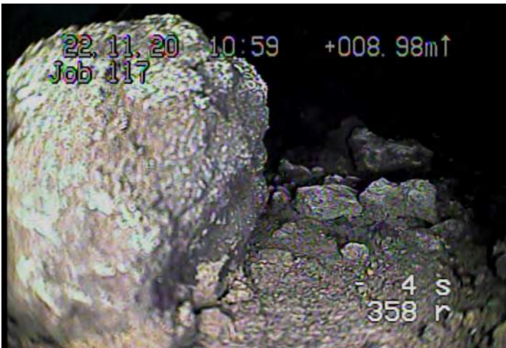
DNGV - Deposits Ingress: Gravel @ 8.9 m.
