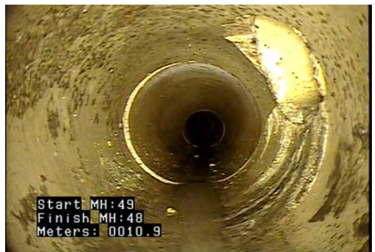
TB - Tap, Break-in / Hammer @ 10.9 m.
