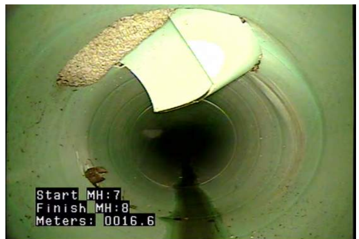
TBI - Tap, Break-in / Hammer: Intruding @ 16.6 m.
