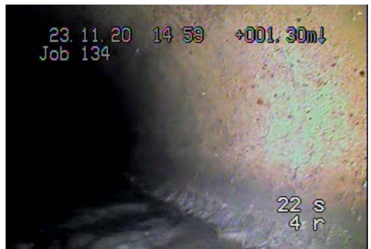
MSA - Survey Abandoned @ 1.0 m. Unable to pass gravel in line.
