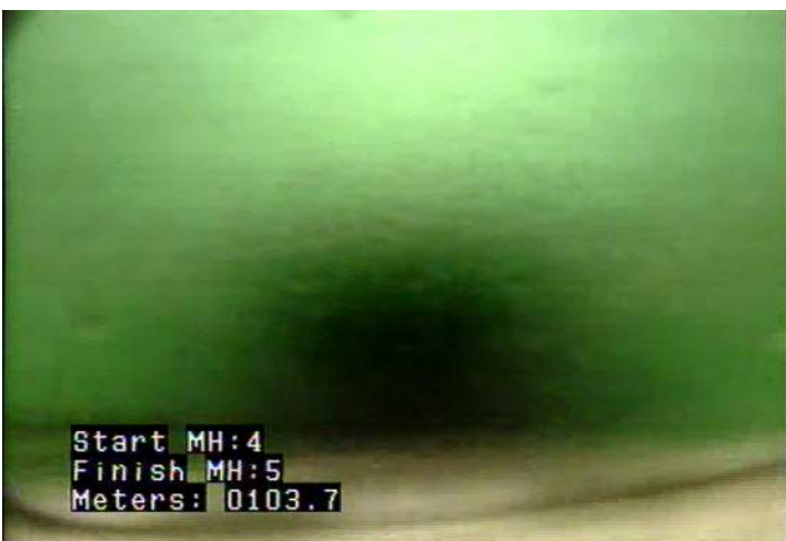
MWLS - Water Level: Sag @ 103.7 m.
