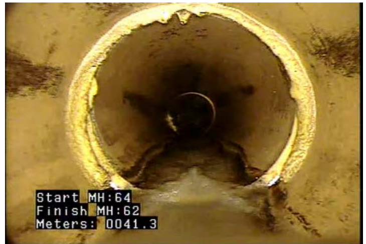
DAE - Deposits Attached: Encrustation @ 41.3 m.
