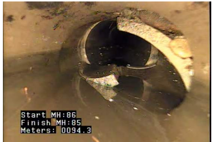
BSV - Pipe Broken: Soil Visible @ 94.4 m.
