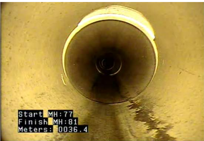
H - Hole in Pipe @ 36.4 m. Piece of pipe missing at joint, ground visible, roots
