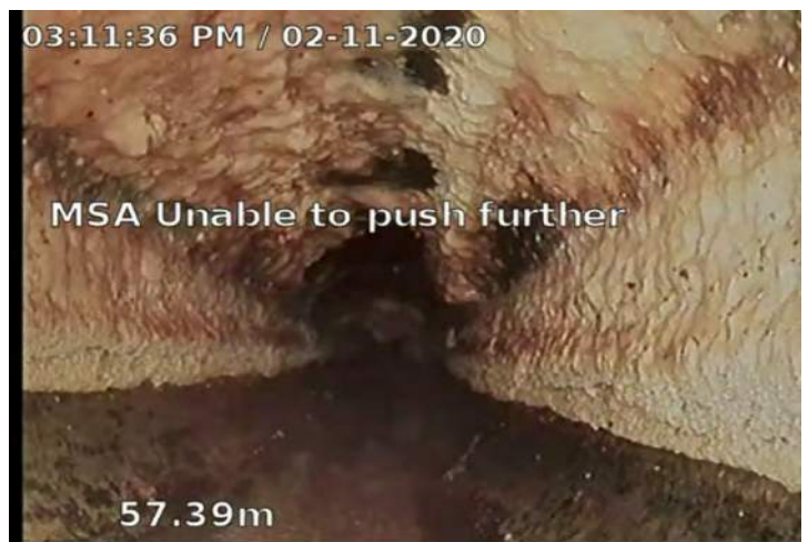
DAGS - Deposits Attached: Grease @ 57.4 m.
