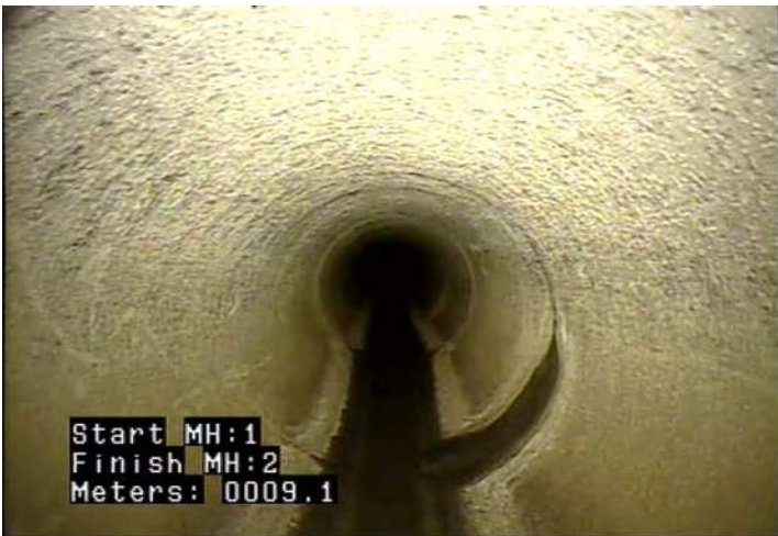
IS - Infiltration - Stain @ 9.1 m.
