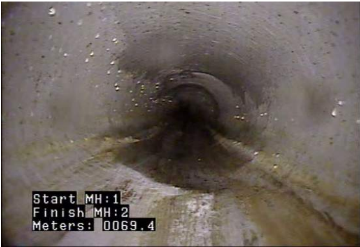
D - Pipe Deformed @ 75.1 m.
