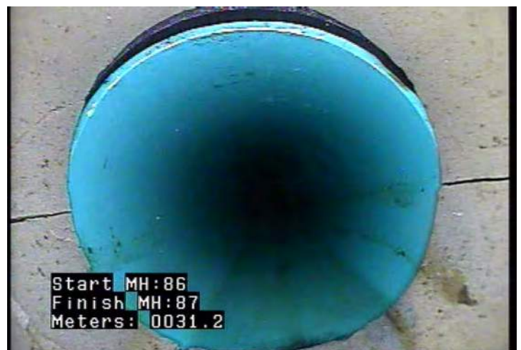
RPR - Point Repair - Pipe Replaced @ 31.2 m. PVC Repair
