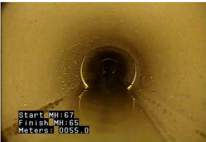
MWLS - Water Level: Sag @ 55.0 m.
