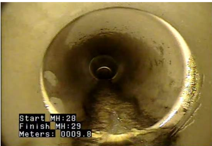
DAE - Deposits Attached: Encrustation @ 9.8 m.
