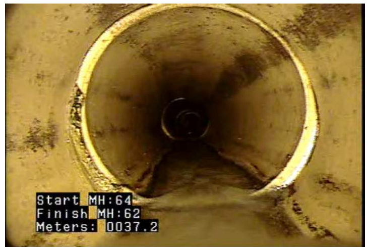
DAE - Deposits Attached: Encrustation @ 37.2 m.
