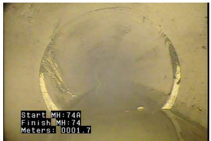
RFJ - Roots, Fine: Joint @ 1.7 m. Fine roots at most joints
