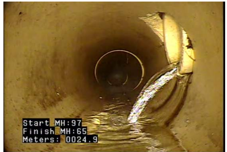
TBA - Tap, Break-in / Hammer: Active @ 24.9 m.
