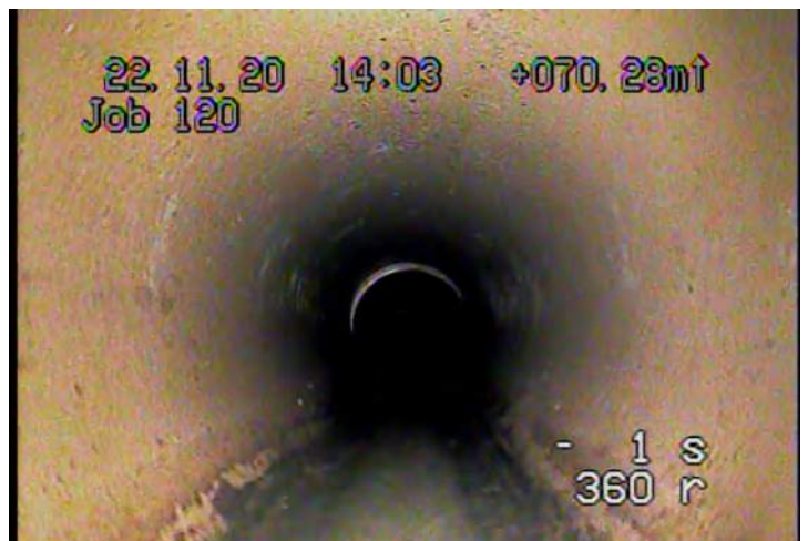
MSA - Survey Abandoned @ 70.3 m. Unable to crawl over joint.
