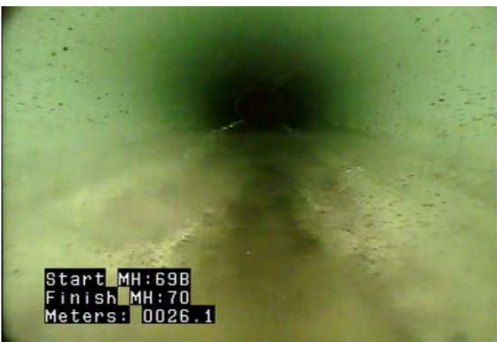
MWLS - Water Level: Sag @ 26.1 m.
