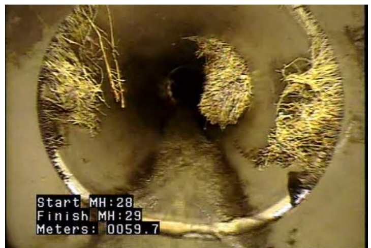
RMJ - Roots, Medium, Joint @ 59.7 m.
