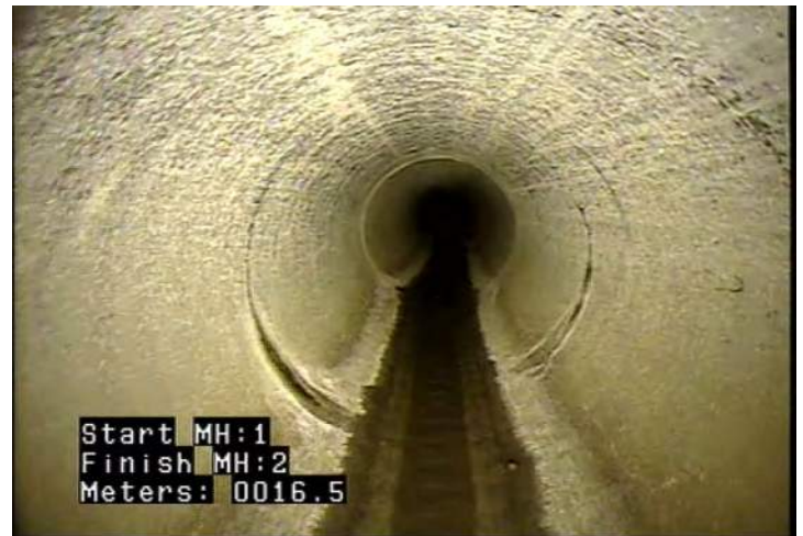
CS - Crack Spiral @ 16.5 m.
