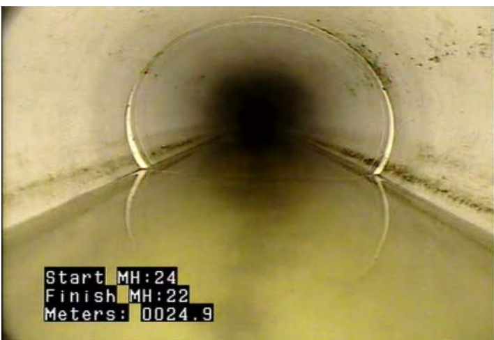
D - Pipe Deformed @ 24.9 m.
