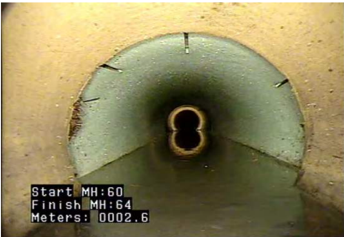
MSC - Dimension/Shape Change @ 2.6 m. RFJ - Roots, Fine: Joint @ 2.6 m.
