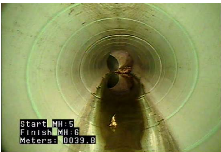
MWLS - Water Level: Sag @ 39.8 m.
