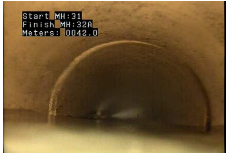
DAE - Deposits Attached: Encrustation @ 42.0 m.
