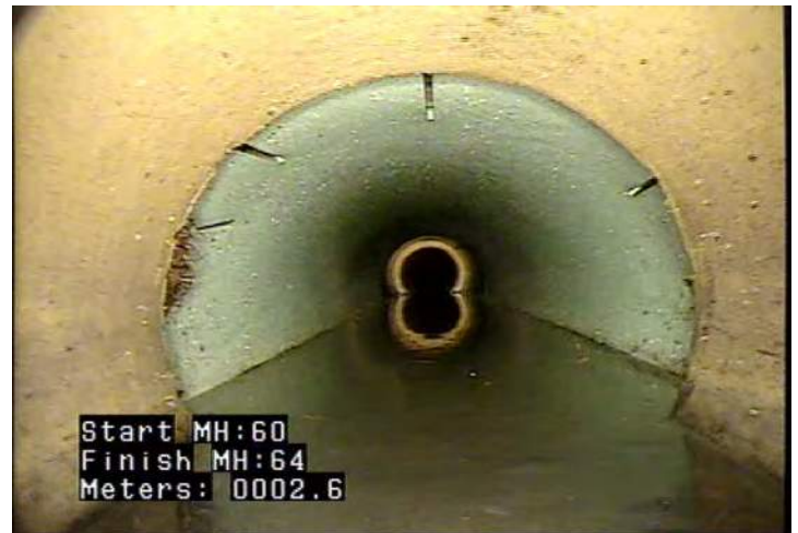
MSC - Dimension/Shape Change @ 2.6 m. RFJ - Roots, Fine: Joint @ 2.6 m.
