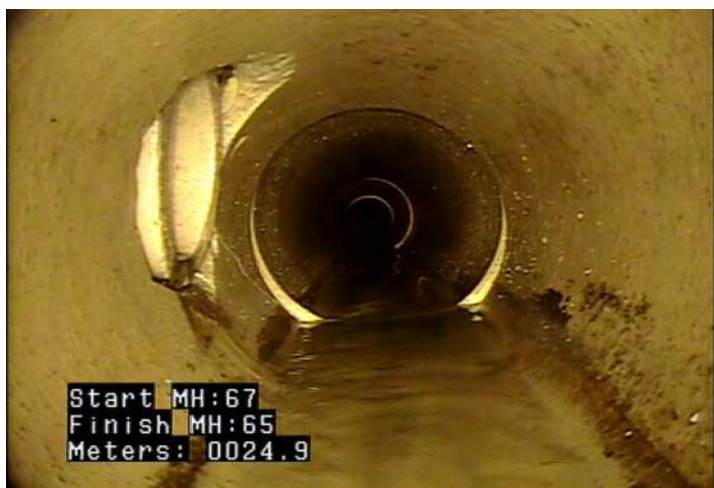
TB - Tap, Break-in / Hammer @ 24.9 m.
