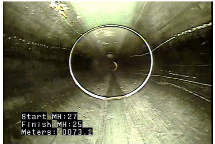
DAGS - Deposits Attached: Grease @ 73.2 m.
