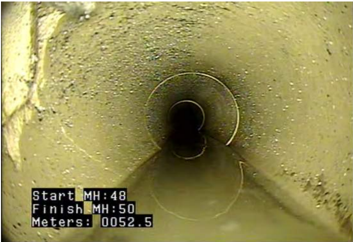
CS - Crack Spiral @ 52.5 m.
