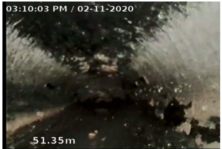
DAGS - Deposits Attached: Grease @ 51.4 m.
