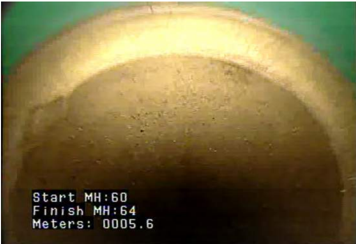
RPR - Point Repair - Pipe Replaced @ 5.6 m. PVC Ends
