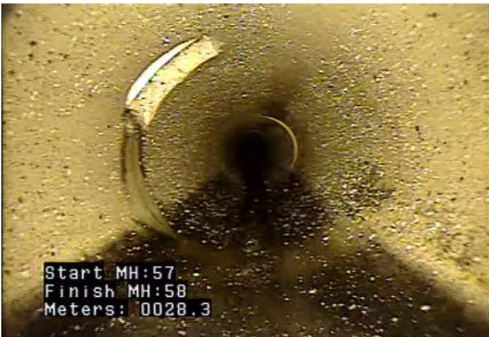
TB - Tap, Break-in / Hammer @ 28.3 m.
