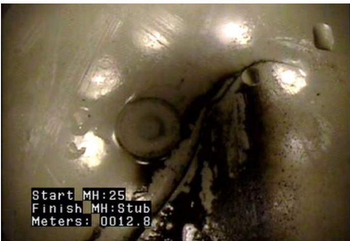
AEP - Access Point - End of Pipe @ 12.8 m. Stub - Crack in cap.
