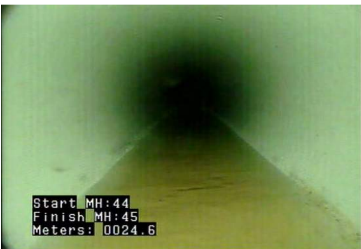
MWLS - Water Level: Sag @ 24.6 m.
