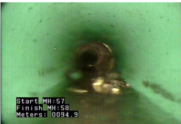
DSGV - Deposits Settled: Gravel @ 94.9 m.
