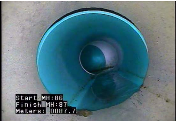
JOM - Joint Offset (displaced): Medium @ 87.7 m.
