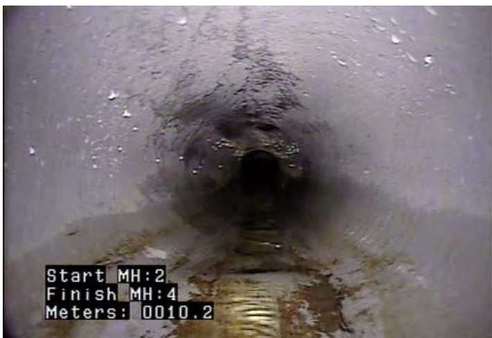
D - Pipe Deformed @ 10.2 m.
