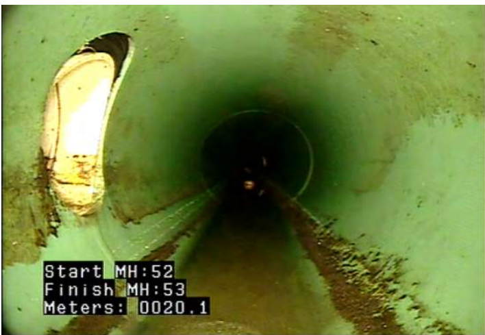
TSD - Tap, Saddle: Defective @ 20.1 m. Hole for service overcut.
