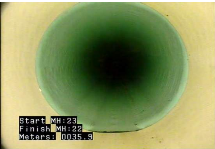
MMC - Material Change @ 35.9 m. White to Blue PVC
