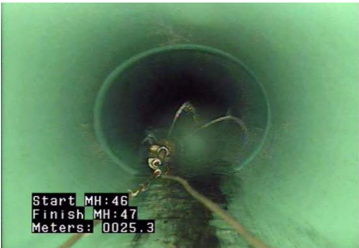
D - Pipe Deformed @ 25.3 m. Oval
