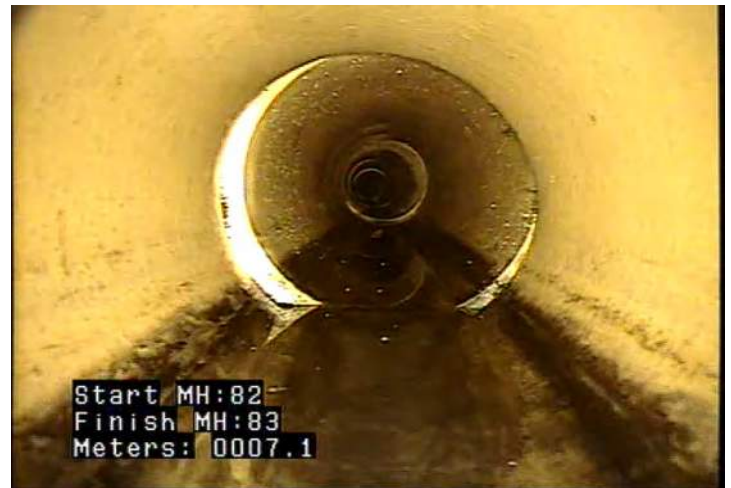
JOM - Joint Offset (displaced): Medium @ 7.1 m.
