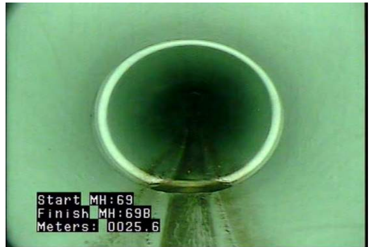
D - Pipe Deformed @ 25.6 m. Oval
