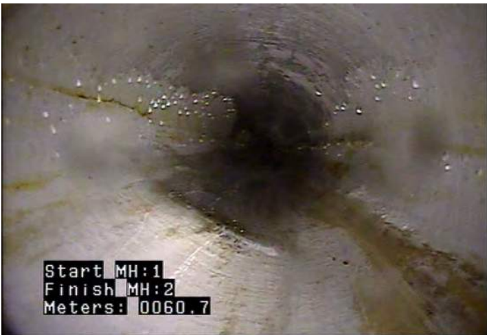
D - Pipe Deformed @ 60.7 m.
