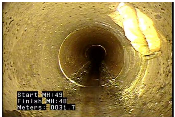
TBI - Tap, Break-in / Hammer: Intruding @ 31.7 m.
