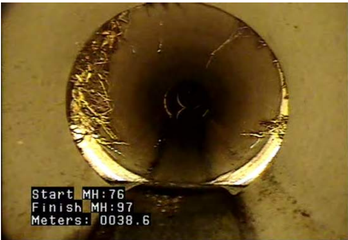
JOM - Joint Offset (displaced): Medium @ 38.6 m.
