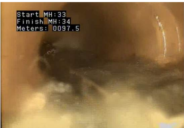
JAM - Joint Angular: Medium @ 97.5 m.
