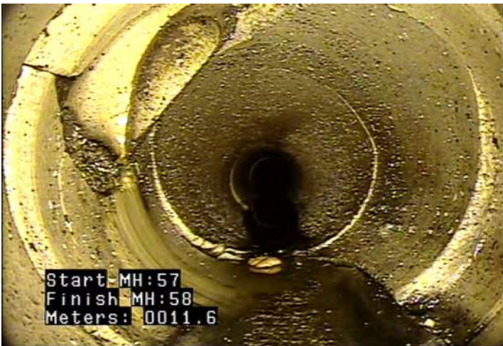
TB - Tap, Break-in / Hammer @ 11.6 m.
