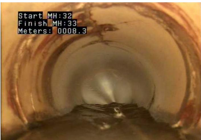
DAE - Deposits Attached: Encrustation @ 8.3 m.
