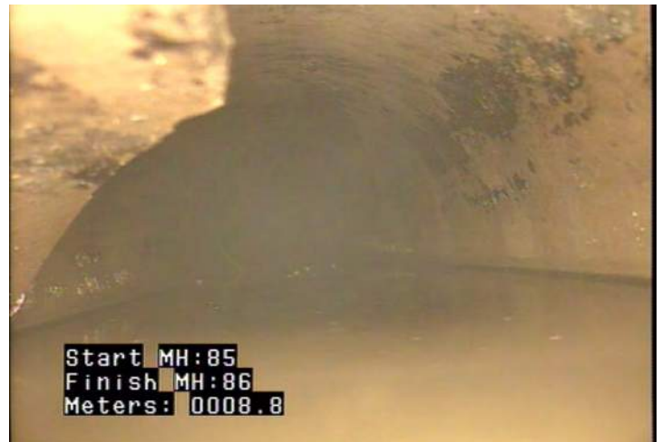
MSA - Survey Abandoned @ 8.8 m. Unable to pass broken pipe.
