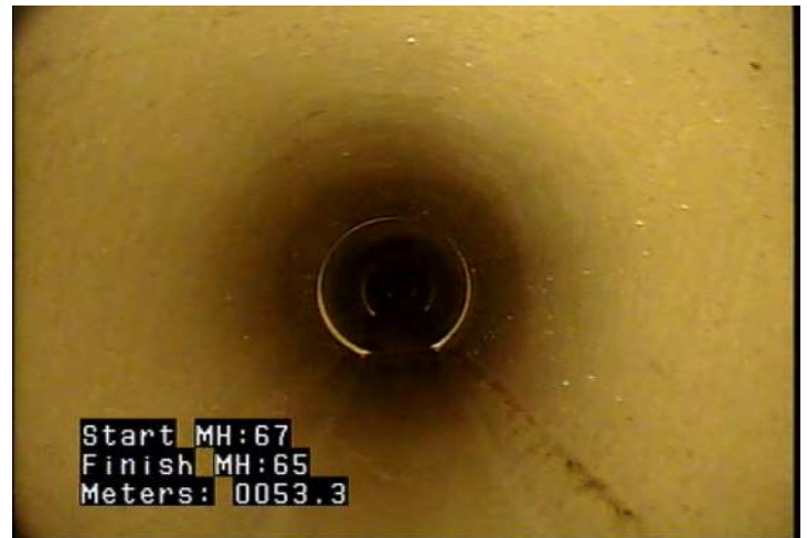
MWLS - Water Level: Sag @ 53.3 m.
