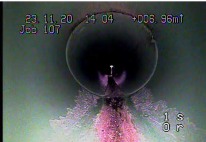
OBJ - Obstacle - Object Wedged in Joint @ 4.2 m. Branch
