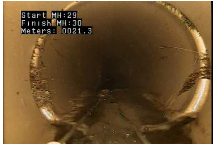
MWLS - Water Level: Sag @ 21.3 m.
