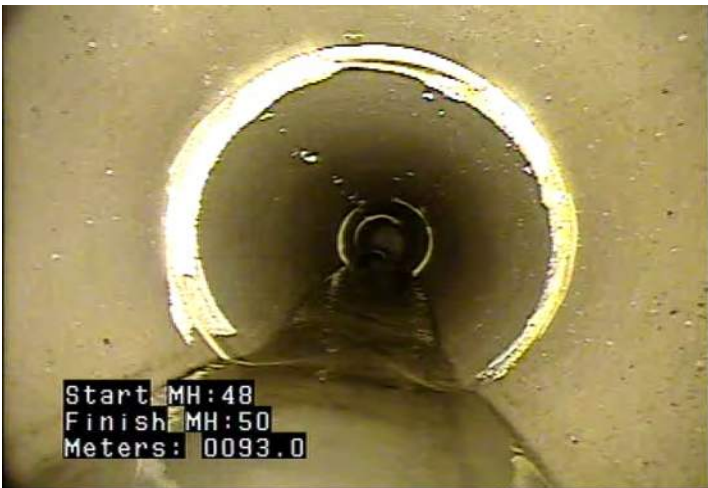
FS - Fracture Spiral @ 93.0 m.
