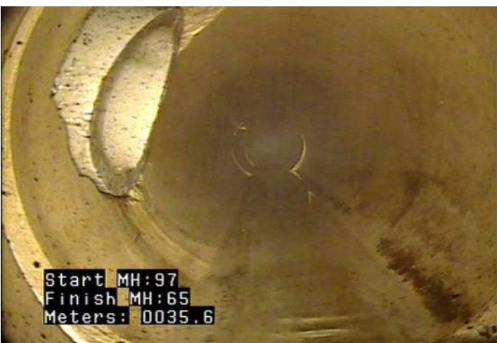
TB - Tap, Break-in / Hammer @ 35.6 m.
