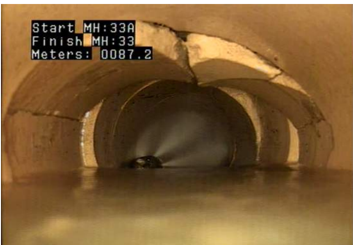
B - Pipe Broken @ 87.2 m.
