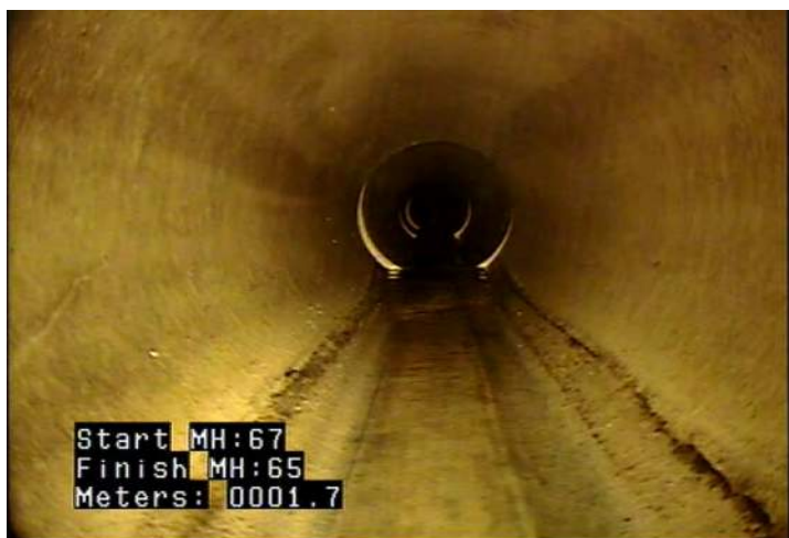
CS - Crack Spiral @ 0.5 m.
