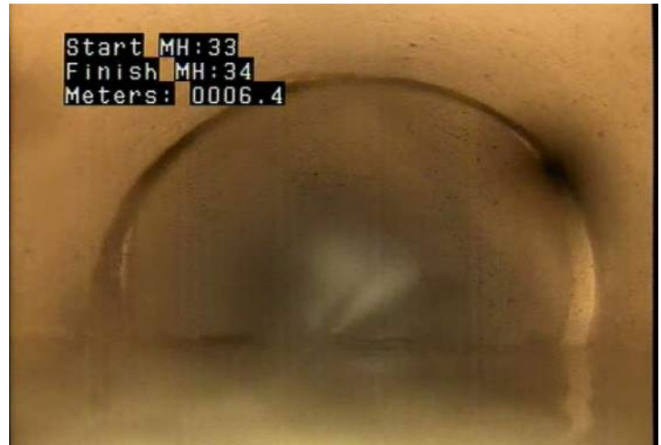
DAE - Deposits Attached: Encrustation @ 6.4 m.
