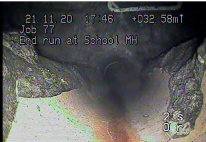
AMH - Access Point - Manhole @ 32.6 m. School MH - Troughing in MH Broken
