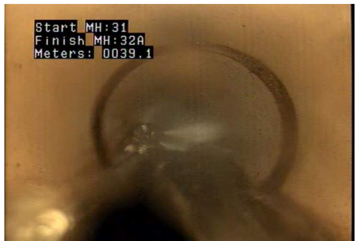
DAE - Deposits Attached: Encrustation @ 39.1 m.
