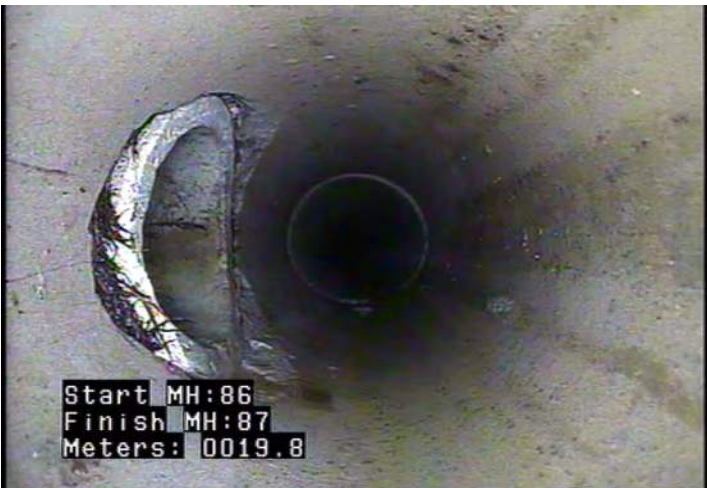
TB - Tap, Break-in / Hammer @ 19.8 m.
