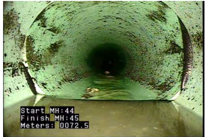
ISSR - Intruding Seal Material - Sealing Ring @ 72.5 m. Possibly sealing ring holding back debris/water at bottom of pipe
