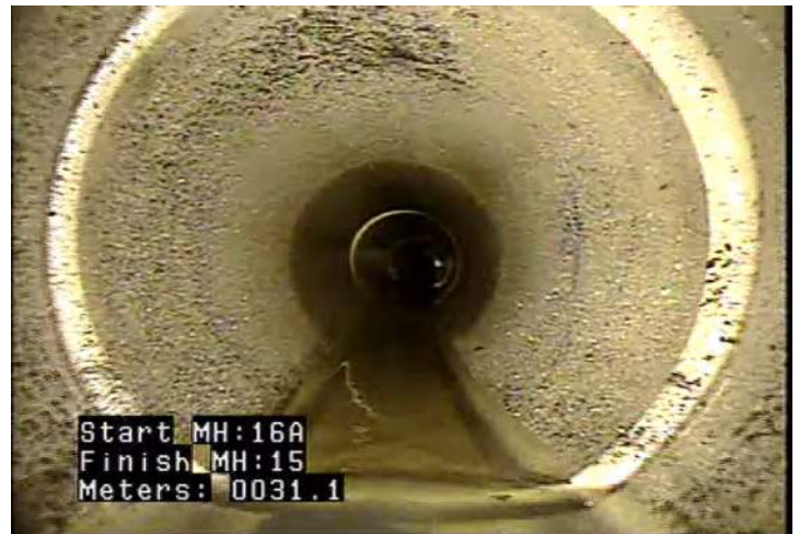
MWLS - Water Level: Sag @ 31.1 m.
