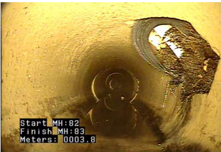
RMC - Roots, Medium: Connection @ 3.8 m.
