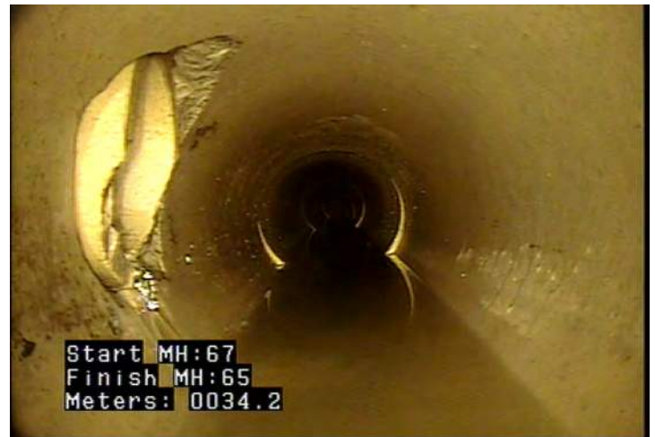
TBA - Tap, Break-in / Hammer: Active @ 34.2 m.
