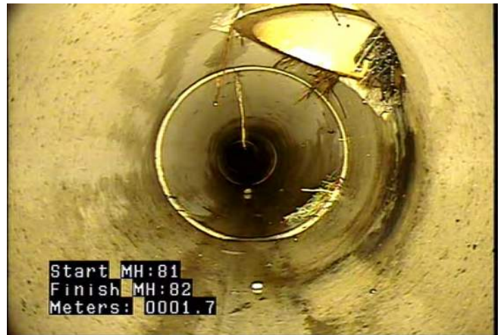
RFC - Roots, Fine: Connection @ 1.7 m.
