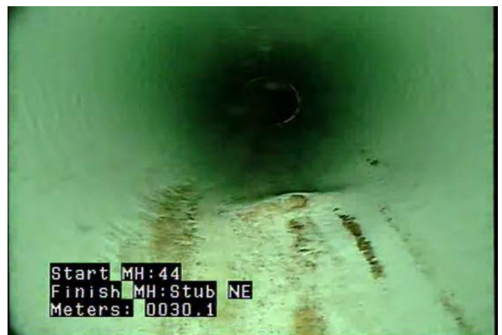
D - Pipe Deformed @ 30.1 m.
