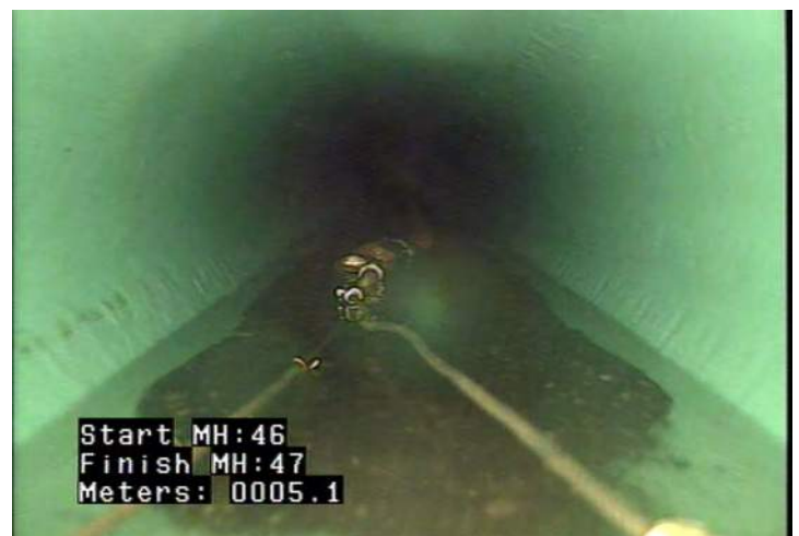
DSGV - Deposits Settled: Gravel @ 5.1 m.
