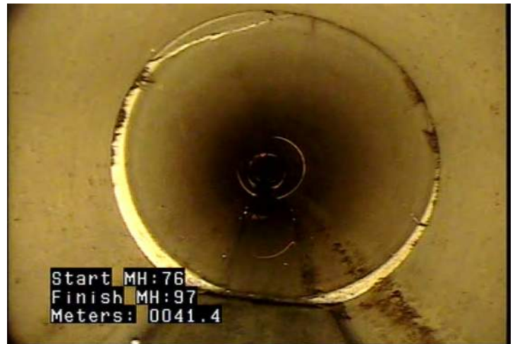
FS - Fracture Spiral @ 41.4 m.
