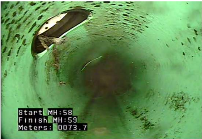
RFC - Roots, Fine: Connection @ 73.7 m.
