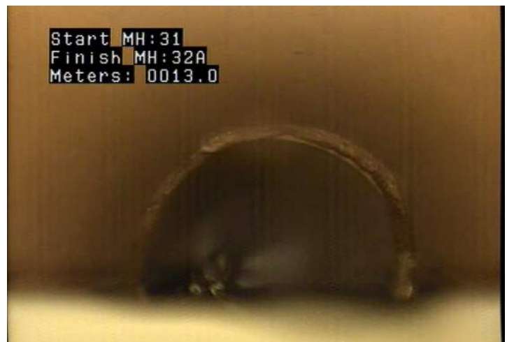
DAE - Deposits Attached: Encrustation @ 13.0 m.
