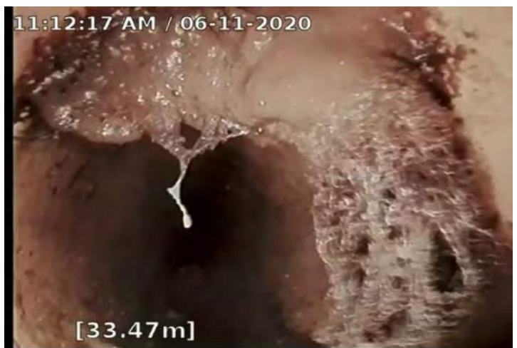
RMJ - Roots, Medium, Joint @ 33.4 m.
