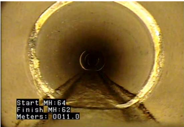
DAE - Deposits Attached: Encrustation @ 11.0 m.
