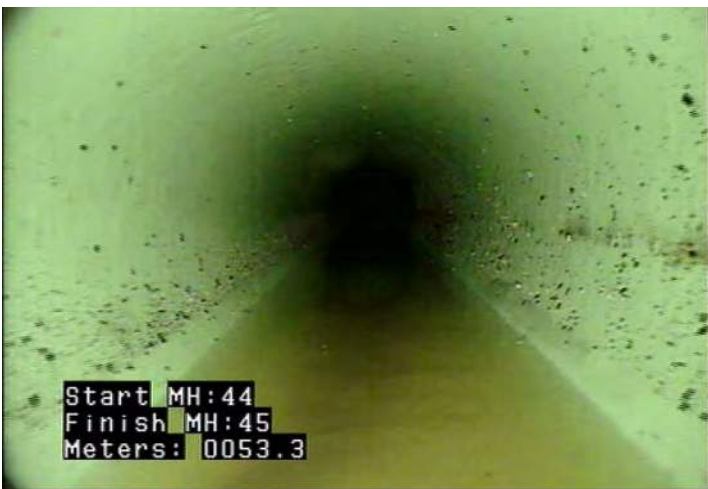
MWLS - Water Level: Sag @ 53.3 m.
