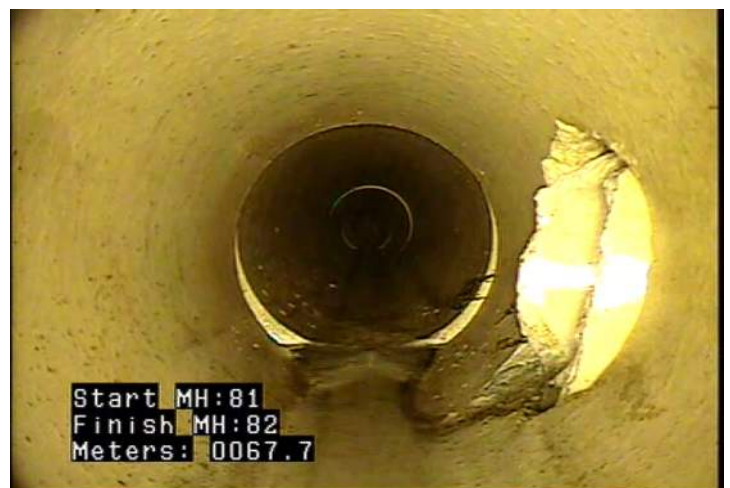
TBI - Tap, Break-in / Hammer: Intruding @ 67.7 m.
