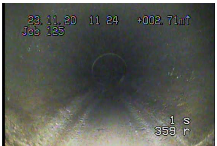
ISGT - Intruding Seal Material - Grout @ 1.6 m.
