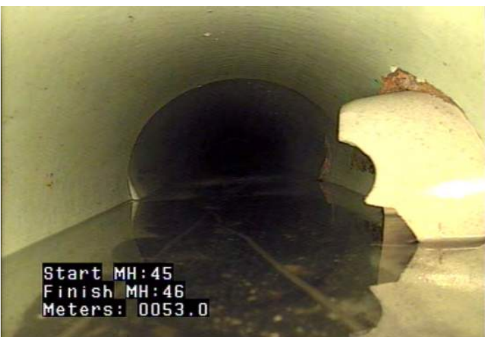
TSI - Tap, Saddle: Intruding @ 53.0 m. Connecting pipe broken
