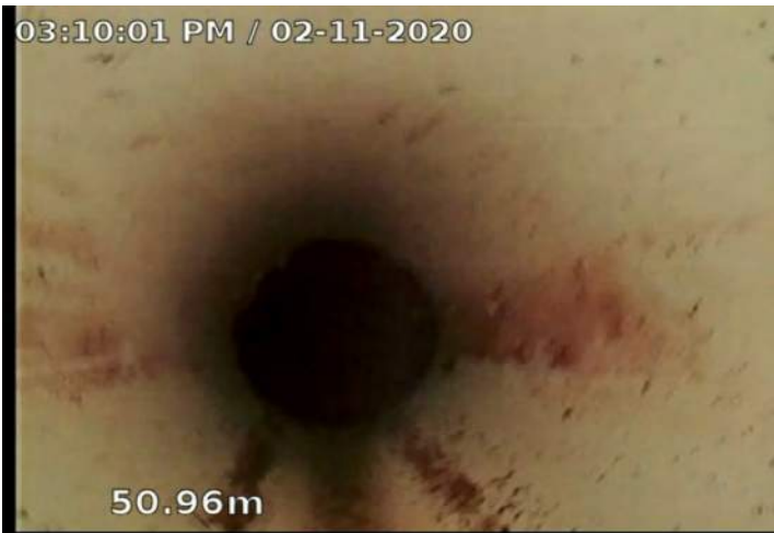
MMC - Material Change @ 51.0 m. PVC to ABS
