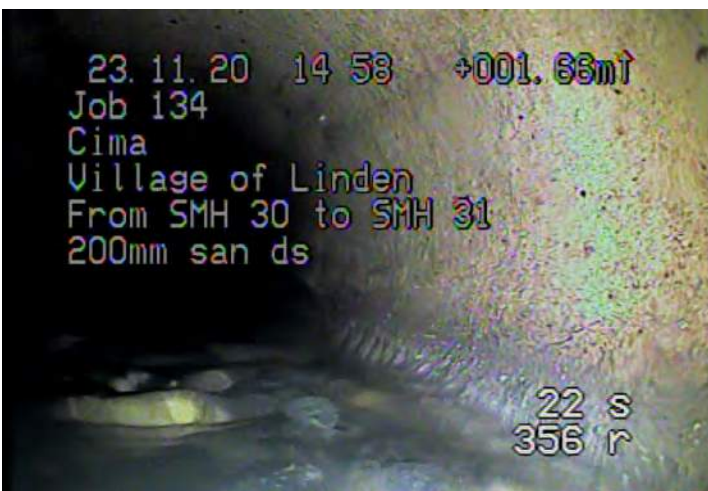
DSGV - Deposits Settled: Gravel @ 0.5 m.
