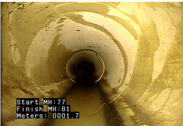
CM - Crack Multiple @ 0.5 m.
