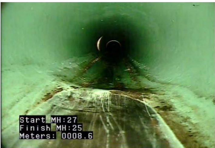
D - Pipe Deformed @ 8.6 m.
