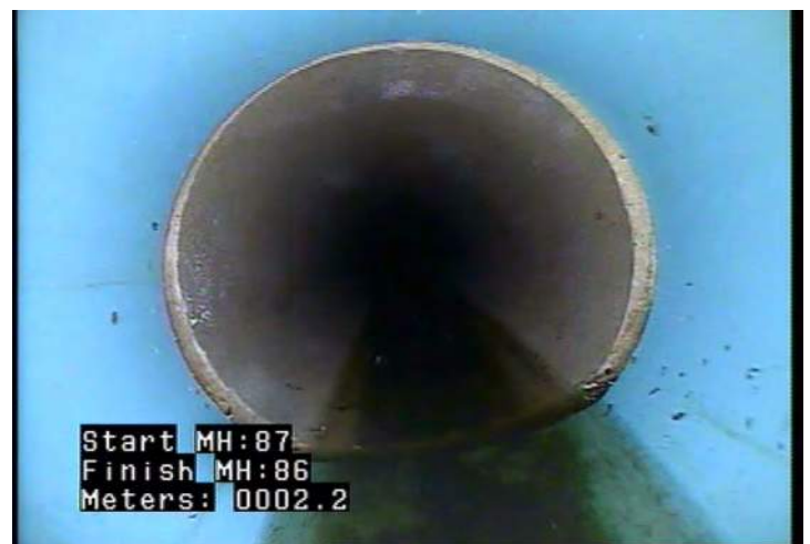
MMC - Material Change @ 2.3 m. PVC to Clay tile
