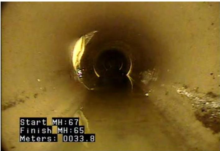
MWLS - Water Level: Sag @ 33.8 m.
