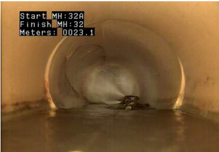
CM - Crack Multiple @ 23.1 m.
