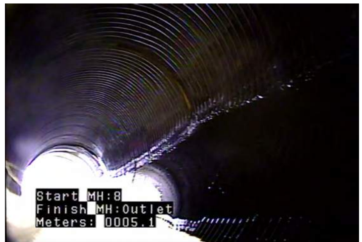
MSA - Survey Abandoned @ 5.1 m. Ts into a bigger storm line.
