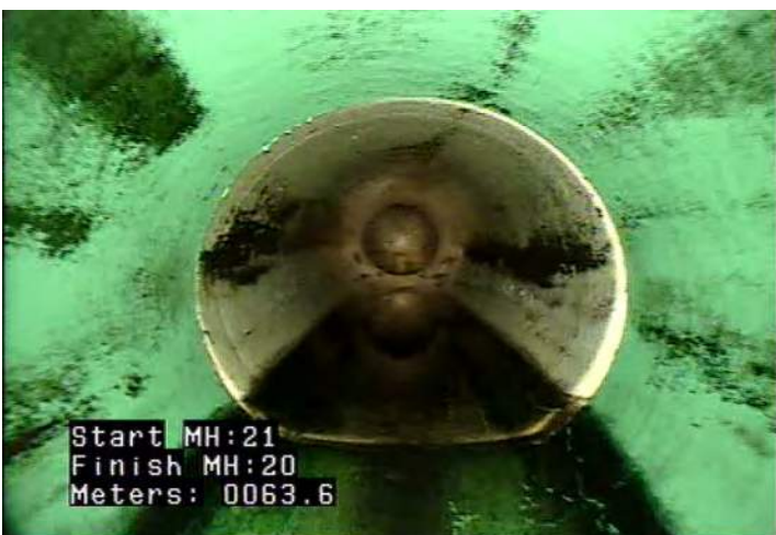
MMC - Material Change @ 63.6 m. Blue to White PVC
