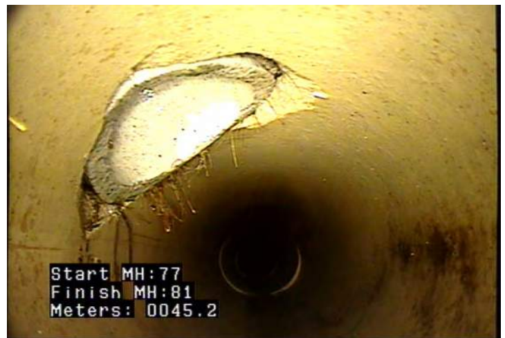
RFC - Roots, Fine: Connection @ 45.1 m.
