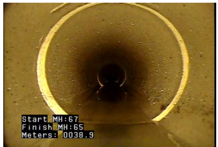
MWLS - Water Level: Sag @ 38.9 m.
