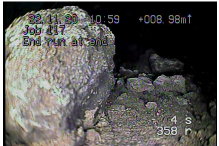
MSA - Survey Abandoned @ 9.0 m. Pipe ends in gravel
