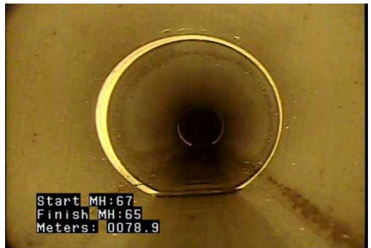
MWLS - Water Level: Sag @ 78.9 m.
