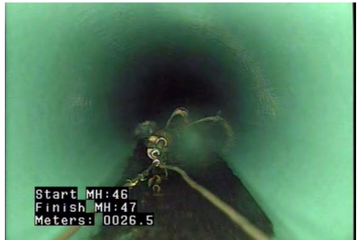
DSGV - Deposits Settled: Gravel @ 26.5 m.
