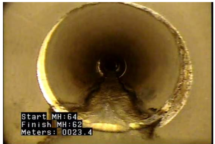
DAE - Deposits Attached: Encrustation @ 24.8 m.
