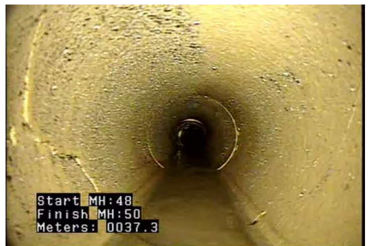
B - Pipe Broken @ 37.4 m.
