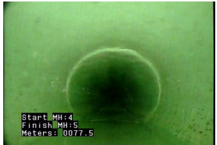
MWLS - Water Level: Sag @ 77.5 m.
