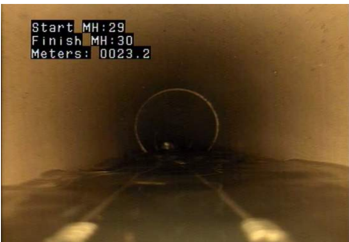
DSGV - Deposits Settled: Gravel @ 23.2 m.
