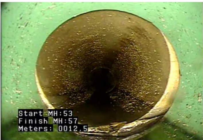
JOM - Joint Offset (displaced): Medium @ 12.5 m.
