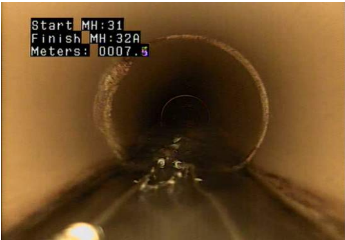
DAE - Deposits Attached: Encrustation @ 7.4 m.
