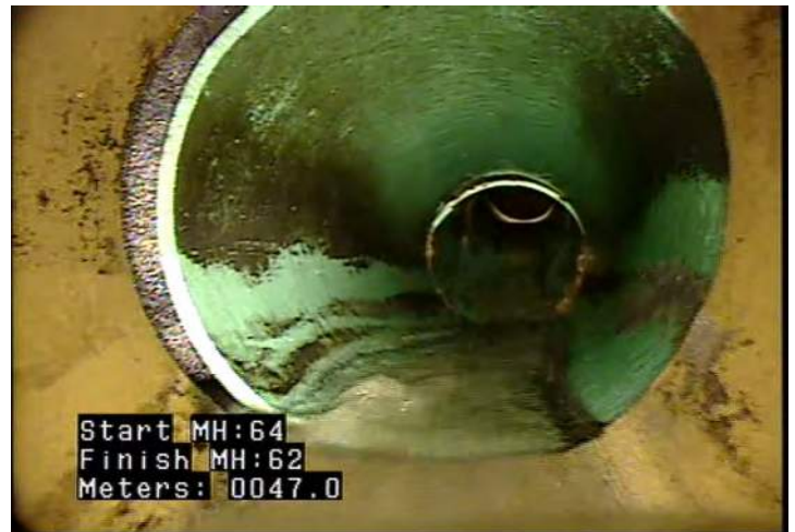
MMC - Material Change @ 47.0 m. Clay tile to PVC
