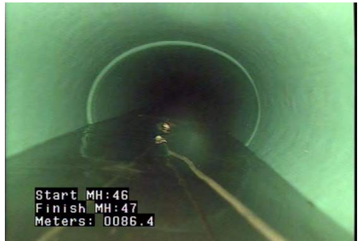
D - Pipe Deformed @ 86.4 m. Oval
