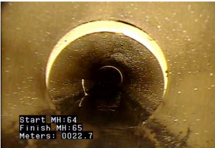
JOL - Joint Offset (displaced): Large @ 22.7 m.
