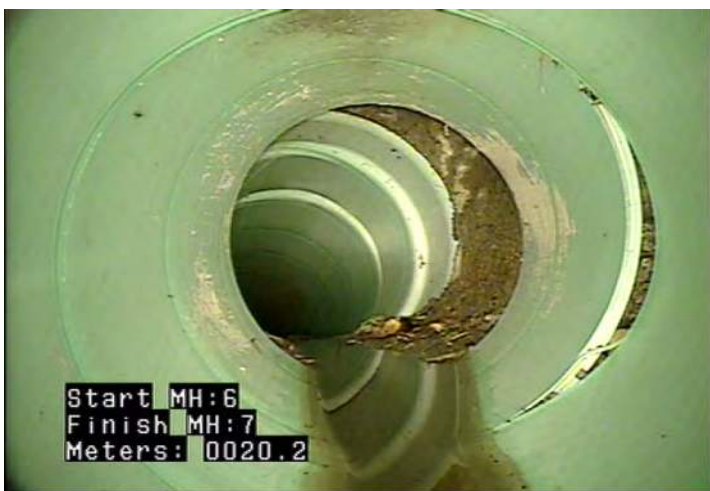
JOM - Joint Offset (displaced): Medium @ 20.2 m.
