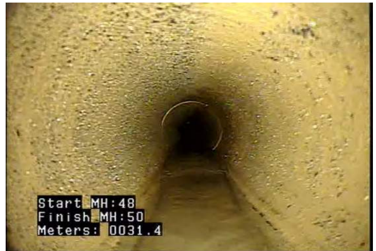
FM - Fracture Multiple @ 31.4 m.
