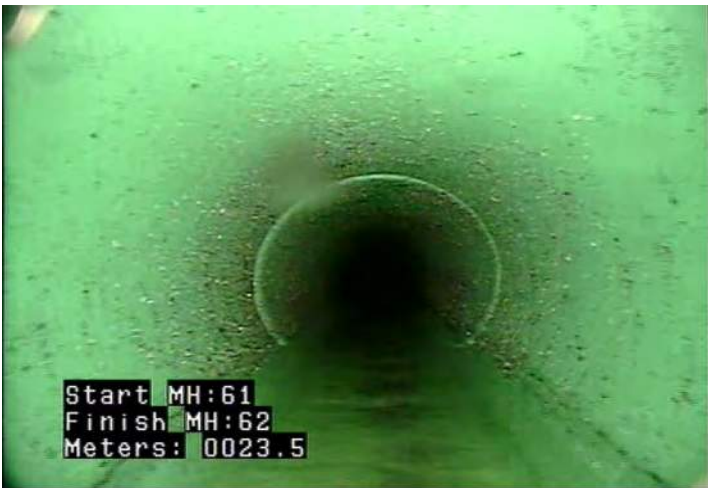
MWLS - Water Level: Sag @ 23.5 m.
