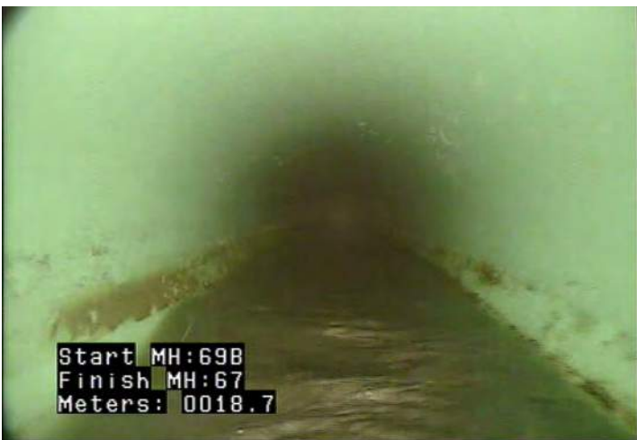
MWLS - Water Level: Sag @ 18.7 m.
