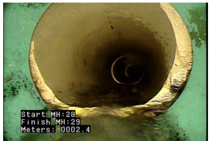
MMC - Material Change @ 2.4 m. PVC to Clay tile
