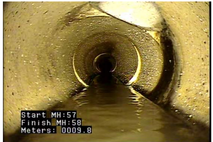
TB - Tap, Break-in / Hammer @ 9.8 m.
