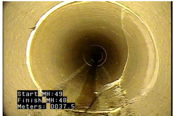
FM - Fracture Multiple @ 37.5 m.
