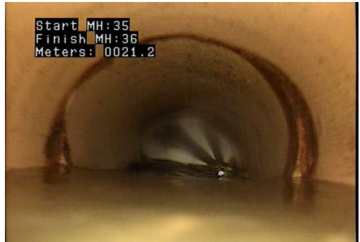
DAE - Deposits Attached: Encrustation @ 21.2 m.
