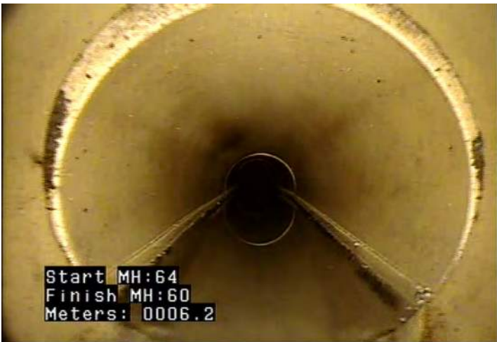
MWLS - Water Level: Sag @ 6.2 m.
