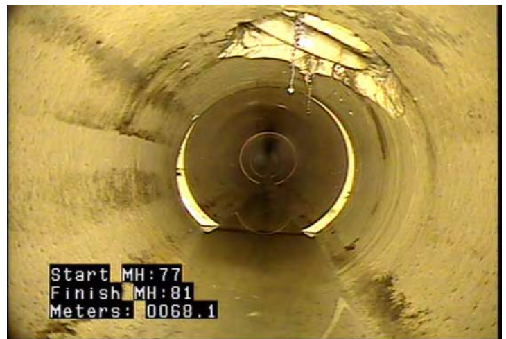
TB - Tap, Break-in / Hammer @ 68.1 m.
