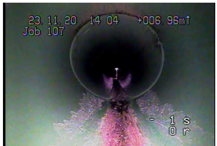
DSGV - Deposits Settled: Gravel @ 4.2 m.
