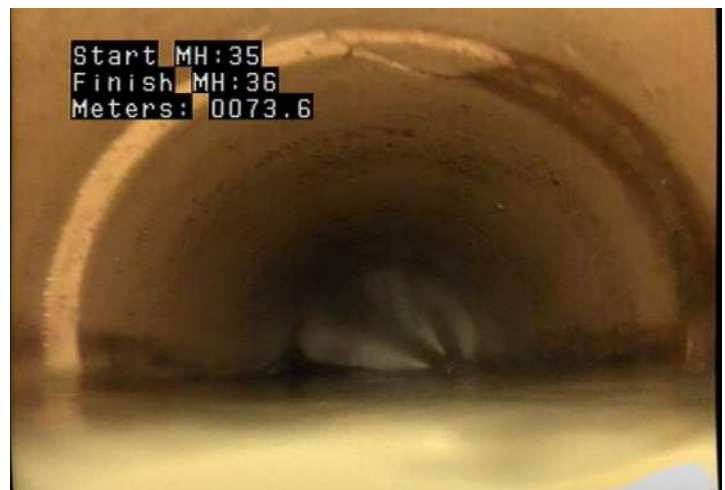
FC - Fracture Circumferential @ 73.6 m.
