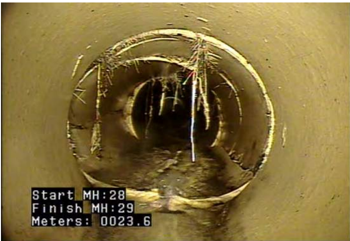
RFB - Roots, Fine: Barrel @ 23.6 m.
