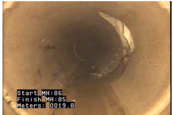
TB - Tap, Break-in / Hammer @ 19.8 m.
