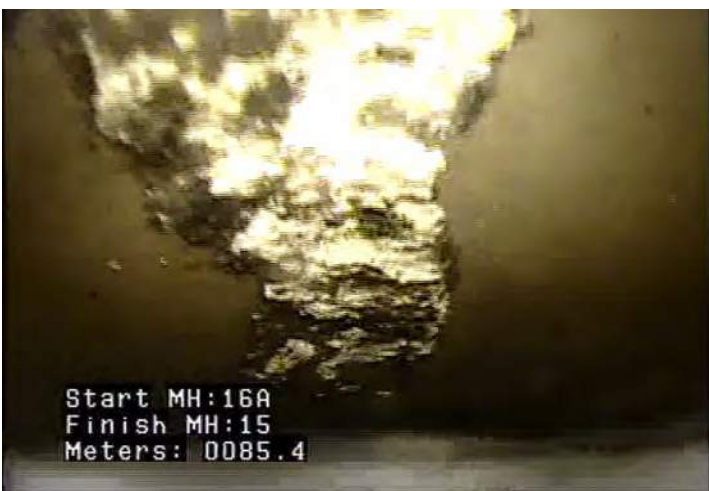
DAGS - Deposits Attached: Grease @ 85.6 m.
