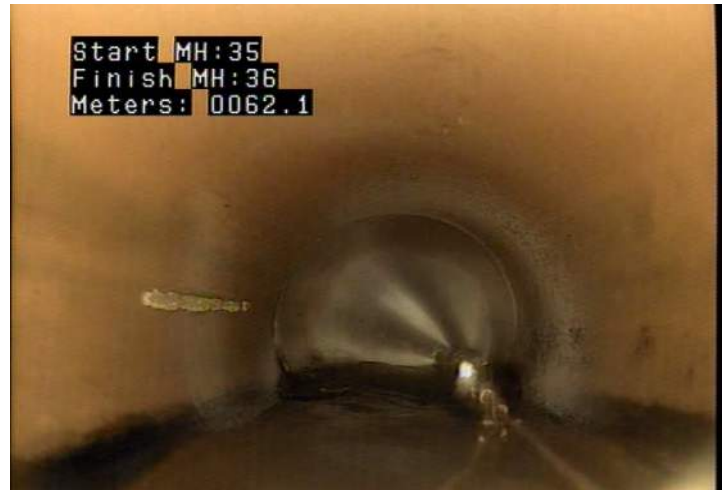
DAGS - Deposits Attached: Grease @ 62.1 m.
