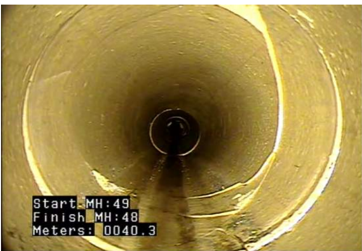
FM - Fracture Multiple @ 40.3 m.
