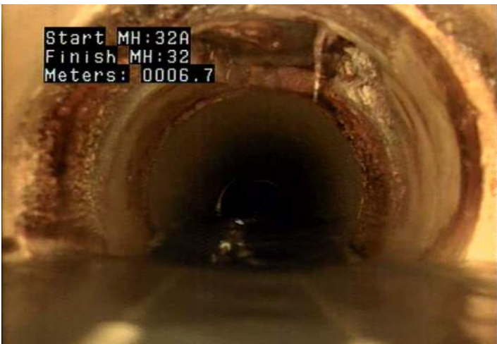
DAE - Deposits Attached: Encrustation @ 6.7 m.
