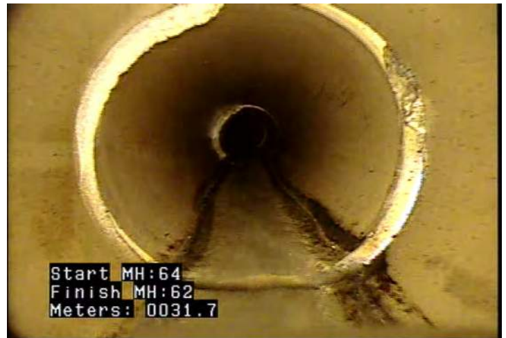
DAE - Deposits Attached: Encrustation @ 31.7 m.
