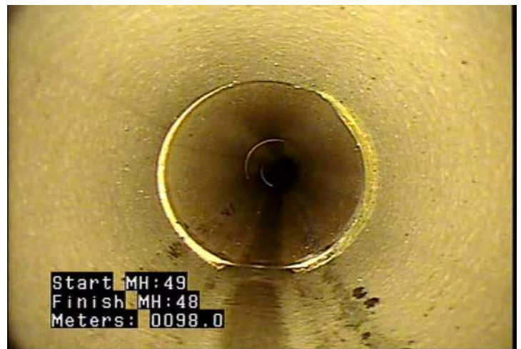
DAE - Deposits Attached: Encrustation @ 98.0 m.
