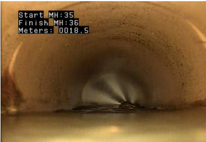
DAE - Deposits Attached: Encrustation @ 18.5 m.
