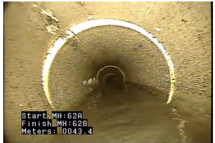
DAGS - Deposits Attached: Grease @ 43.4 m.
