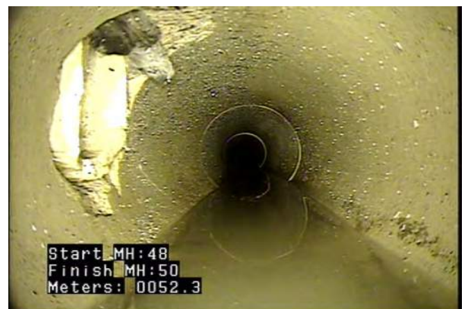
TBD - Tap, Break-in / Hammer: Defective @ 52.3 m. Plastic intruding from top of service.
