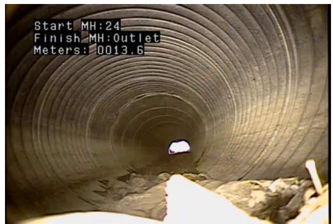
MSA - Survey Abandoned @ 13.6 m. Unable to pass rocks. Rest of line examined with zoom. 10% gravel viewed.
