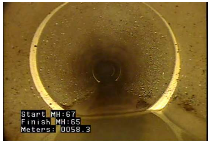
MWLS - Water Level: Sag @ 58.3 m.
