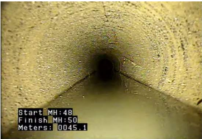
CM - Crack Multiple @ 45.1 m.
