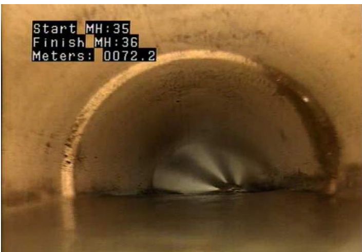
DAE - Deposits Attached: Encrustation @ 72.2 m.
