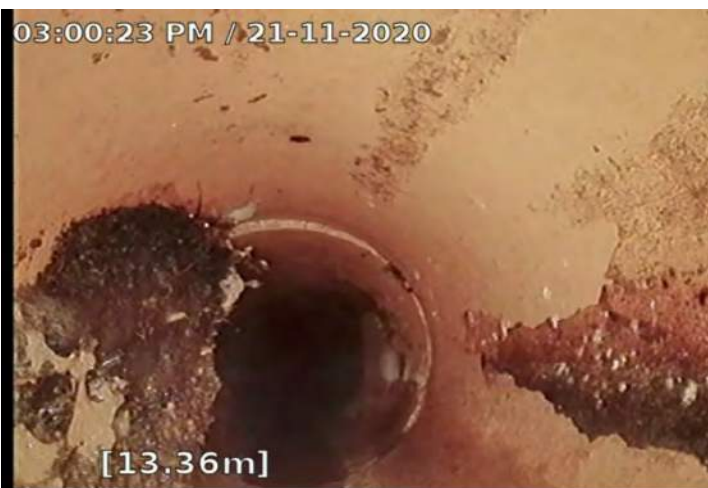
RMJ - Roots, Medium, Joint @ 13.3 m.
