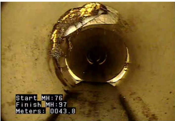
RMC - Roots, Medium: Connection @ 43.8 m.
