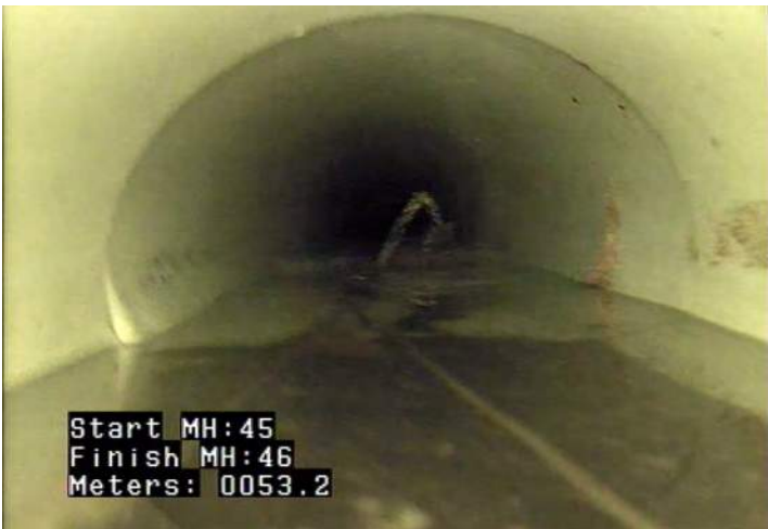
B - Pipe Broken @ 53.2 m. See Job 34R
