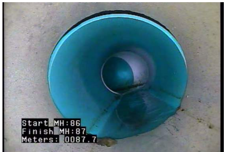
MMC - Material Change @ 87.7 m. Clay tile to PVC
