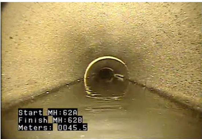
MWLS - Water Level: Sag @ 45.5 m.
