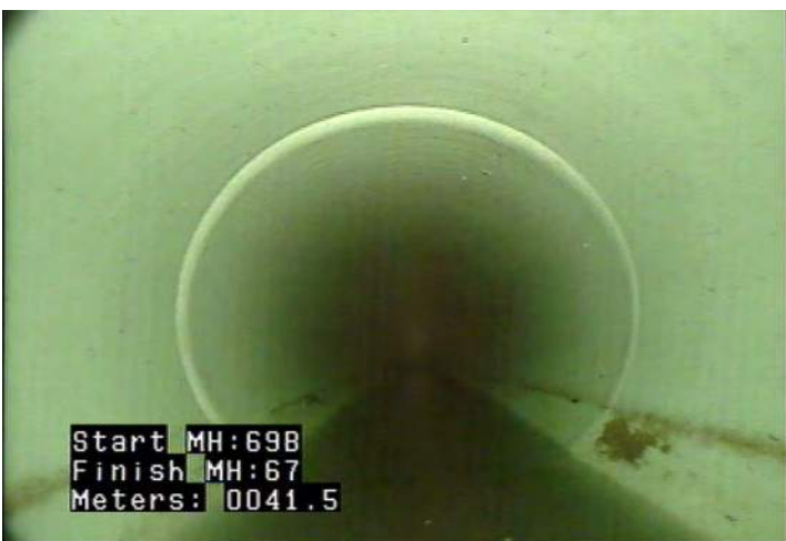
MWLS - Water Level: Sag @ 41.5 m.
