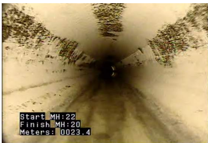
MWLS - Water Level: Sag @ 23.4 m.
