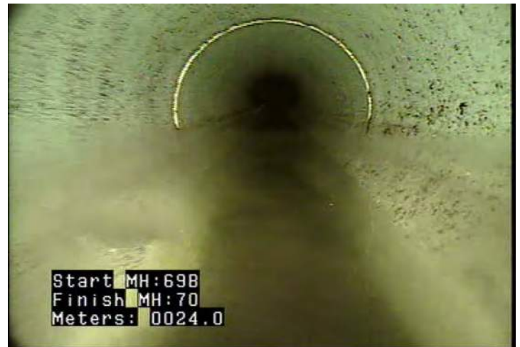
MWLS - Water Level: Sag @ 24.0 m.
