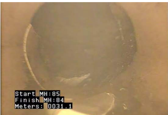
FC - Fracture Circumferential @ 31.1 m.
