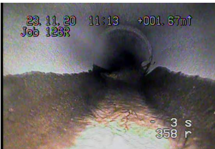
ISGT - Intruding Seal Material - Grout @ 1.3 m.
