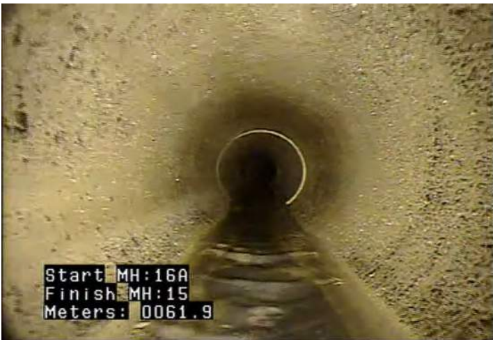
MWLS - Water Level: Sag @ 61.9 m.
