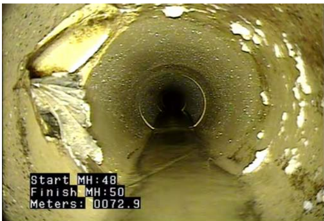
TBD - Tap, Break-in / Hammer: Defective @ 72.9 m. Plastic intruding from bottom of service.
