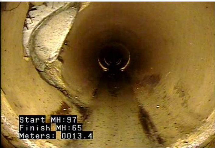
TB - Tap, Break-in / Hammer @ 13.4 m.
