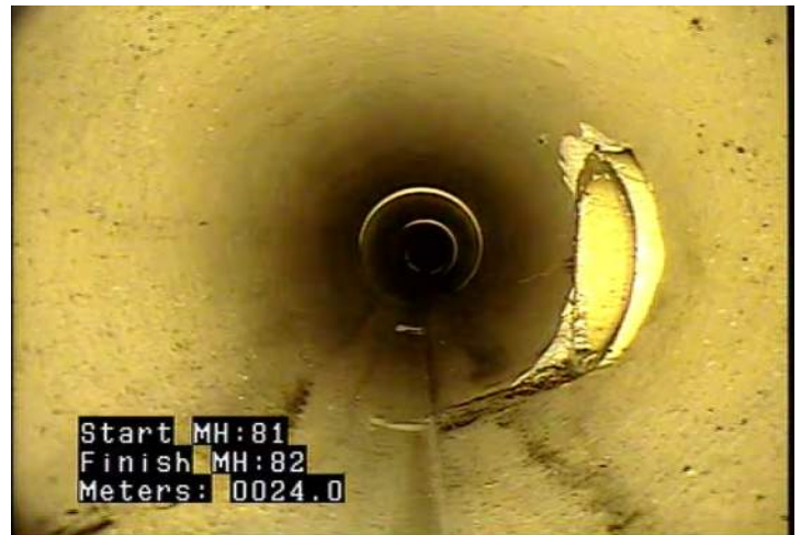
TB - Tap, Break-in / Hammer @ 24.0 m.
