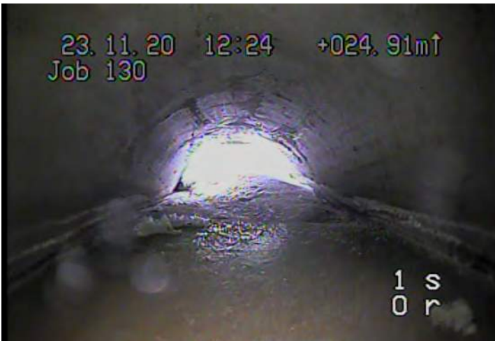
MMC - Material Change @ 24.5 m. PVC to Concrete
