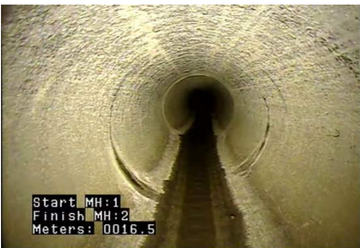
IS - Infiltration - Stain @ 16.7 m.
