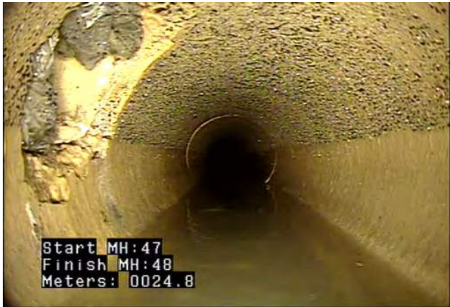
TBD - Tap, Break-in / Hammer: Defective @ 24.8 m. Plastic intruding from top of service.
