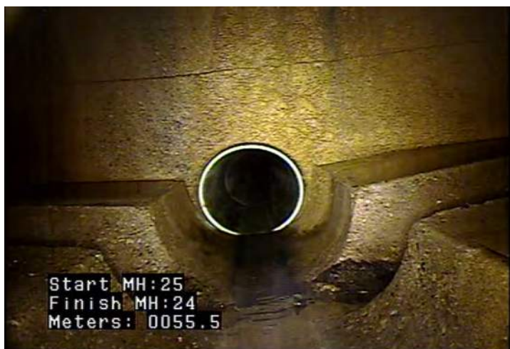
AMH - Access Point - Manhole @ 55.5 m. S MH 24
