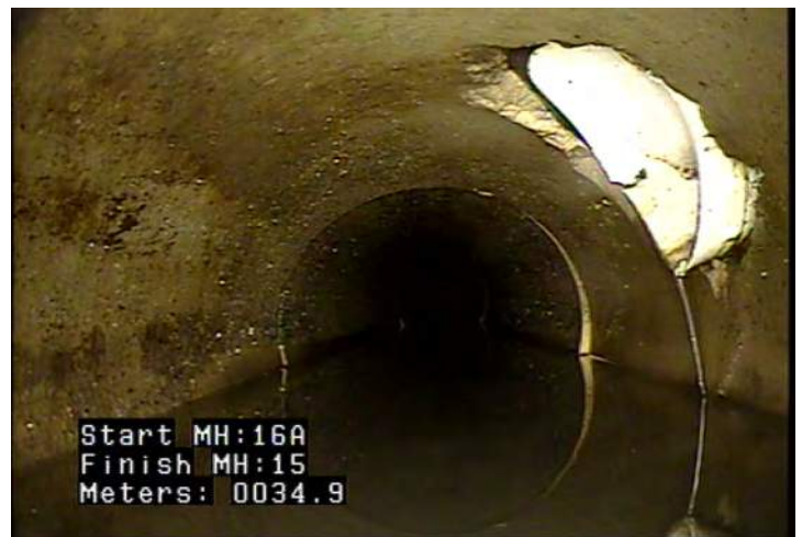
TB - Tap, Break-in / Hammer @ 34.9 m.
