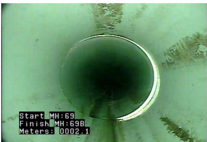
JOM - Joint Offset (displaced): Medium @ 2.1 m.
