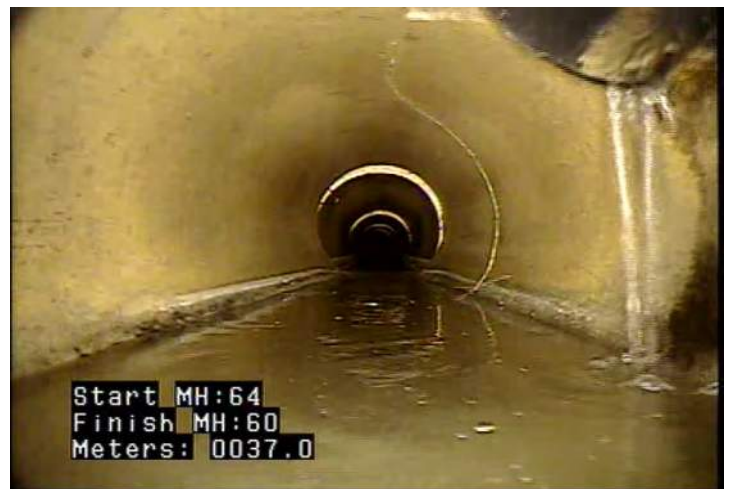
CS - Crack Spiral @ 37.1 m.
