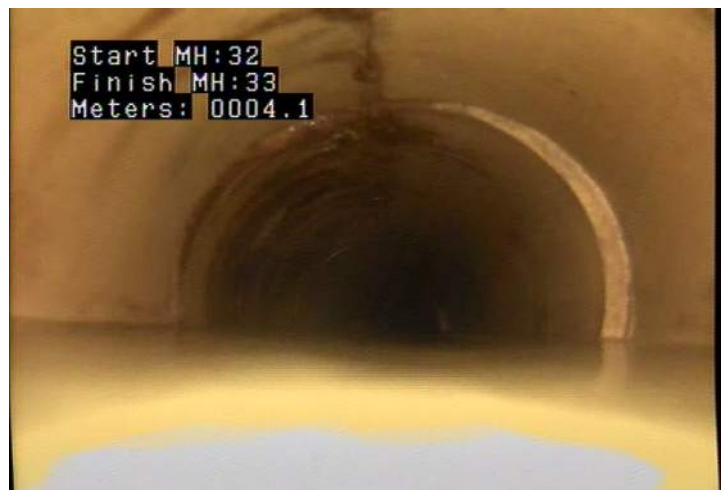
DAE - Deposits Attached: Encrustation @ 4.1 m.
