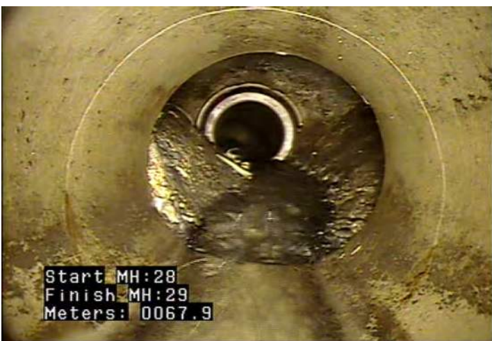
CC - Crack Circumferential @ 67.9 m.
