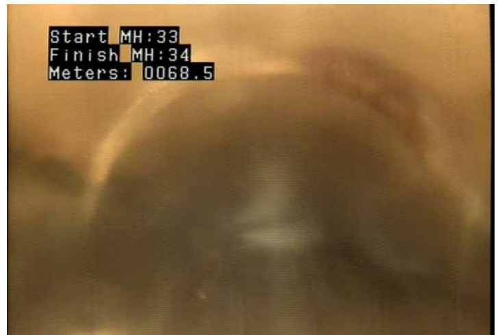
DAE - Deposits Attached: Encrustation @ 68.5 m.
