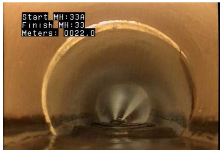
CC - Crack Circumferential @ 22.0 m.
