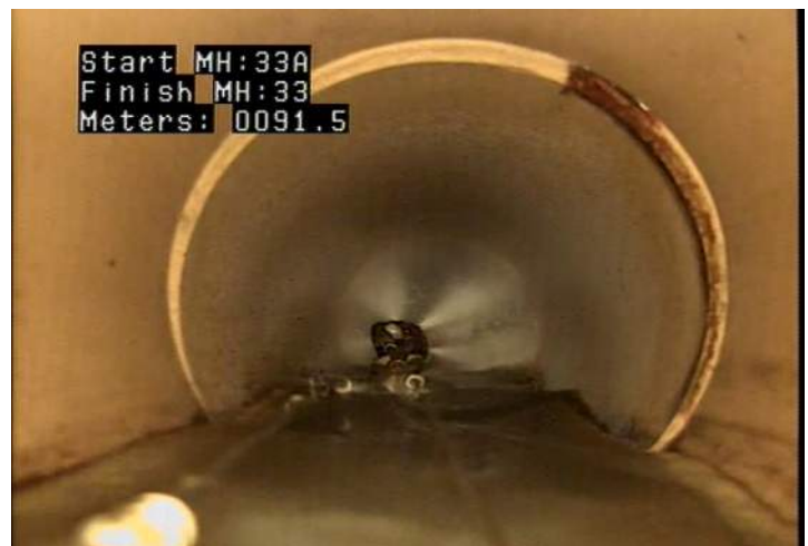
DAE - Deposits Attached: Encrustation @ 91.5 m.
