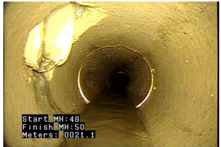
TBI - Tap, Break-in / Hammer: Intruding @ 21.1 m.
