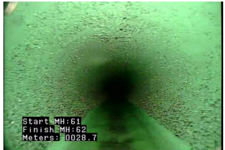
MWLS - Water Level: Sag @ 28.7 m.
