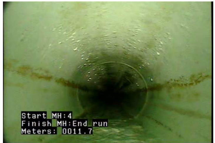
MWLS - Water Level: Sag @ 11.7 m.
