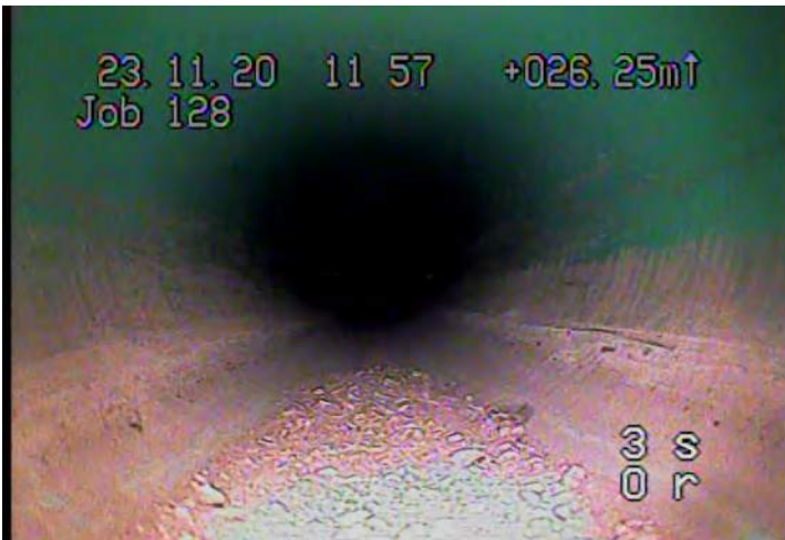
DSGV - Deposits Settled: Gravel @ 24.5 m.
