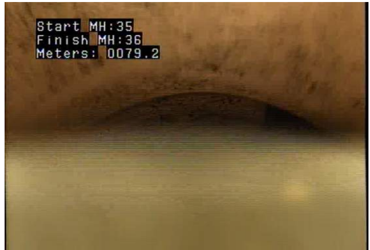
DAE - Deposits Attached: Encrustation @ 79.2 m.
