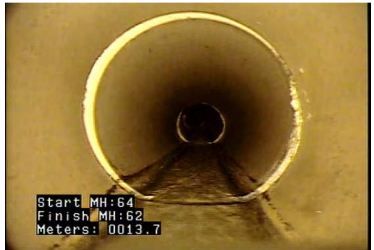
DAE - Deposits Attached: Encrustation @ 13.7 m.
