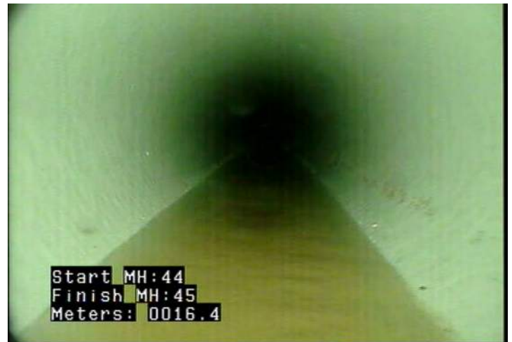
MWLS - Water Level: Sag @ 16.3 m.
