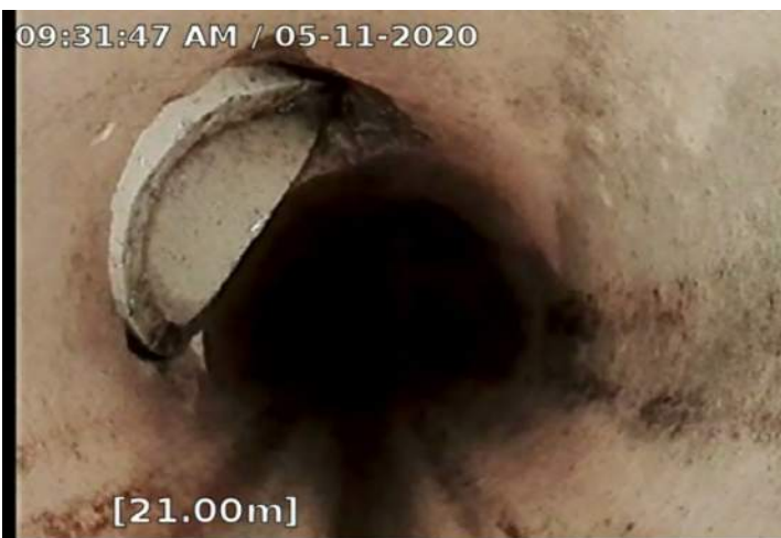
MSA - Survey Abandoned @ 21.0 m. @ Service. Rest of line seen in Job 52.
