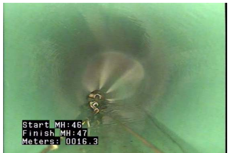
MWLS - Water Level: Sag @ 16.3 m. Flusher on
