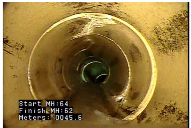
CM - Crack Multiple @ 45.6 m.
