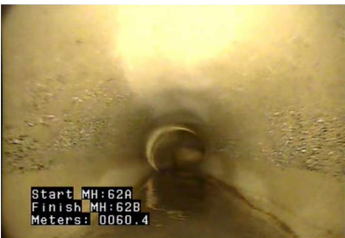
MWLS - Water Level: Sag @ 60.4 m.
