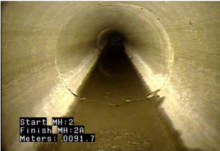
MWLS - Water Level: Sag @ 91.7 m.
