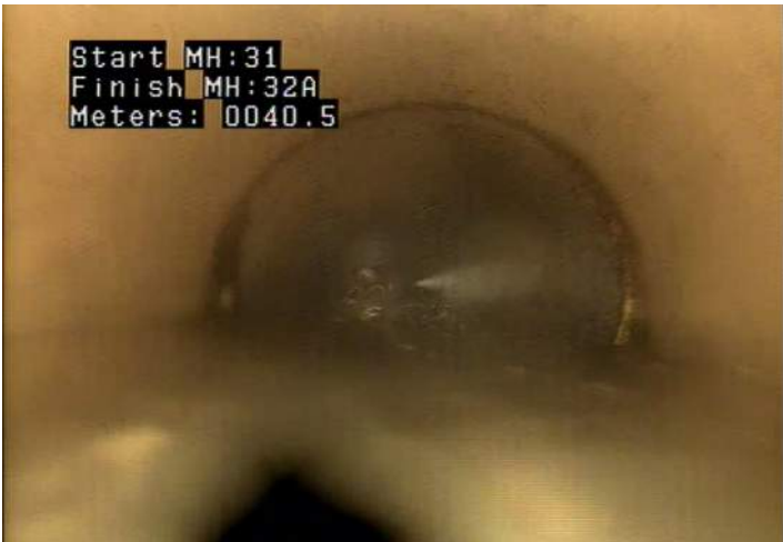
DAE - Deposits Attached: Encrustation @ 40.5 m.
