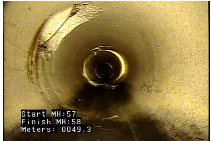
TB - Tap, Break-in / Hammer @ 49.3 m.
