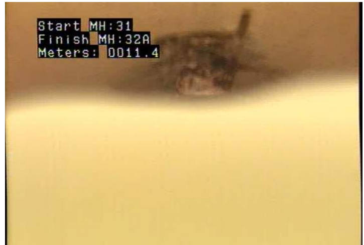
H - Hole in Pipe @ 11.4 m. Hole cut
