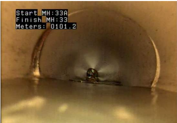
DAE - Deposits Attached: Encrustation @ 101.2 m.
