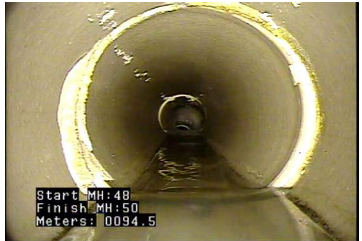
DAE - Deposits Attached: Encrustation @ 94.5 m.
