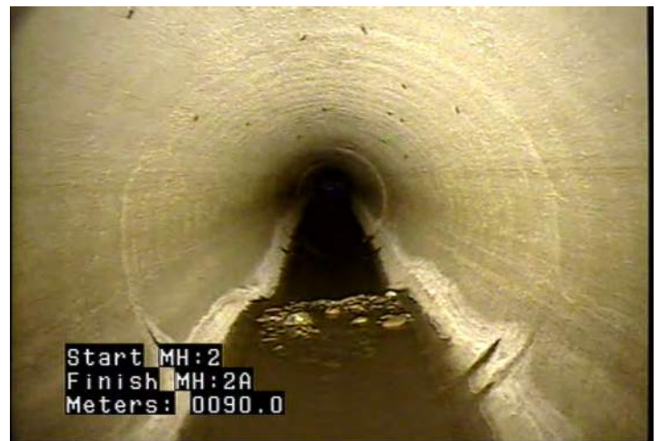
DSGV - Deposits Settled: Gravel @ 90.0 m.
