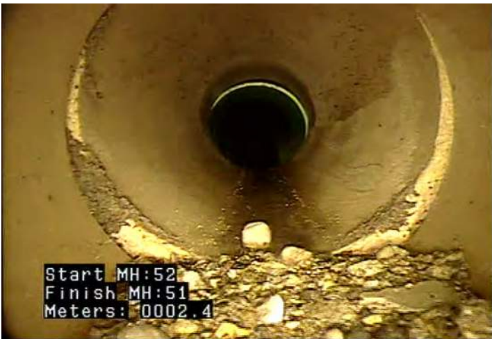
JOM - Joint Offset (displaced): Medium @ 2.4 m.
