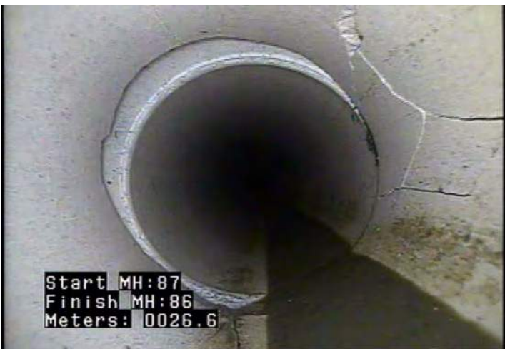
B - Pipe Broken @ 26.6 m. Broken joint, piece missing
