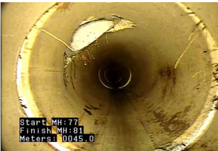
TB - Tap, Break-in / Hammer @ 45.1 m.
