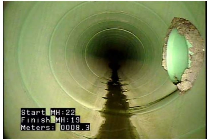
TB - Tap, Break-in / Hammer @ 8.3 m. Concrete around service
