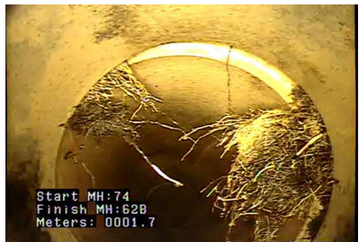
RMJ - Roots, Medium, Joint @ 1.7 m.
