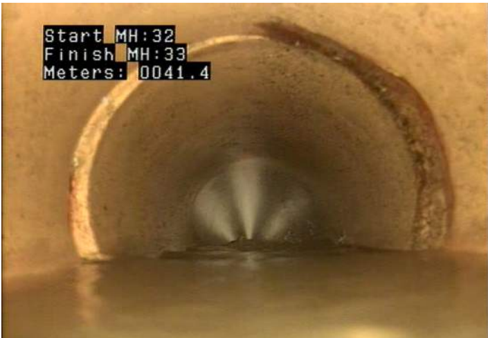
DAE - Deposits Attached: Encrustation @ 41.4 m.
