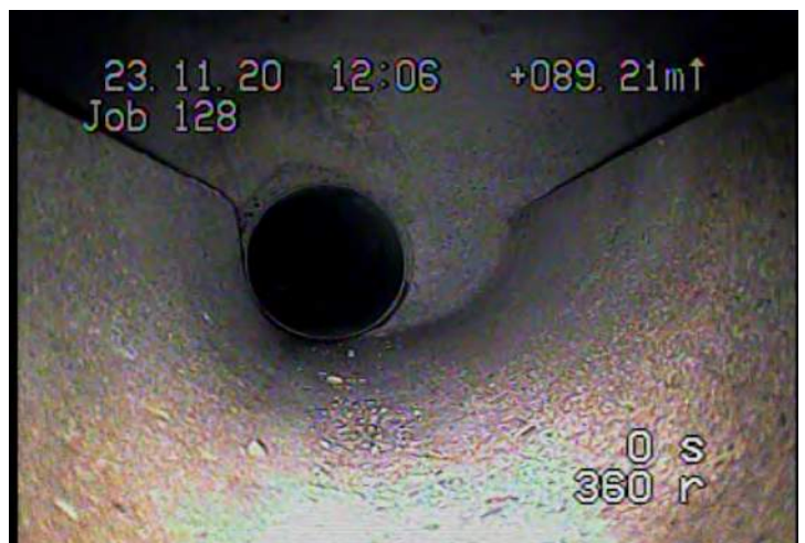
AMH - Access Point - Manhole @ 89.2 m. ST MH 9
