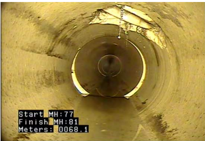
RFC - Roots, Fine: Connection @ 68.1 m.
