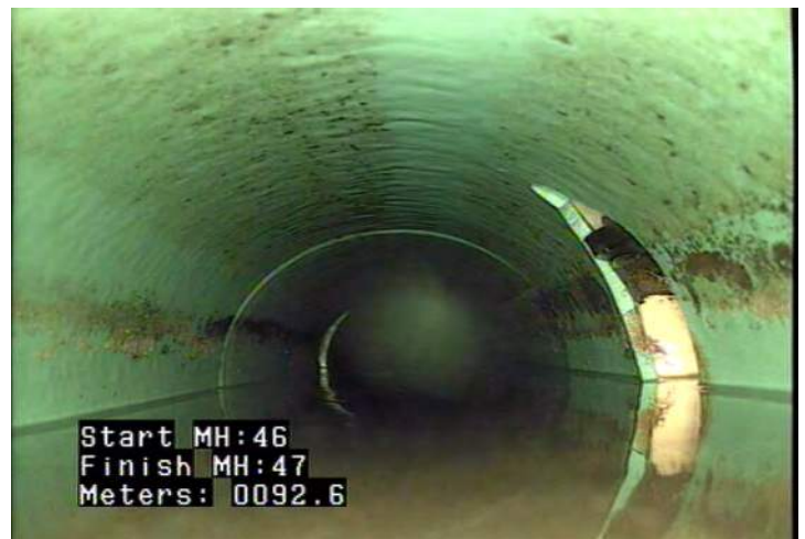
TSD - Tap, Saddle: Defective @ 92.6 m. Service offset from hole cut in pipe.
