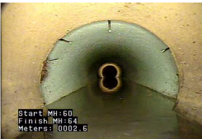
RPR - Point Repair - Pipe Replaced @ 2.6 m. PVC MSC - Dimension/Shape Change @ 5.3 m.
