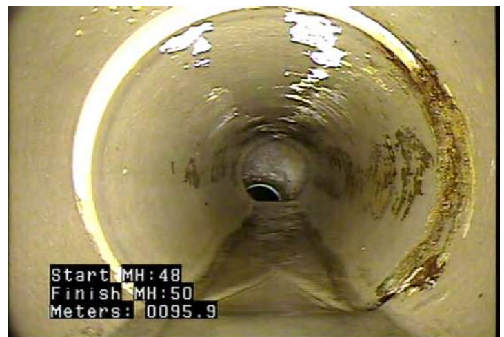
DAE - Deposits Attached: Encrustation @ 95.9 m.
