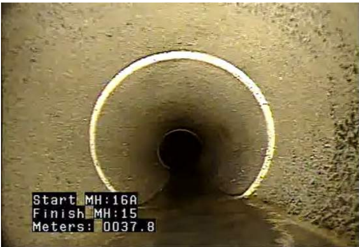
MWLS - Water Level: Sag @ 37.8 m.
