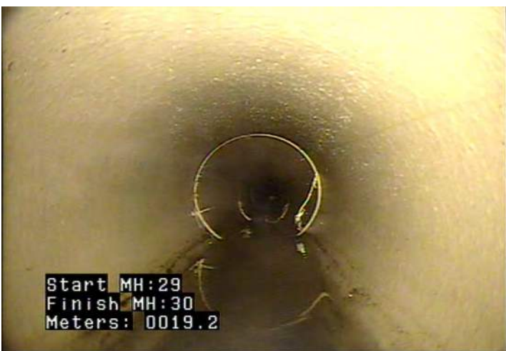
MSA - Survey Abandoned @ 19.2 m. Unable to pass rock wedged in joint.
