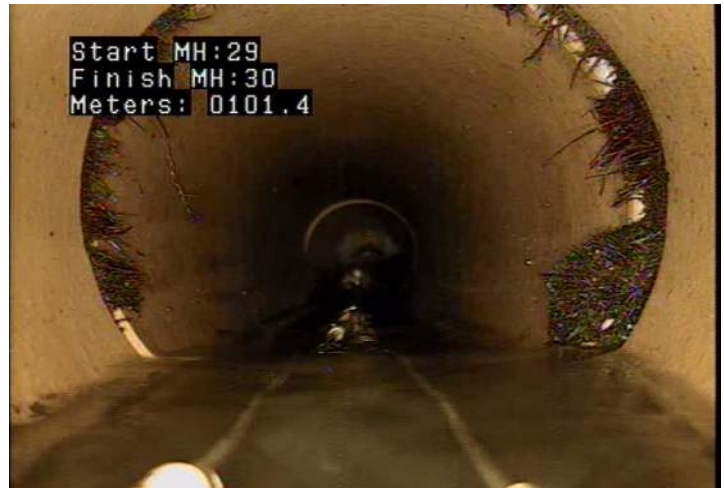
RMJ - Roots, Medium, Joint @ 101.4 m.
