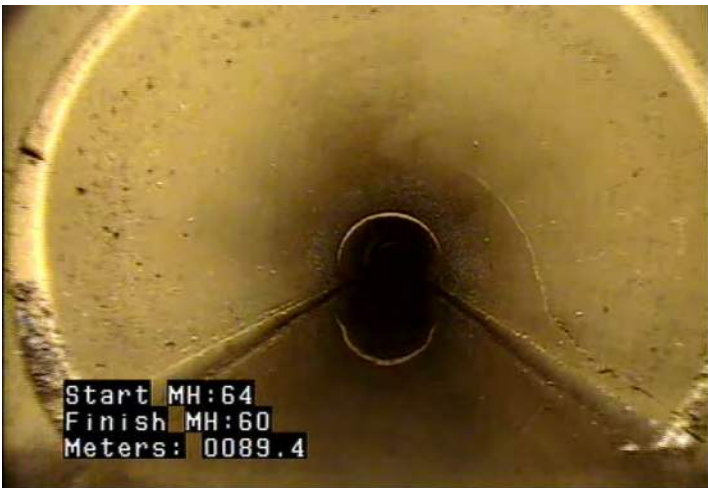
CS - Crack Spiral @ 89.4 m.
