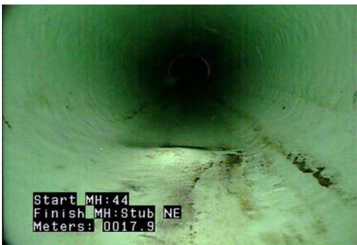
D - Pipe Deformed @ 17.9 m.
