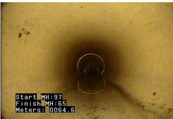
MWLS - Water Level: Sag @ 64.6 m.
