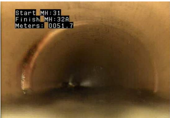
DAE - Deposits Attached: Encrustation @ 51.7 m.
