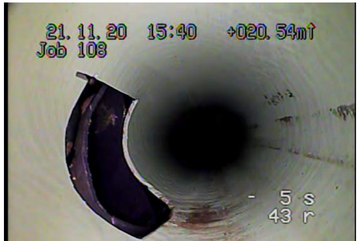
TSD - Tap, Saddle: Defective @ 20.5 m.
