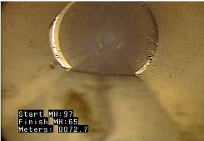
H - Hole in Pipe @ 72.7 m. Piece missing at joint
