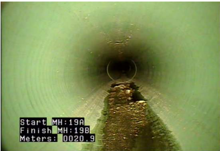
DSGV - Deposits Settled: Gravel @ 20.9 m.
