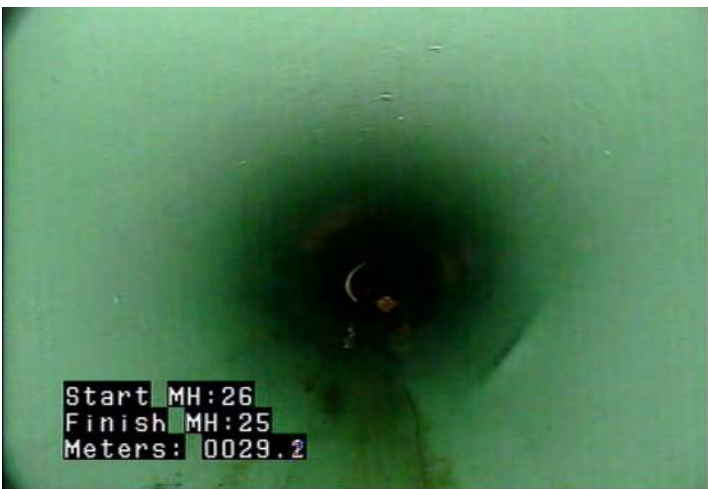
D - Pipe Deformed @ 29.2 m.
