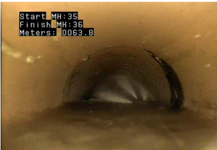
DAGS - Deposits Attached: Grease @ 63.8 m.
