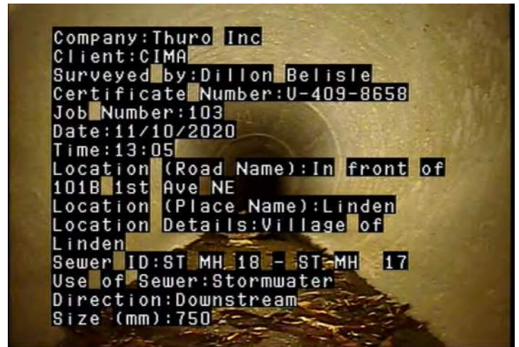
DSGV - Deposits Settled: Gravel @ 0.0 m.
