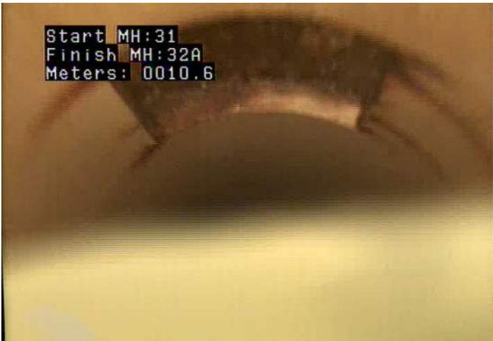
H - Hole in Pipe @ 10.6 m. Cut into pipe
