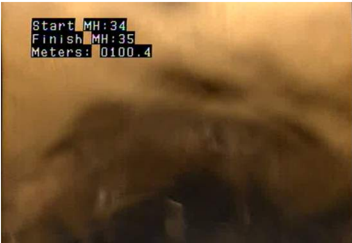
RMJ - Roots, Medium, Joint @ 100.4 m.
