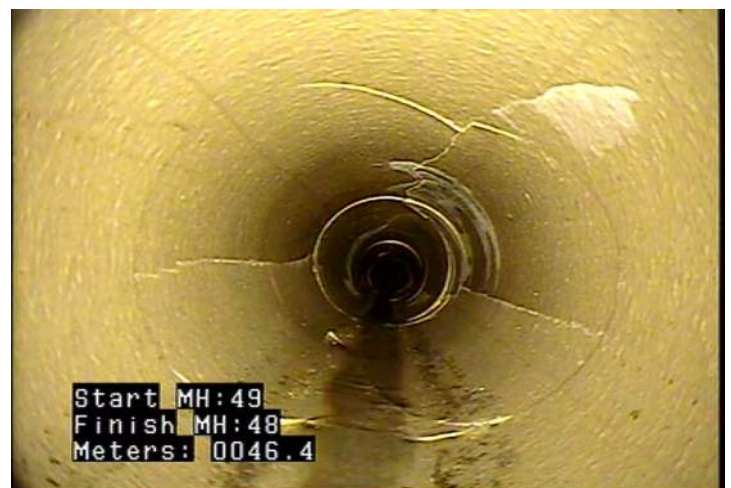
FM - Fracture Multiple @ 46.4 m.
