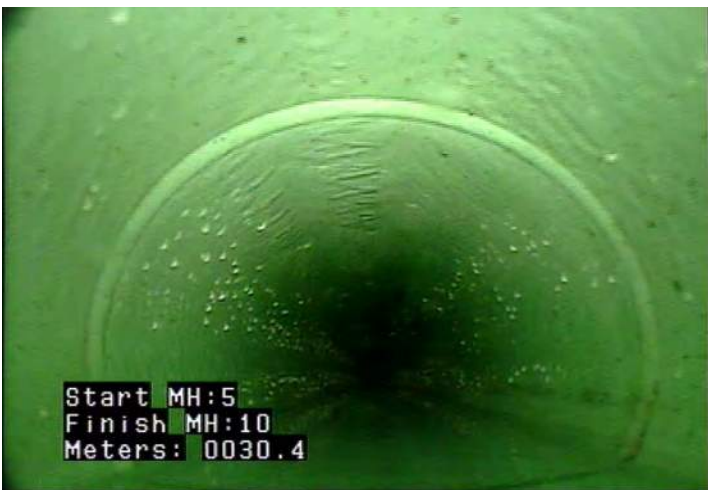
MWLS - Water Level: Sag @ 30.4 m.
