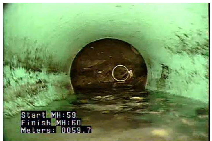
DSGV - Deposits Settled: Gravel @ 59.7 m.
