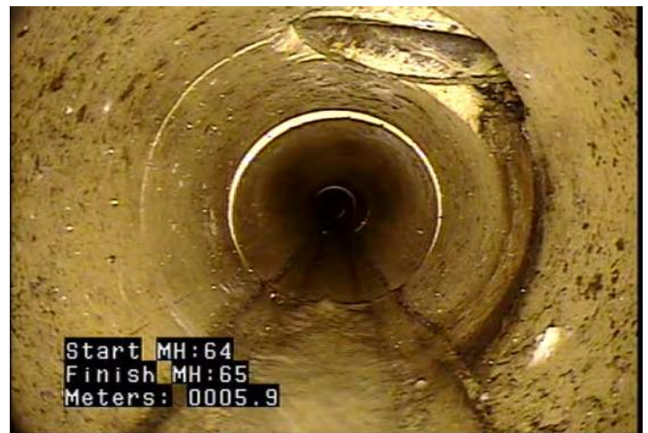
TB - Tap, Break-in / Hammer @ 5.9 m.
