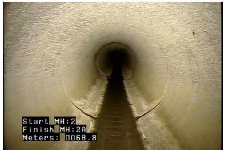
CC - Crack Circumferential @ 68.8 m.
