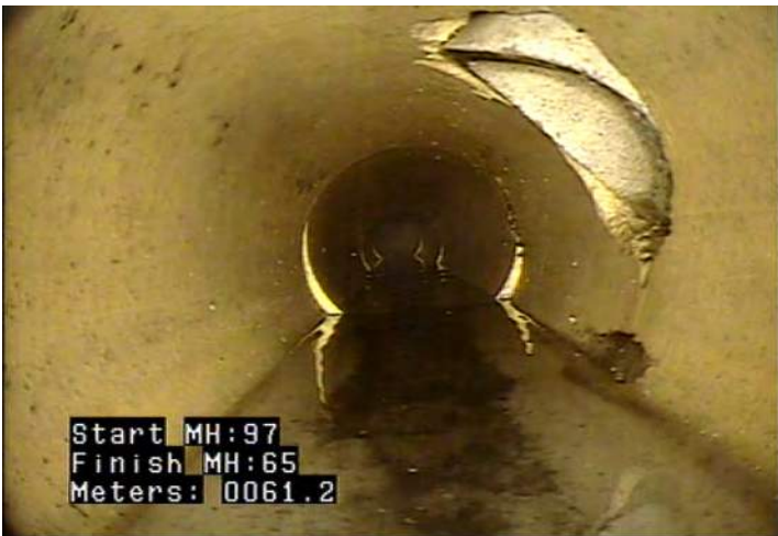
TB - Tap, Break-in / Hammer @ 61.2 m.
