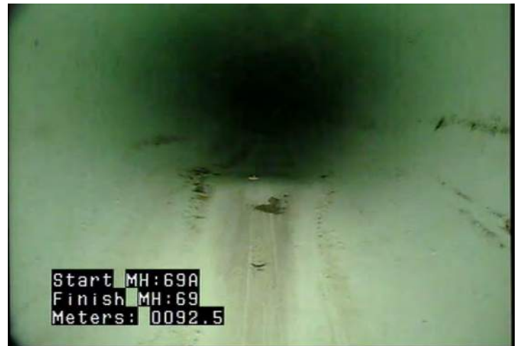
D - Pipe Deformed @ 92.5 m.
