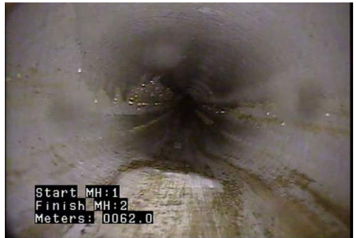
D - Pipe Deformed @ 62.0 m.
