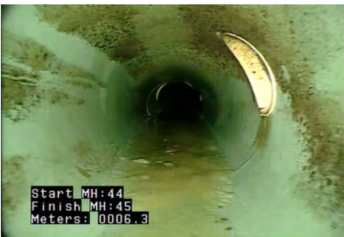
MWLS - Water Level: Sag @ 6.3 m.
