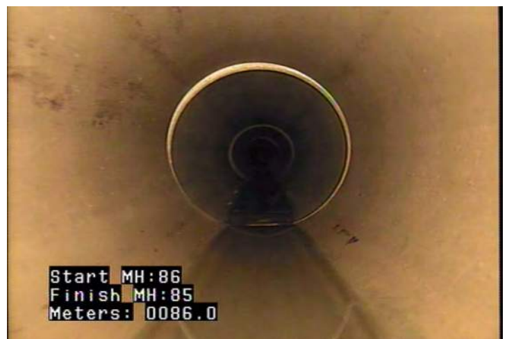
MWLS - Water Level: Sag @ 86.0 m.
