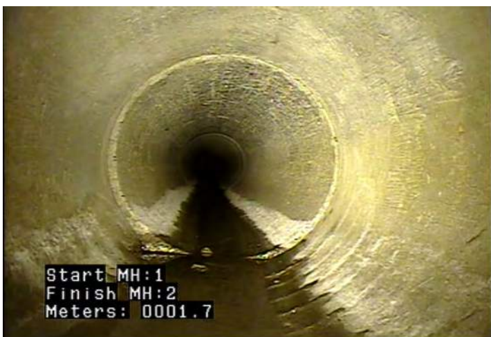
SRP - Surface: Reinforcement Projecting @ 1.7 m.
