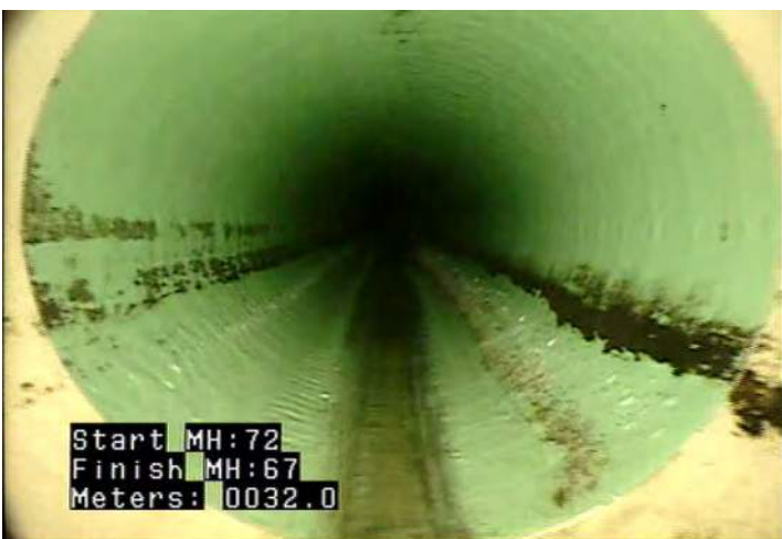
MMC - Material Change @ 32.0 m. White to Blue PVC
