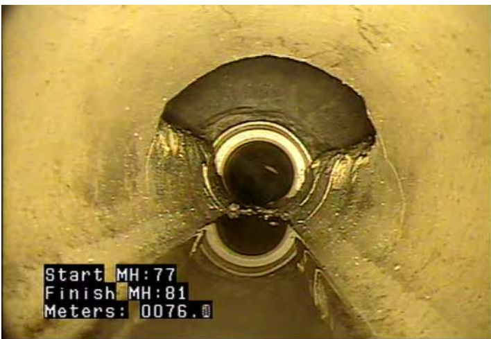
CS - Crack Spiral @ 76.0 m.
