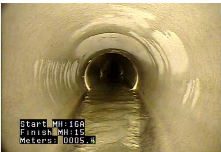
MWLS - Water Level: Sag @ 5.5 m.
