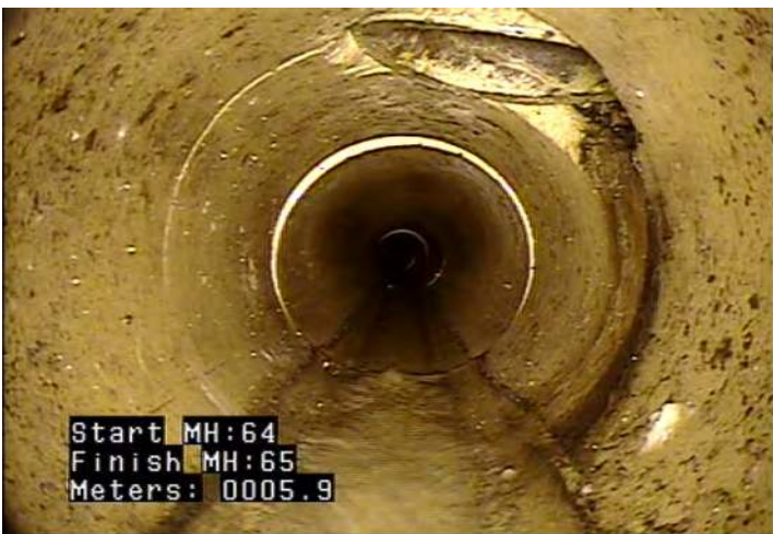
CC - Crack Circumferential @ 5.9 m.
