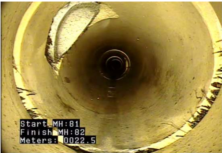
RFC - Roots, Fine: Connection @ 22.5 m.
