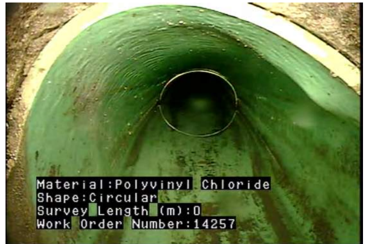
MWLS - Water Level: Sag @ 0.5 m.
