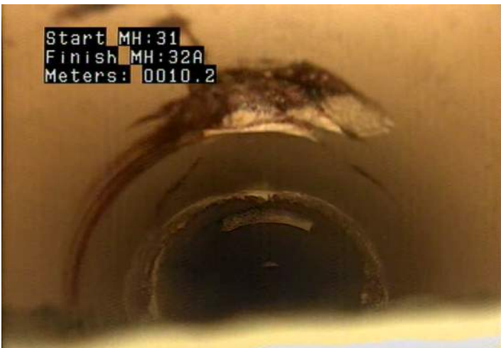
H - Hole in Pipe @ 10.2 m.
