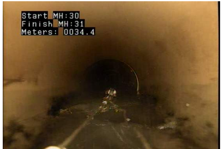
MWLS - Water Level: Sag @ 34.4 m.
