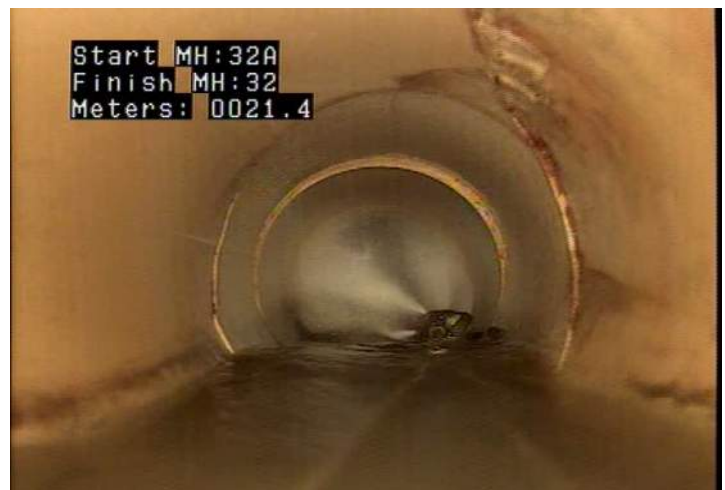
FM - Fracture Multiple @ 21.4 m.
