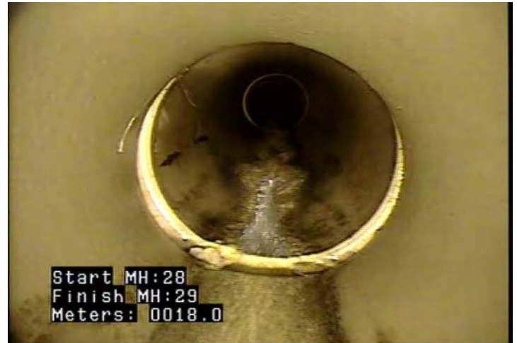
JAM - Joint Angular: Medium @ 18.0 m.
