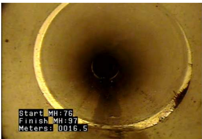
RFJ - Roots, Fine: Joint @ 16.5 m. Fine roots at most joints throughout ipe from 16.5 - 52.4
