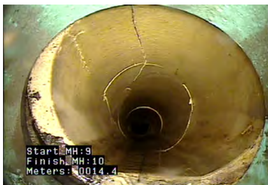
FM - Fracture Multiple @ 14.4 m. Rest of line observed with camera zoom to S MH 10. First length of clay tile line full of fractures. Second length fine. Joint going into S MH 10 is offset large.
