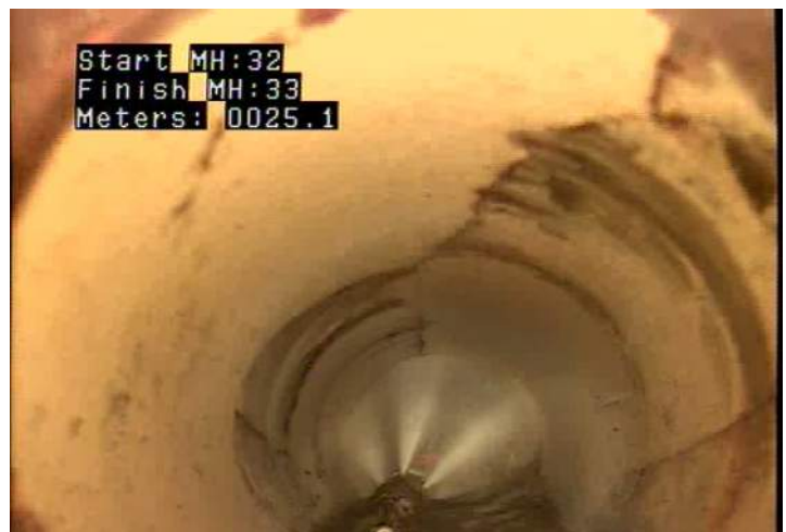
CM - Crack Multiple @ 25.1 m.
