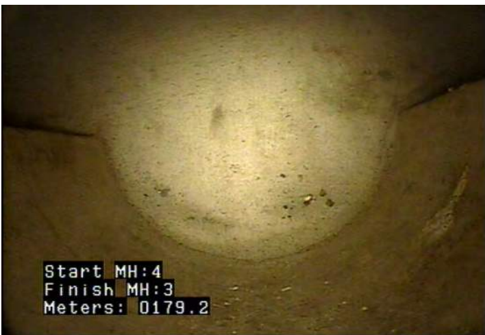
AMH - Access Point - Manhole @ 179.2 m. S MH 3 - Buried
