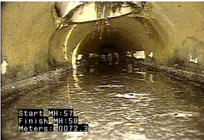
B - Pipe Broken @ 72.4 m. After tap
