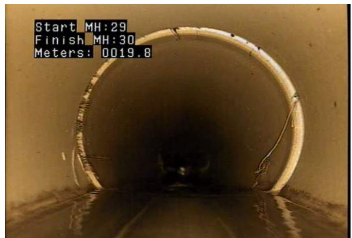
MWLS - Water Level: Sag @ 19.8 m.
