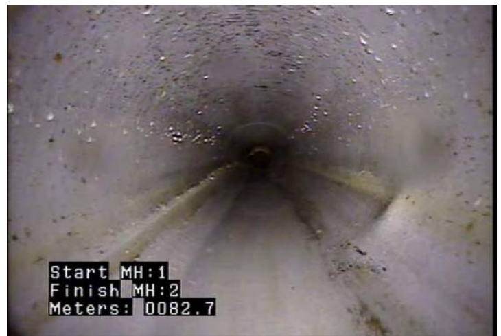
D - Pipe Deformed @ 82.7 m.
