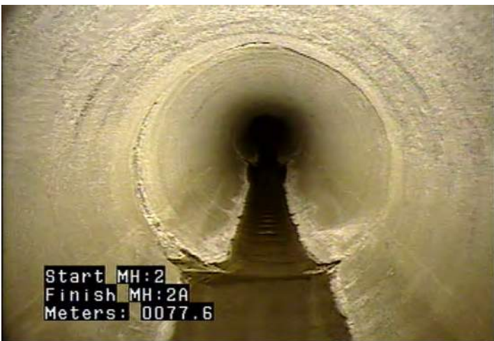
MGO - General Observation @ 77.6 m. Chipped joint 12:00
