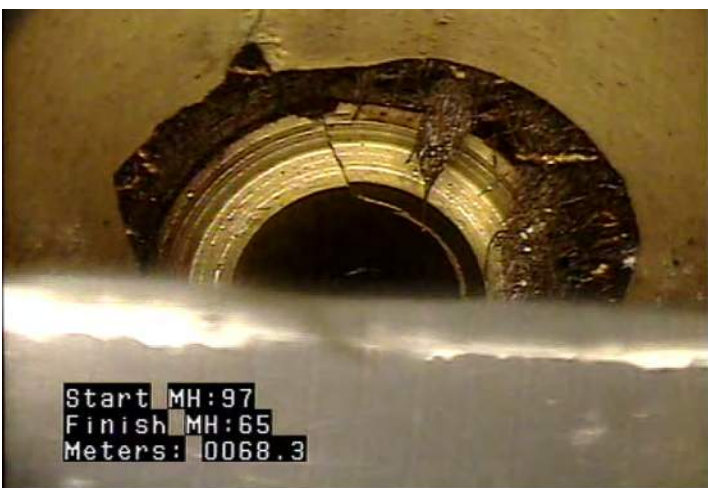
RMJ - Roots, Medium, Joint @ 68.3 m.
