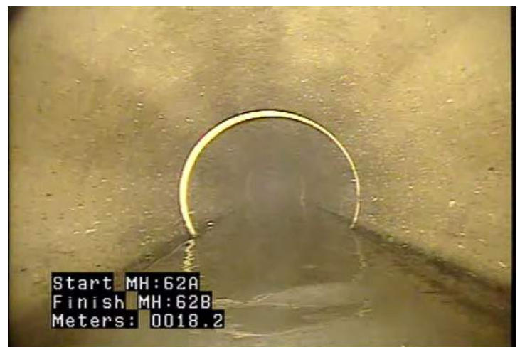
MWLS - Water Level: Sag @ 18.2 m.
