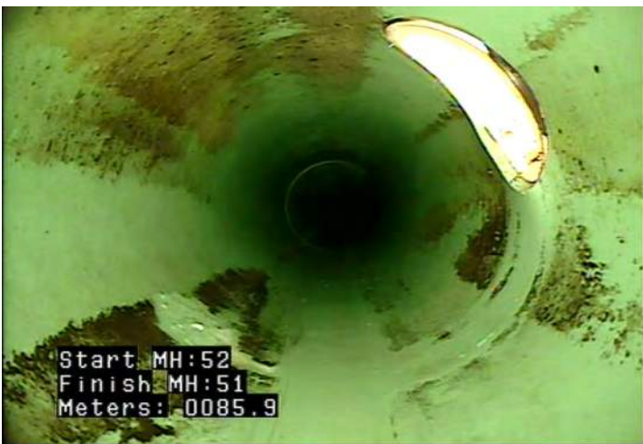
TSD - Tap, Saddle: Defective @ 85.9 m. Gasket visible around service.
