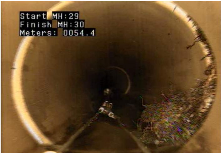
RMJ - Roots, Medium, Joint @ 54.4 m.
