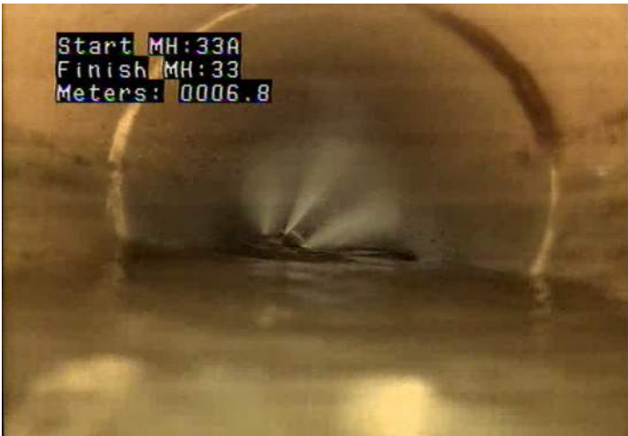
DAE - Deposits Attached: Encrustation @ 6.8 m.
