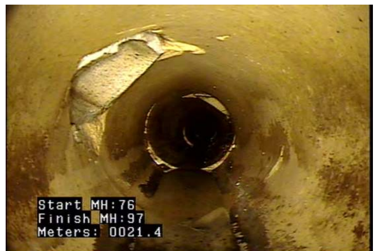
TB - Tap, Break-in / Hammer @ 21.4 m.
