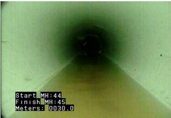
MWLS - Water Level: Sag @ 30.0 m.
