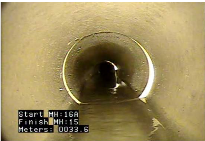
MWLS - Water Level: Sag @ 33.6 m.
