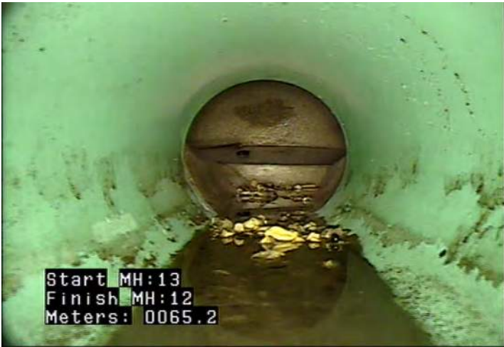
DSGV - Deposits Settled: Gravel @ 65.2 m.
