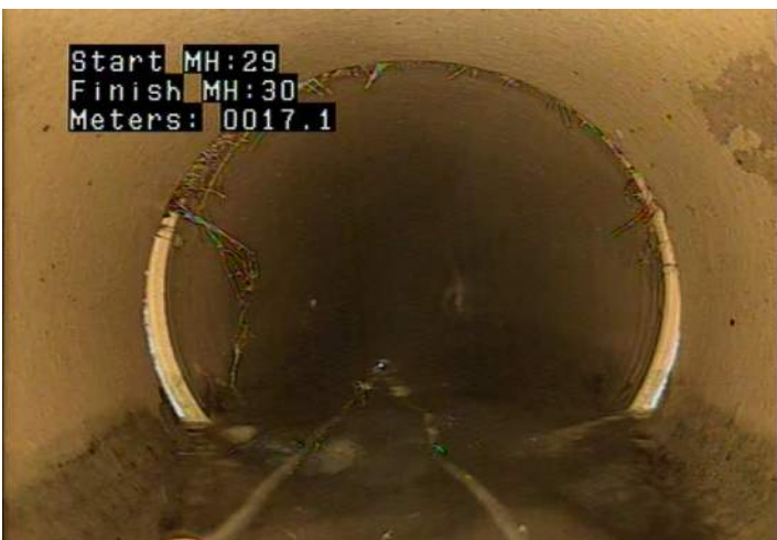
MWLS - Water Level: Sag @ 17.1 m.
