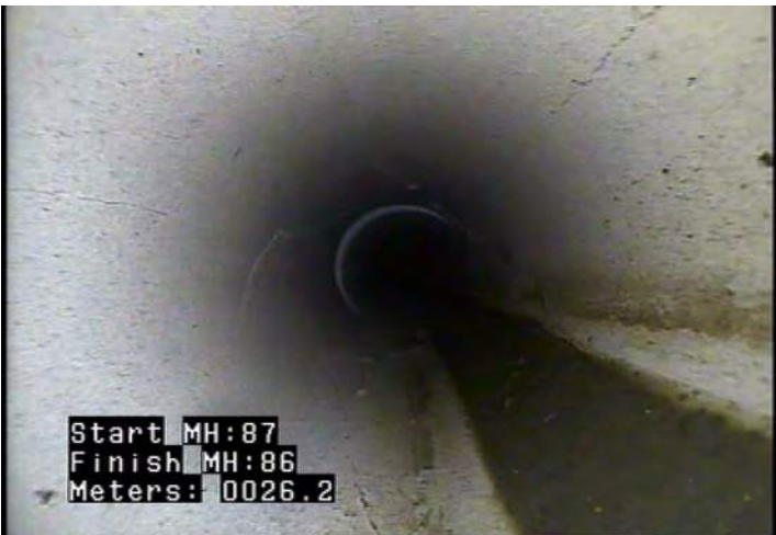
FM - Fracture Multiple @ 26.2 m.
