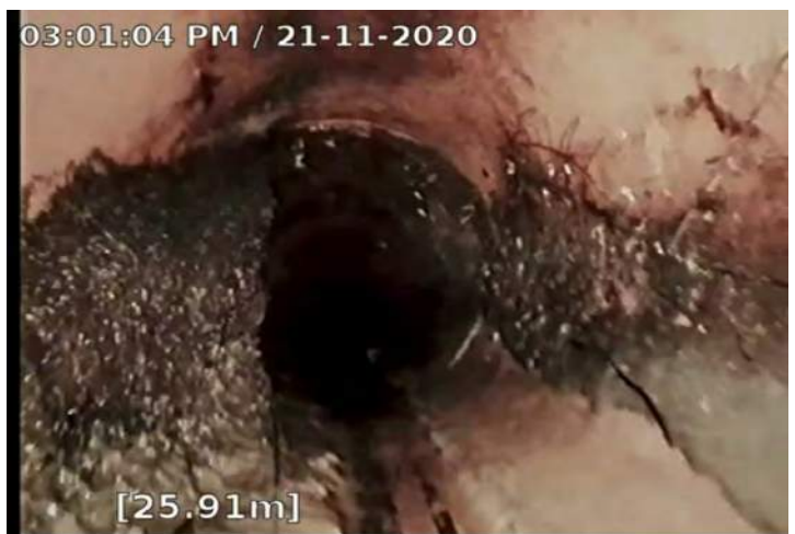
RMJ - Roots, Medium, Joint @ 25.9 m.
