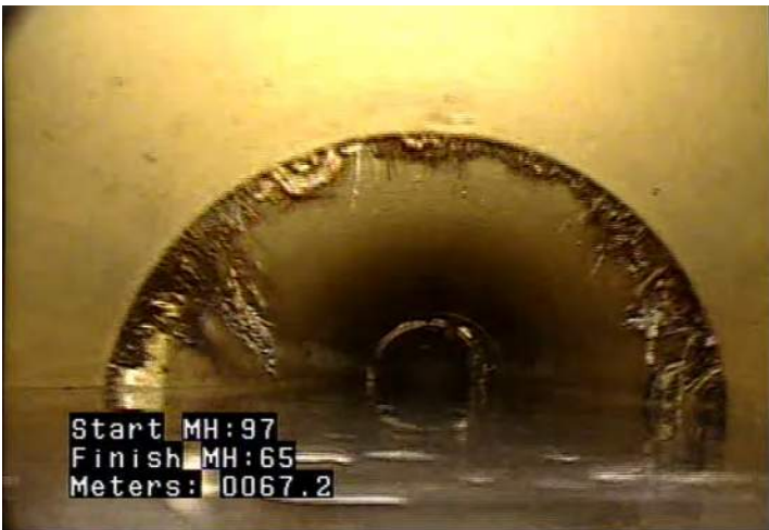
RMJ - Roots, Medium, Joint @ 67.2 m.
