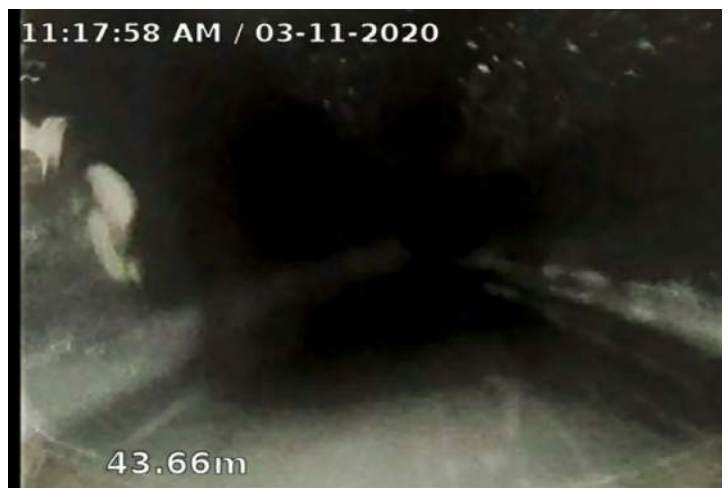
MMC - Material Change @ 43.7 m. Clay tile to ABS
