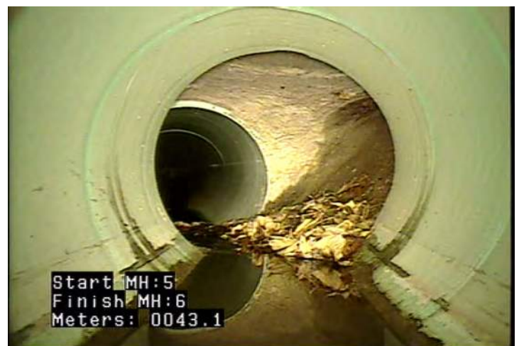
MWLS - Water Level: Sag @ 43.1 m.
