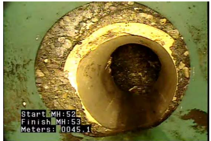
MMC - Material Change @ 45.1 m. PVC to Clay tile
