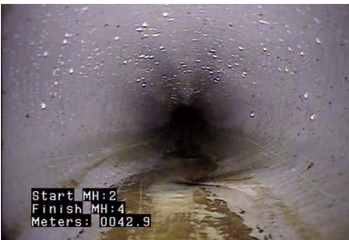
D - Pipe Deformed @ 42.9 m.
