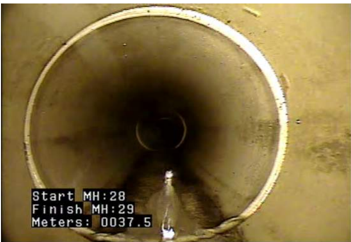
OBJ - Obstacle - Object Wedged in Joint @ 37.5 m. Fork wedged in joint
