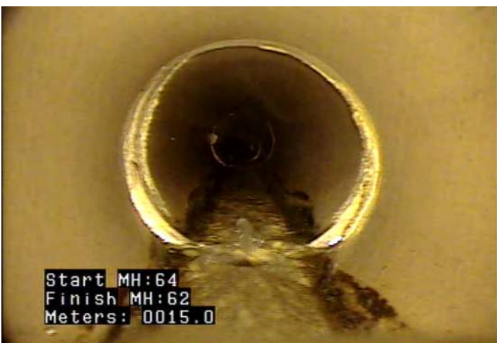
DAE - Deposits Attached: Encrustation @ 15.0 m.
