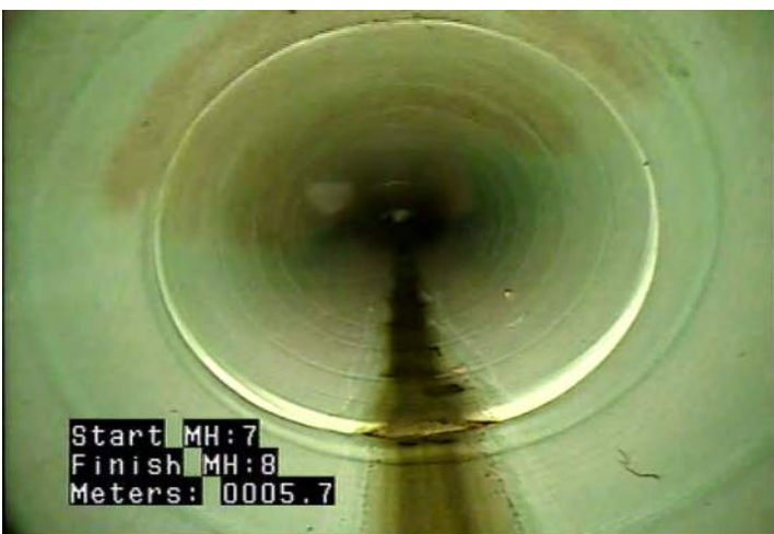
D - Pipe Deformed @ 5.7 m.
