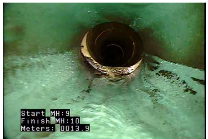
MWLS - Water Level: Sag @ 13.9 m.
