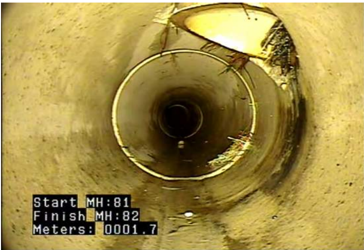
RFB - Roots, Fine: Barrel @ 1.7 m.
