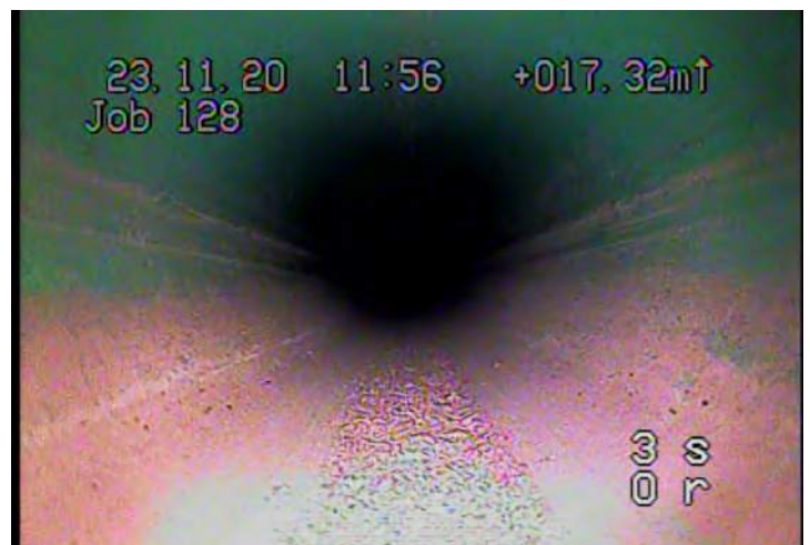
DSGV - Deposits Settled: Gravel @ 15.3 m.
