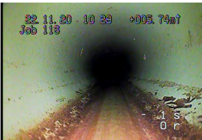
DAE - Deposits Attached: Encrustation @ 3.8 m.
