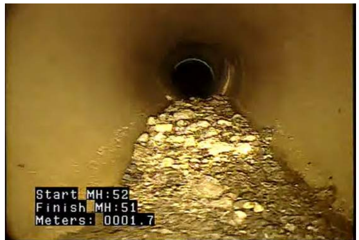
DSGV - Deposits Settled: Gravel @ 1.0 m.
