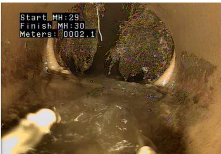
JOL - Joint Offset (displaced): Large @ 2.1 m.
