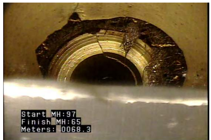
H - Hole in Pipe @ 68.3 m. Pipe missing at joint
