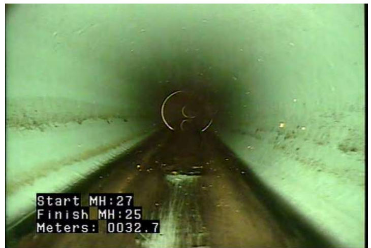
MWLS - Water Level: Sag @ 32.7 m.
