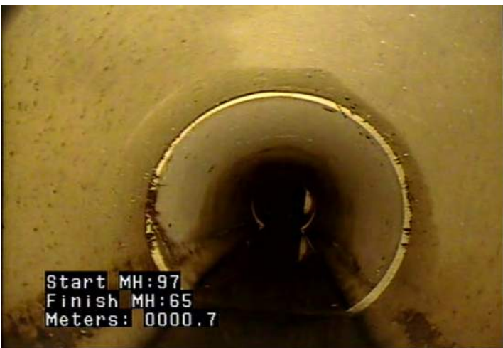
RFJ - Roots, Fine: Joint @ 0.7 m. Fine roots at most joints throughout pipe
