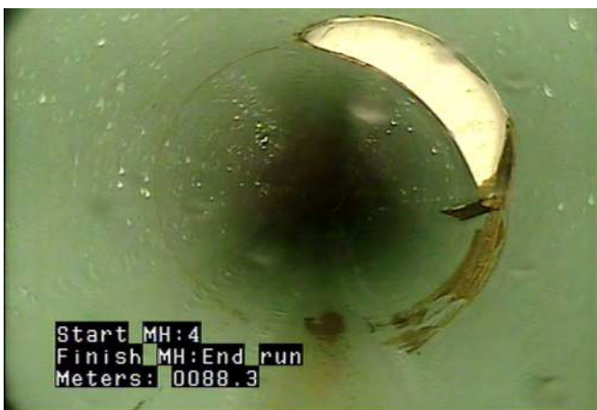
TSD - Tap, Saddle: Defective @ 88.3 m. Broken gasket intruding at bottom of service.
