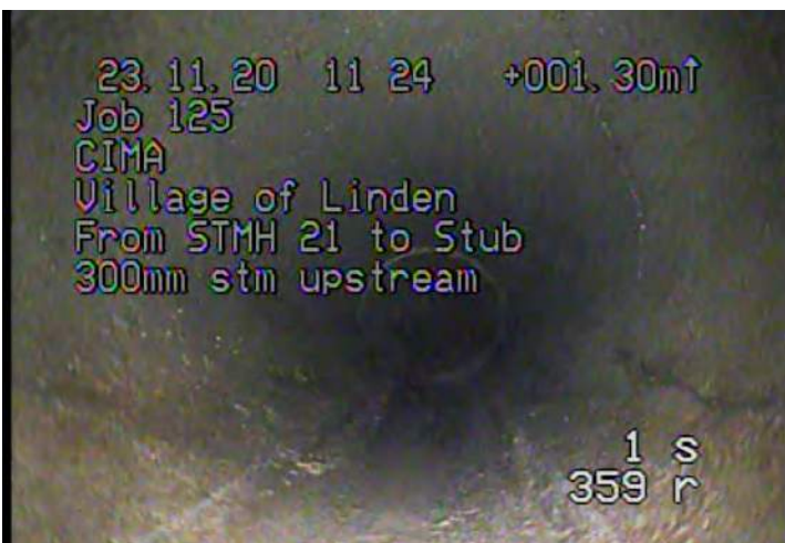
CM - Crack Multiple @ 0.5 m.
