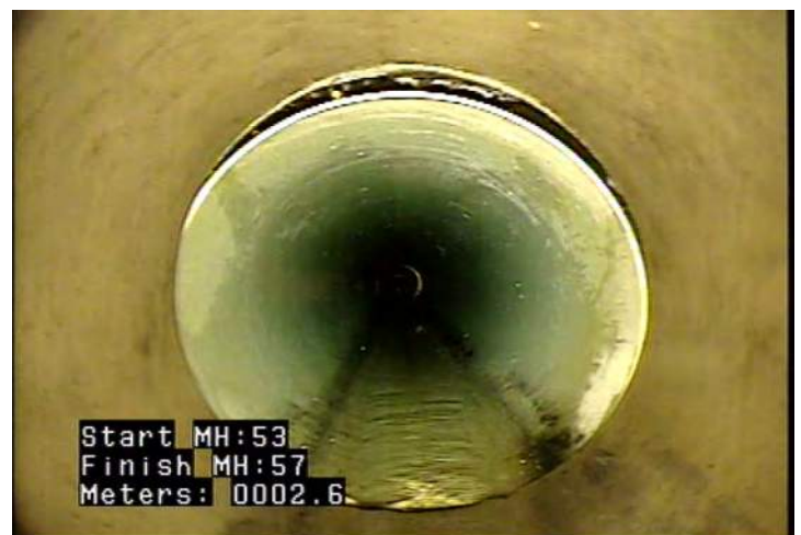
MMC - Material Change @ 2.6 m. Clay tile to PVC
