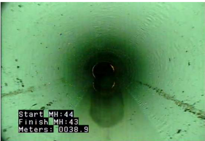
MWLS - Water Level: Sag @ 38.9 m.
