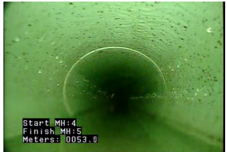
MWLS - Water Level: Sag @ 53.0 m.
