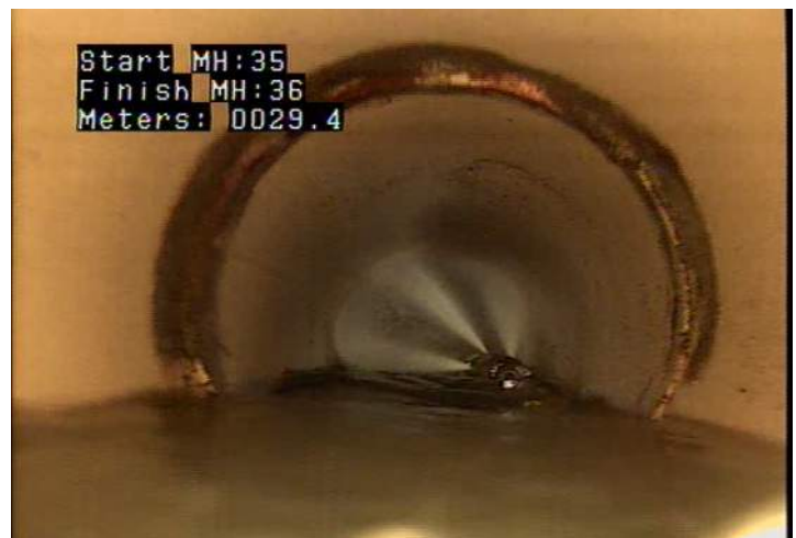
DAE - Deposits Attached: Encrustation @ 29.4 m.
