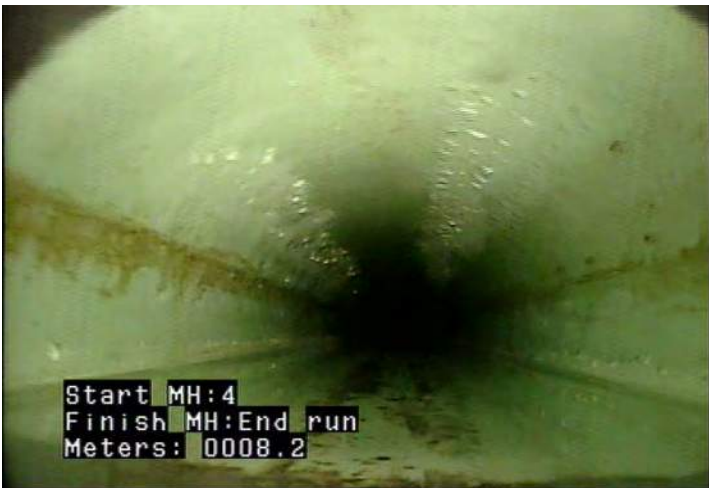
MMC - Material Change @ 8.2 m. Grey PVC to Blue PVC
