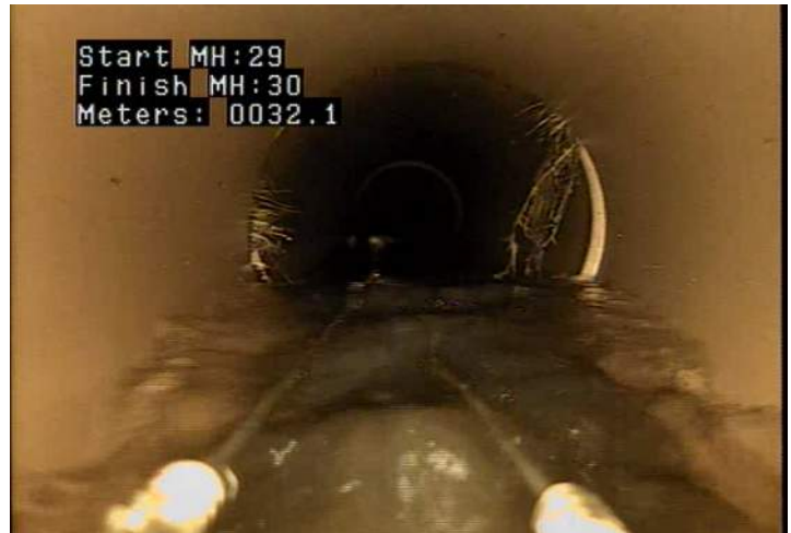
MWLS - Water Level: Sag @ 32.1 m.
