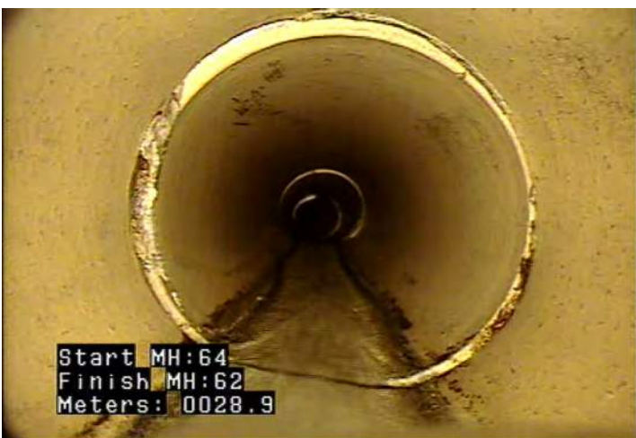
DAE - Deposits Attached: Encrustation @ 28.9 m.
