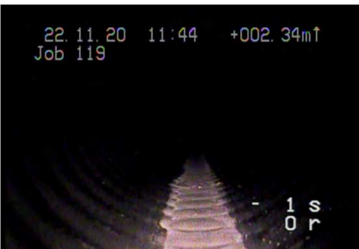
MMC - Material Change @ 2.0 m. PVC to Corrugated Plastic
