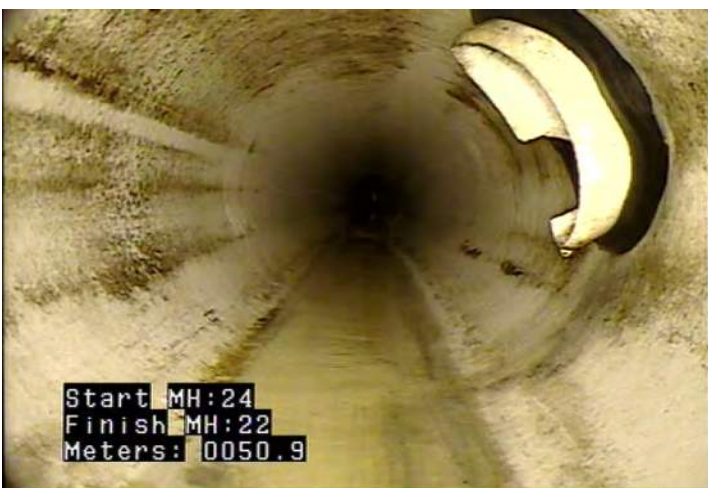
TSI - Tap, Saddle: Intruding @ 50.9 m. Broken
