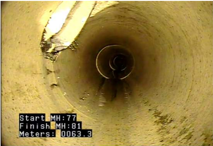
RFC - Roots, Fine: Connection @ 63.3 m.
