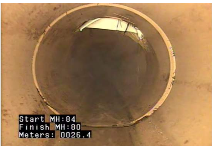
TB - Tap, Break-in / Hammer @ 26.4 m.
