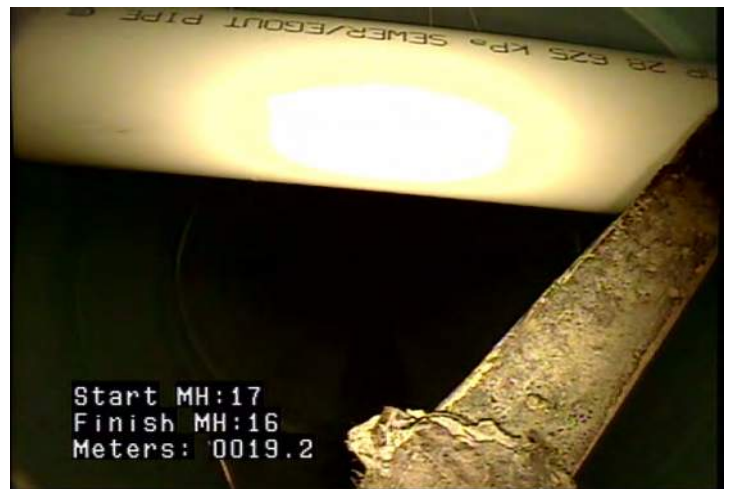
MSA - Survey Abandoned @ 19.2 m. Unable to pass pipe
