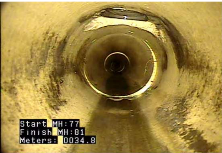
TB - Tap, Break-in / Hammer @ 34.8 m.
