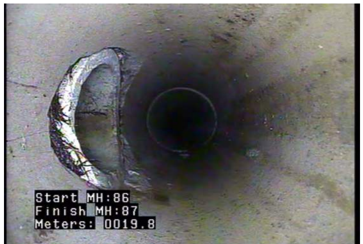
RFC - Roots, Fine: Connection @ 19.8 m.
