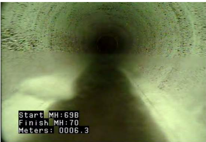
MWLS - Water Level: Sag @ 6.3 m.
