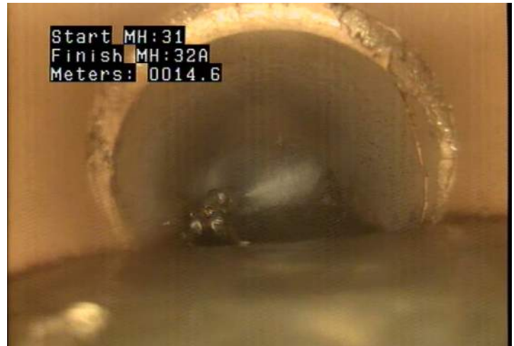
JOM - Joint Offset (displaced): Medium @ 14.6 m.
