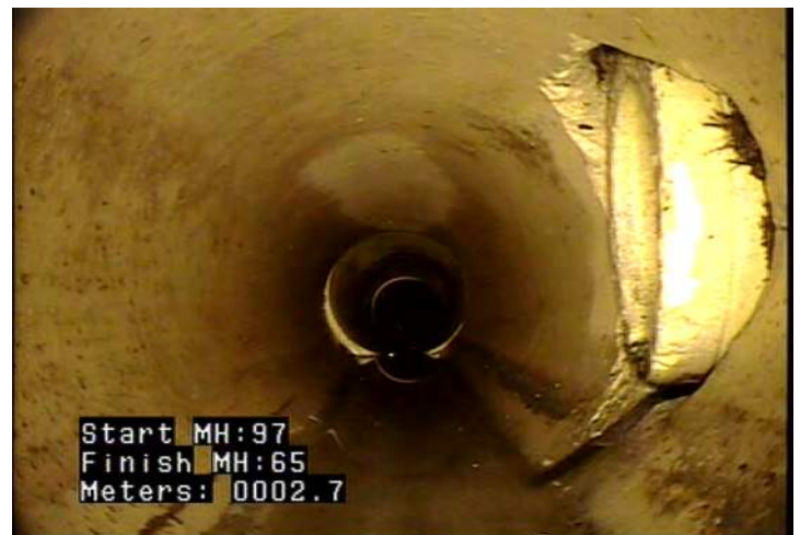
TB - Tap, Break-in / Hammer @ 2.7 m.
