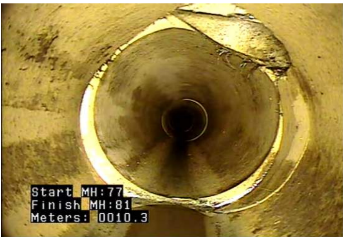
TB - Tap, Break-in / Hammer @ 10.3 m.
