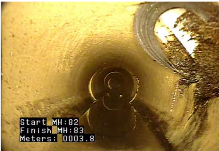
MWLS - Water Level: Sag @ 3.8 m.
