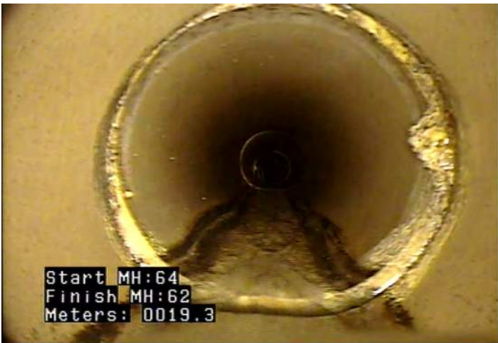
DAE - Deposits Attached: Encrustation @ 19.3 m.
