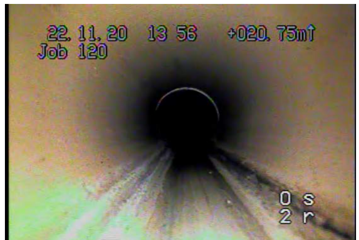
TBA - Tap, Break-in / Hammer: Active @ 25.2 m.
