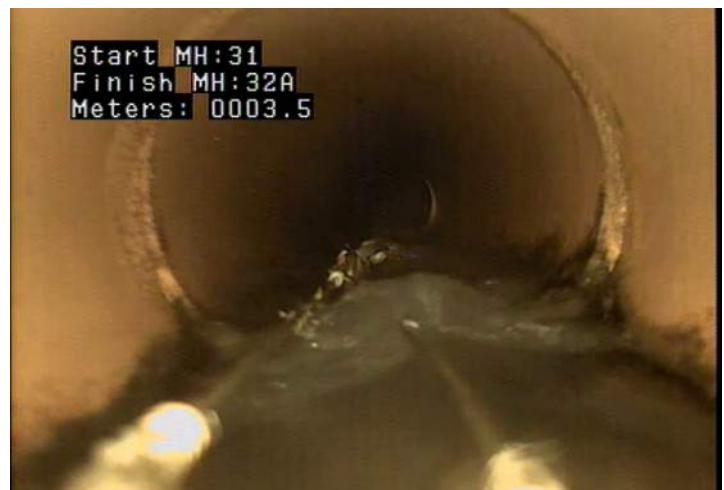
DAE - Deposits Attached: Encrustation @ 3.5 m.
