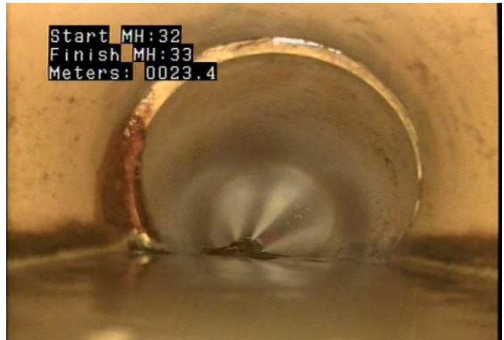
DAE - Deposits Attached: Encrustation @ 23.4 m.
