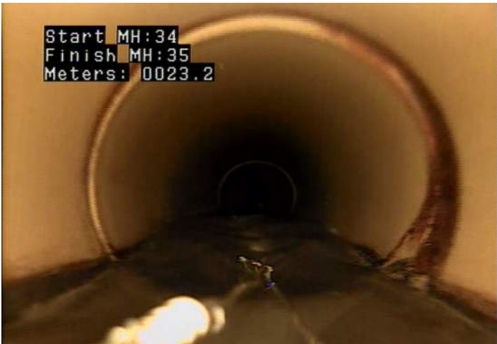
DAE - Deposits Attached: Encrustation @ 23.2 m.
