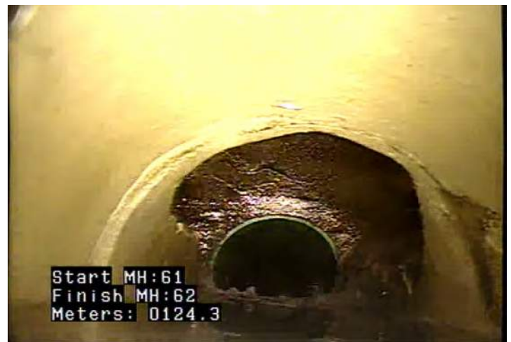
FC - Fracture Circumferential @ 124.3 m.
