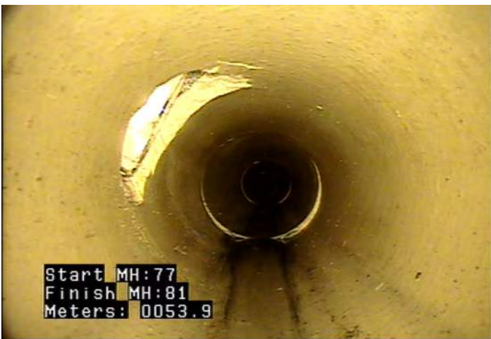
TB - Tap, Break-in / Hammer @ 53.9 m.
