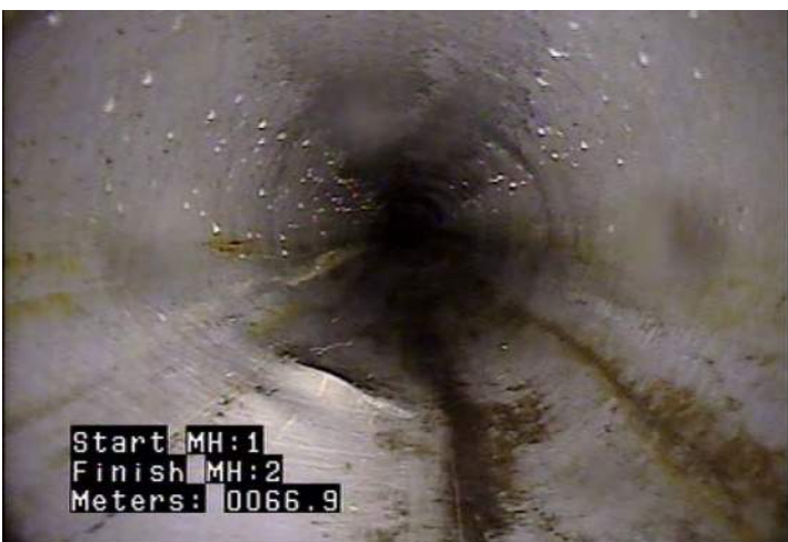
D - Pipe Deformed @ 66.9 m.
