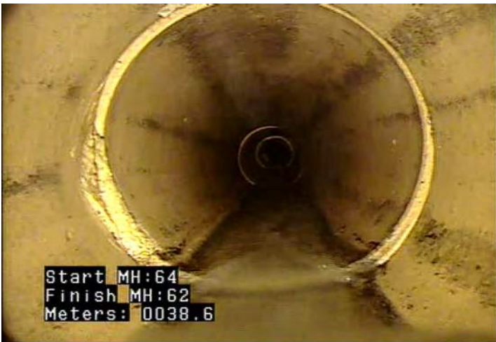
DAE - Deposits Attached: Encrustation @ 38.6 m.
