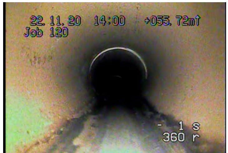
RMJ - Roots, Medium, Joint @ 54.8 m.
