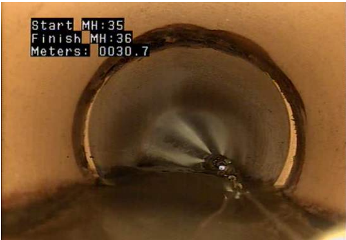
DAE - Deposits Attached: Encrustation @ 30.7 m.
