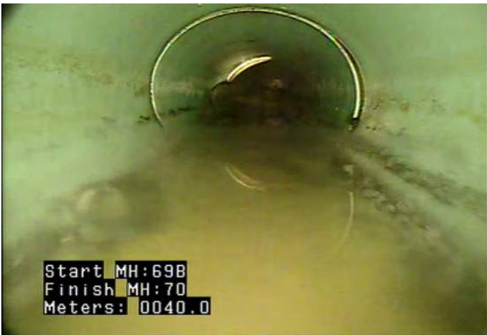
D - Pipe Deformed @ 40.0 m. Oval
