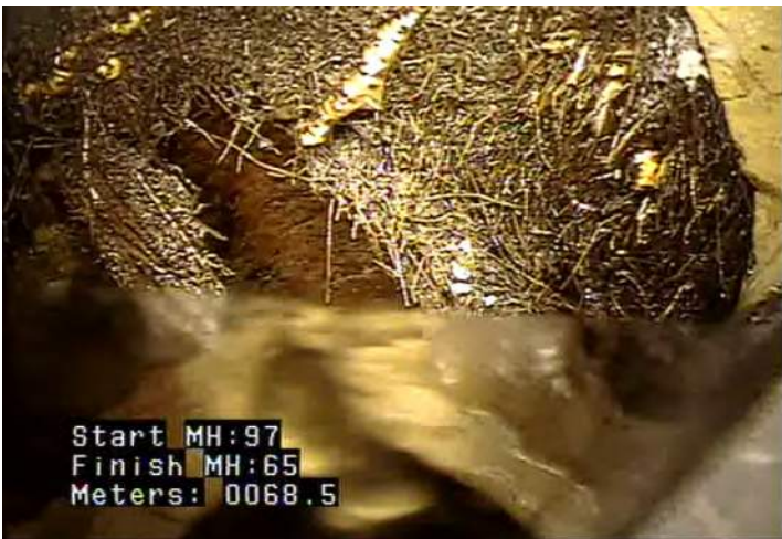
FS - Fracture Spiral @ 68.5 m. Fracture visible in pipesegment after hole
