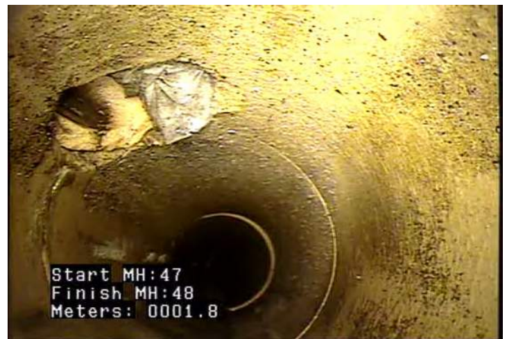
CC - Crack Circumferential @ 1.8 m.
