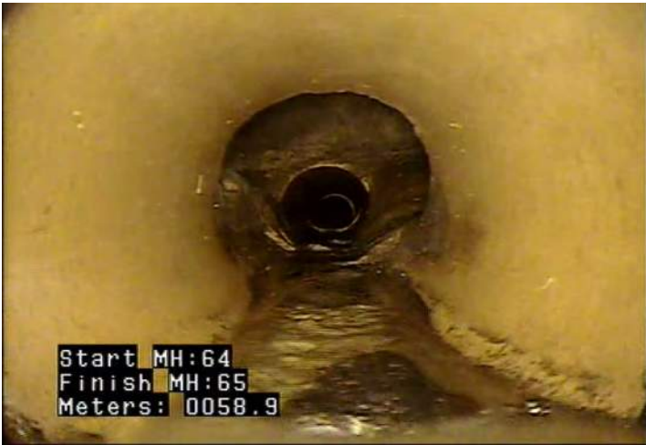
DSGV - Deposits Settled: Gravel @ 58.9 m.
