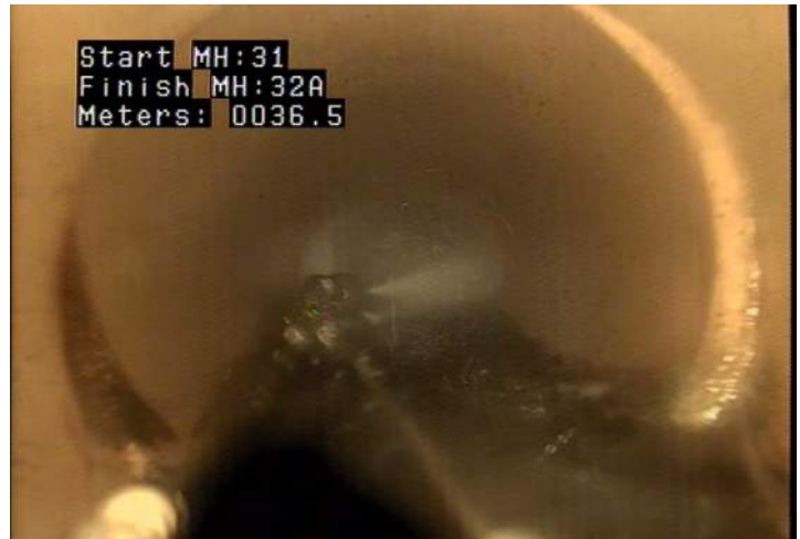
DAE - Deposits Attached: Encrustation @ 36.5 m.
