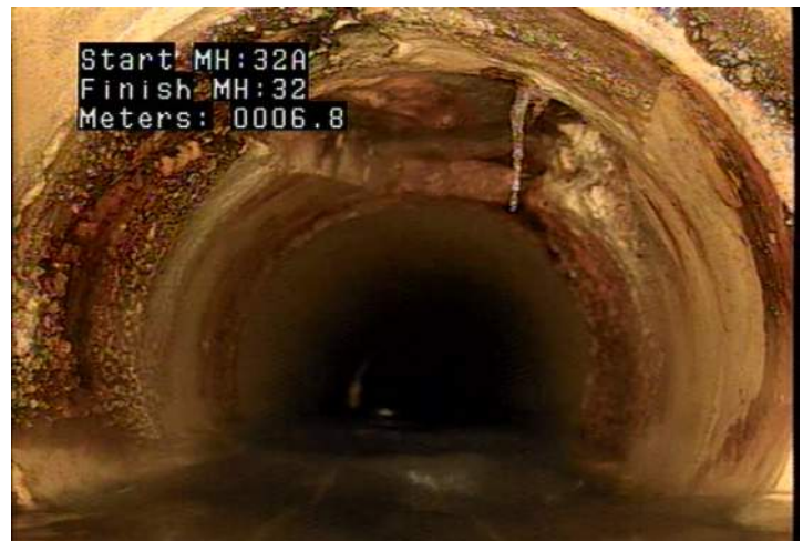
ID - Infiltration - Dripper @ 6.8 m.
