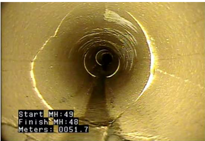
B - Pipe Broken @ 51.7 m.
