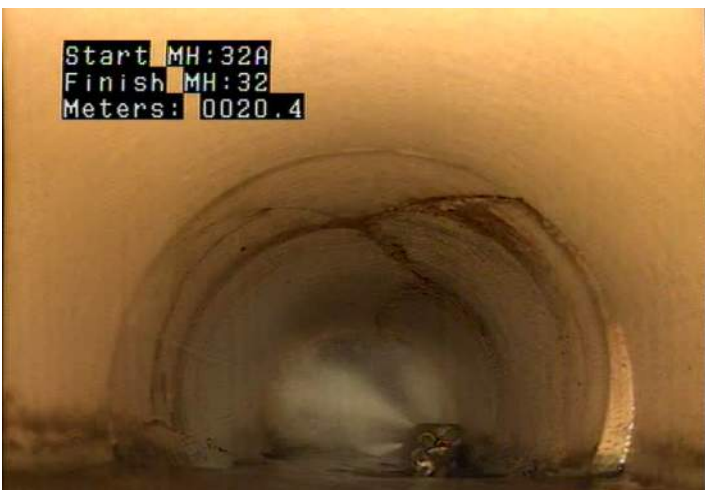
CM - Crack Multiple @ 20.4 m.
