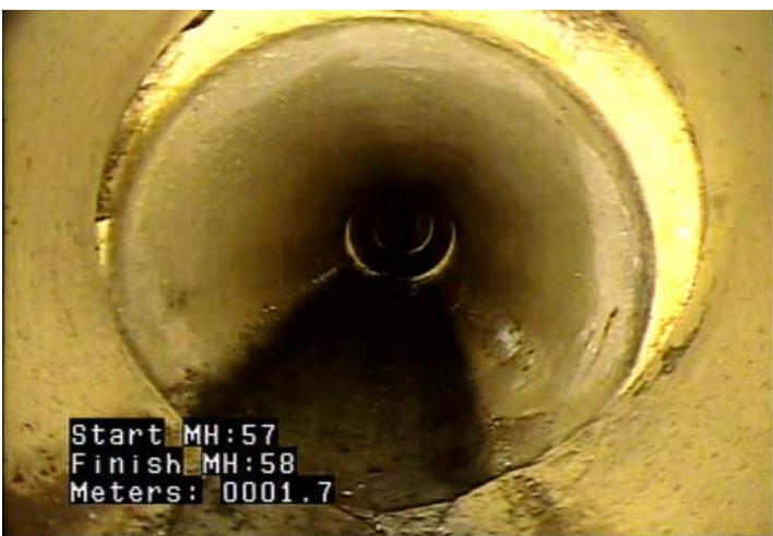
JOL - Joint Offset (displaced): Large @ 1.7 m.
