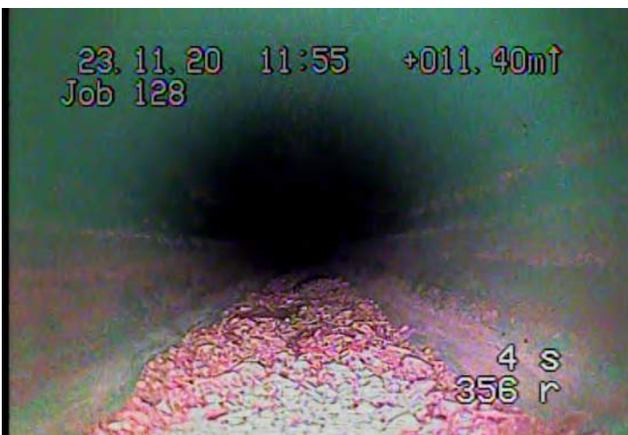
DSGV - Deposits Settled: Gravel @ 9.9 m.
