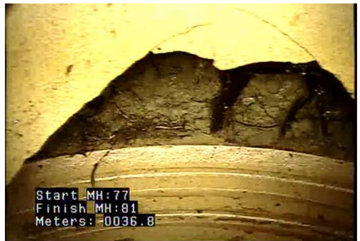
MGP - General Photograph @ 36.8 m. Additional view of hole at joint
