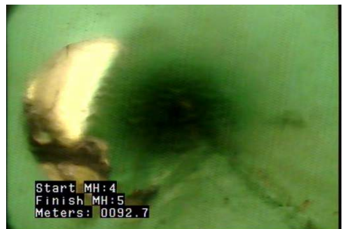
TSD - Tap, Saddle: Defective @ 92.7 m. Gasket at bottom of service holding back debris.
