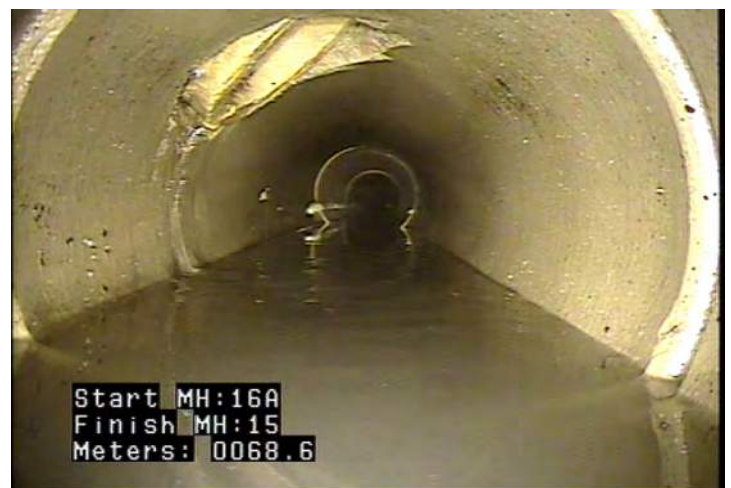
TB - Tap, Break-in / Hammer @ 68.6 m.
