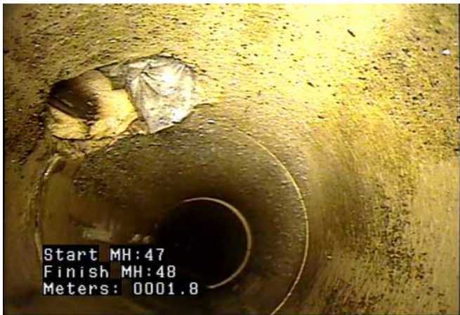
TBD - Tap, Break-in / Hammer: Defective @ 1.8 m. Plastic intruding from top of service.
