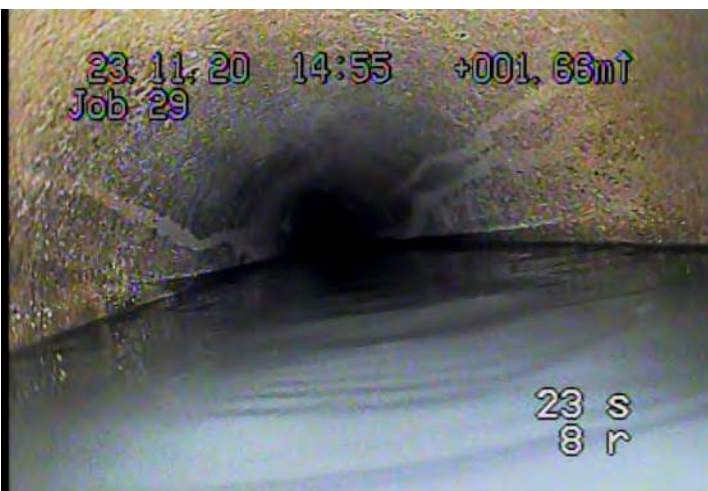
DSGV - Deposits Settled: Gravel @ 1.6 m.
