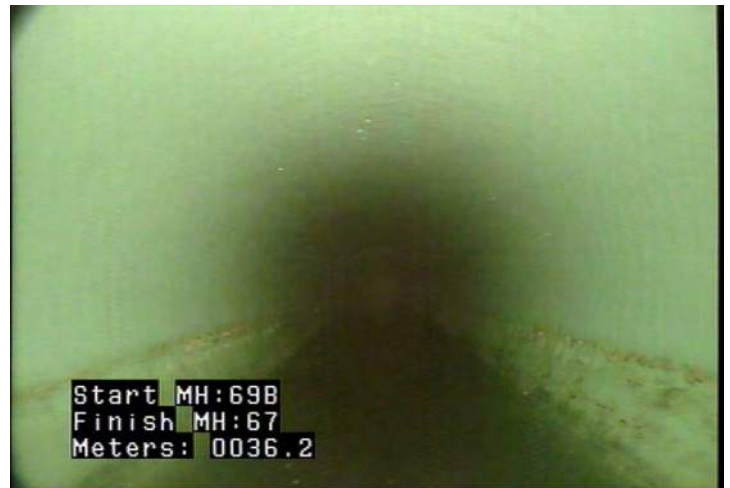
MWLS - Water Level: Sag @ 36.2 m.
