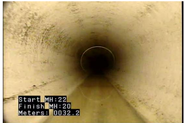
MWLS - Water Level: Sag @ 32.2 m.
