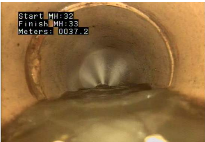
DAE - Deposits Attached: Encrustation @ 37.2 m.
