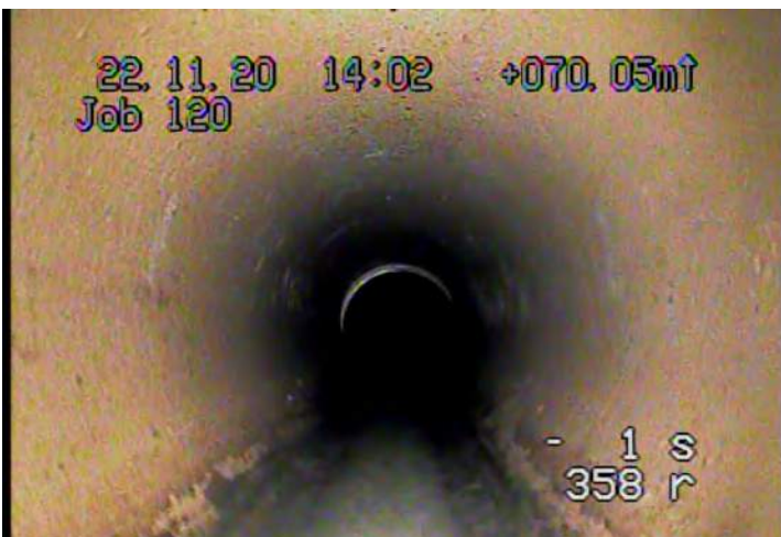
JOL - Joint Offset (displaced): Large @ 69.0 m.
