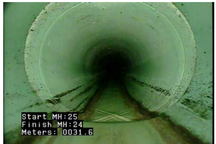
MWLS - Water Level: Sag @ 31.6 m.
