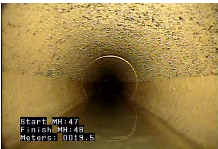
MWLS - Water Level: Sag @ 19.5 m.
