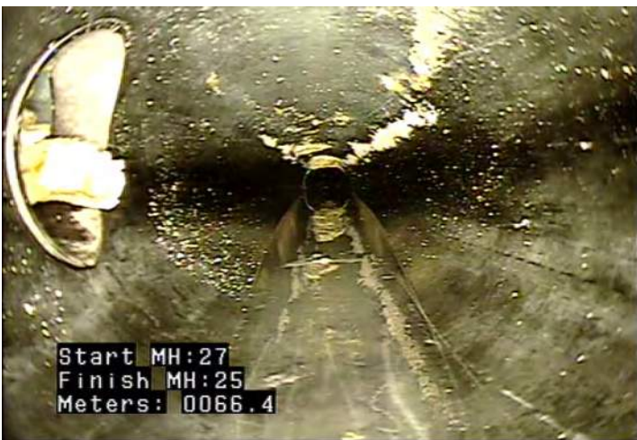
TSD - Tap, Saddle: Defective @ 66.4 m. Full of grease.
