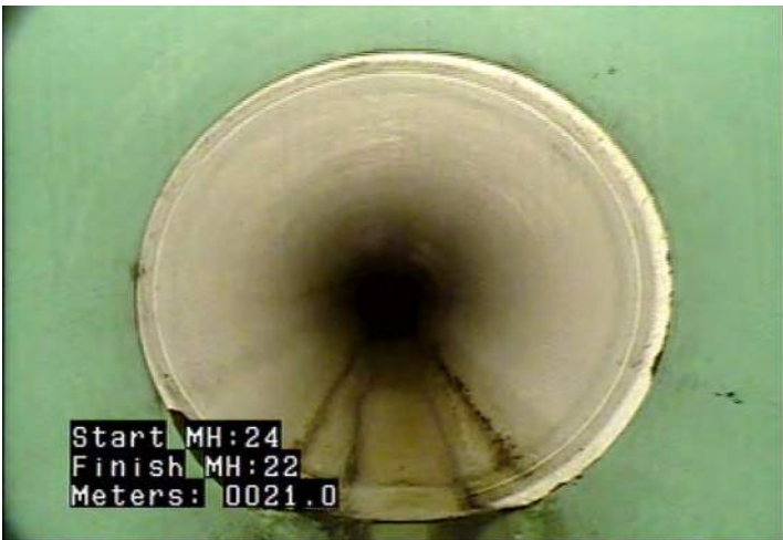
MMC - Material Change @ 21.0 m. Blue PVC to White PVC
