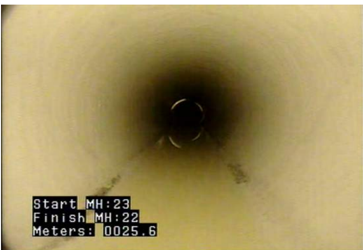
MWLS - Water Level: Sag @ 25.6 m.
