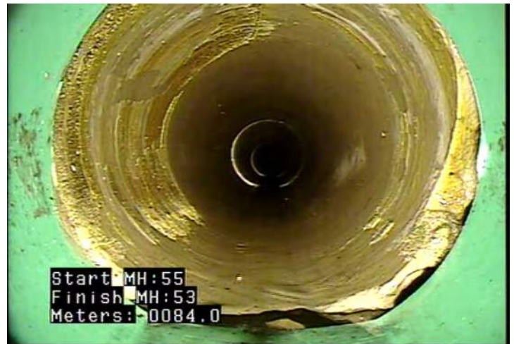
H - Hole in Pipe @ 84.0 m.
