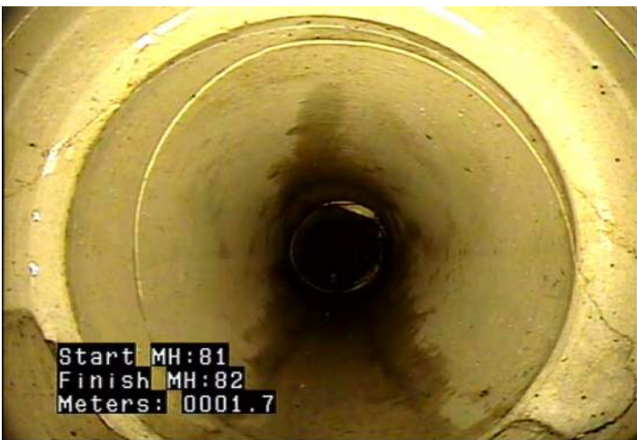
CS - Crack Spiral @ 0.5 m.
