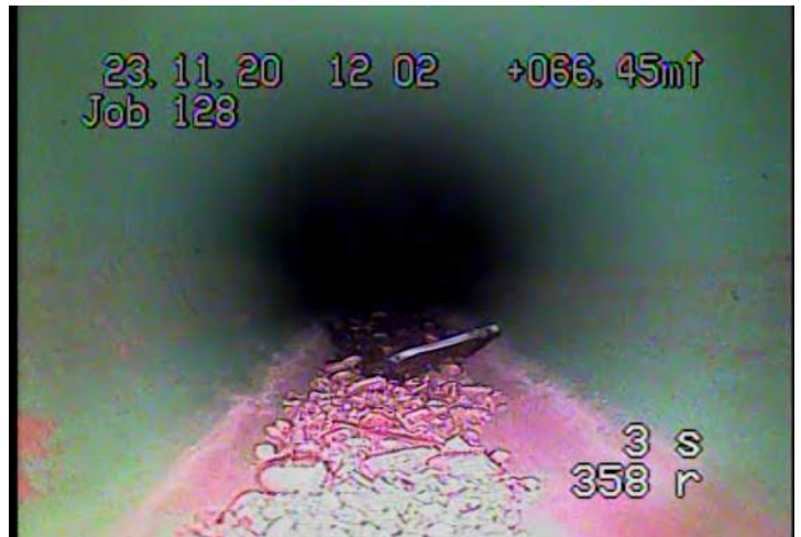
DSGV - Deposits Settled: Gravel @ 66.1 m.
