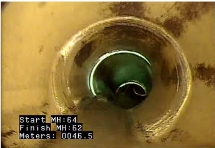
DAE - Deposits Attached: Encrustation @ 46.5 m.
