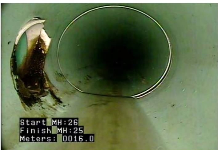
DAE - Deposits Attached: Encrustation @ 16.0 m.
