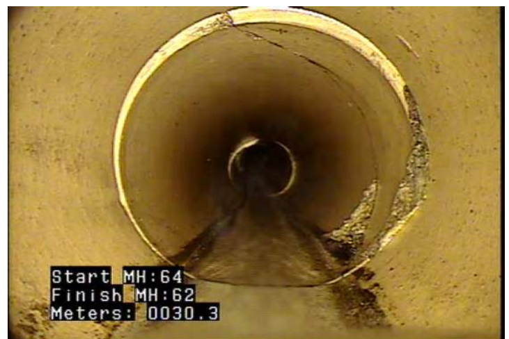
FC - Fracture Circumferential @ 30.3 m.
