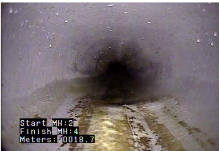
D - Pipe Deformed @ 18.7 m.
