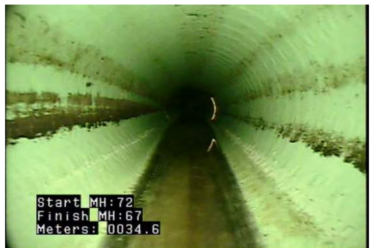
MWLS - Water Level: Sag @ 34.6 m.
