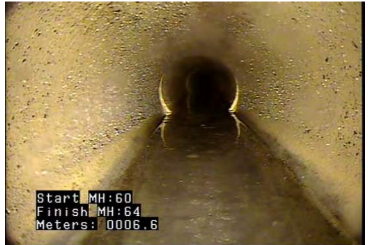
MSA - Survey Abandoned @ 6.6 m. Unable to pass diameter change
