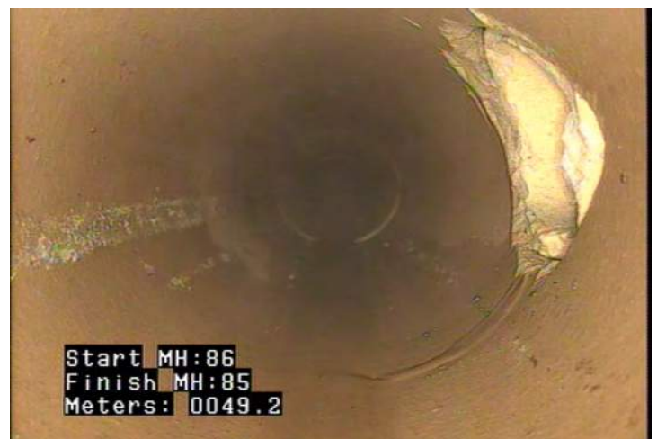
TB - Tap, Break-in / Hammer @ 49.2 m.
