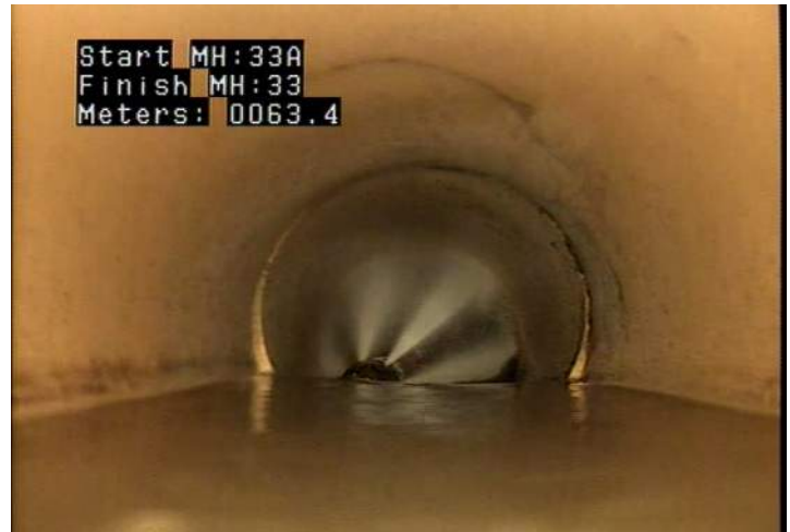
CC - Crack Circumferential @ 63.4 m.
