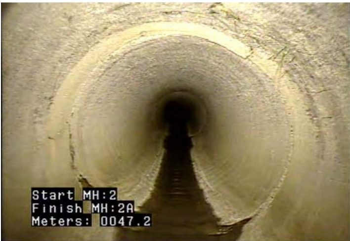
CS - Crack Spiral @ 47.3 m.
