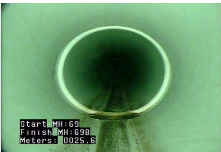
JSM - Joint Separated (open): Medium @ 25.6 m.
