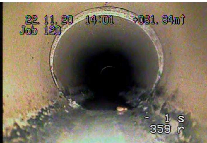
RMJ - Roots, Medium, Joint @ 60.4 m.
