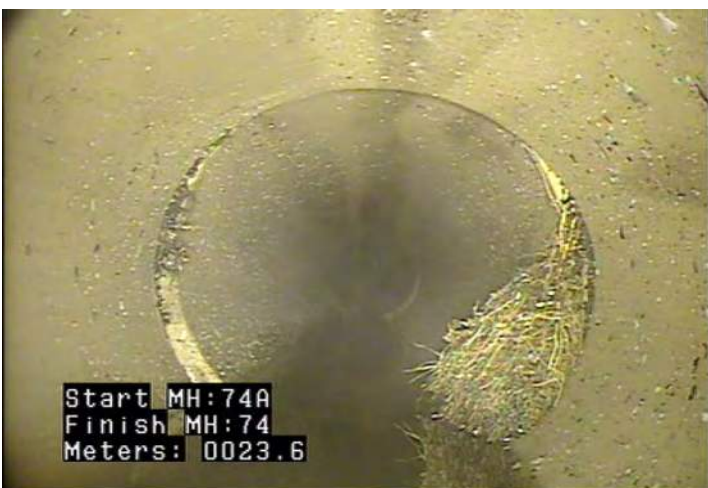
RMJ - Roots, Medium, Joint @ 23.6 m. Moderate roots at most joints
