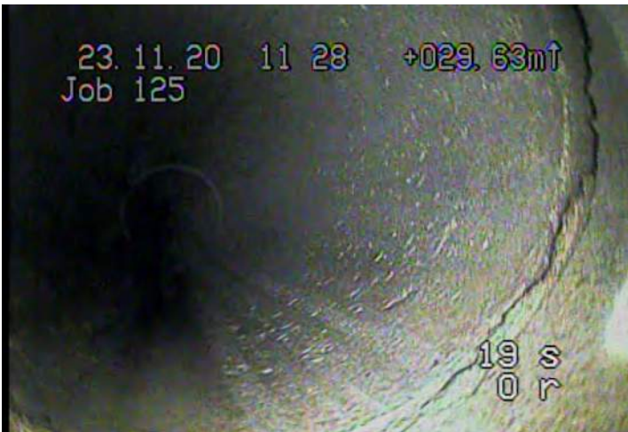
MGO - General Observation @ 29.6 m. Chipped joint
