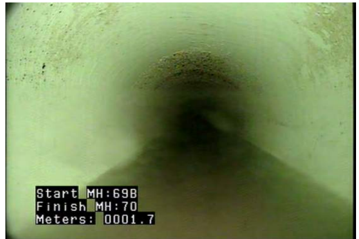
MWLS - Water Level: Sag @ 0.0 m.
