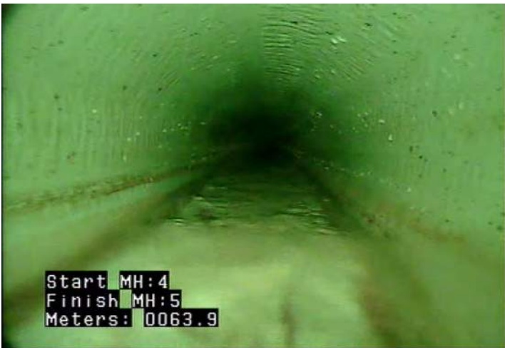
MWLS - Water Level: Sag @ 63.9 m.
