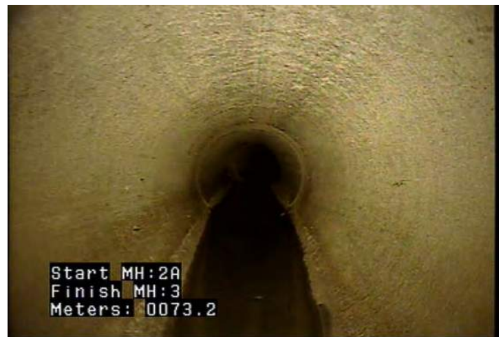
MWL - Water Level @ 73.2 m. Debris in manhole holding back water
