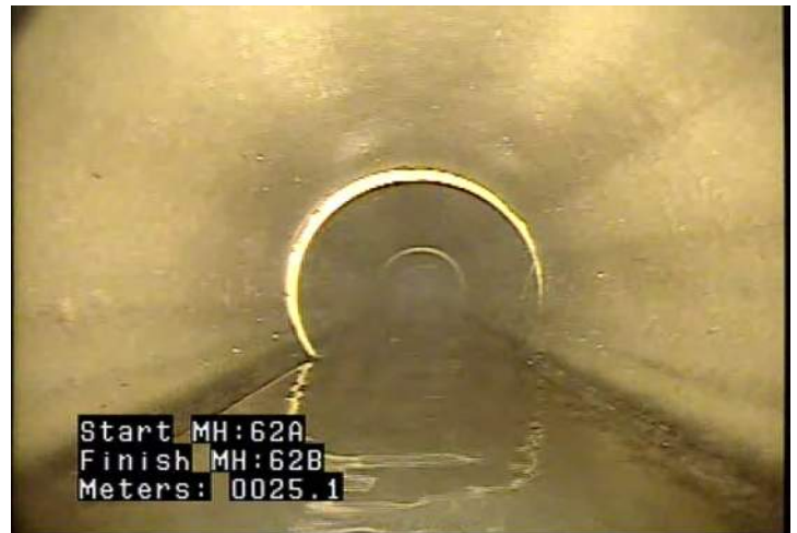
MWLS - Water Level: Sag @ 25.1 m.
