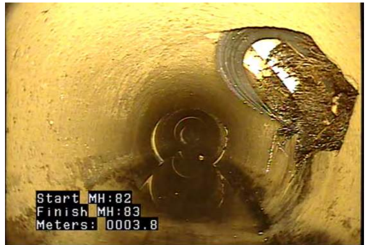
ISSRL - Intruding Seal Material - Sealing Ring: Loose/Poorly Fitting @ 3.8 m.
