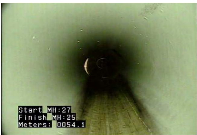
MWM - Water Mark @ 54.1 m. Pipe is 90% stained black from holding material from this point to MH.
