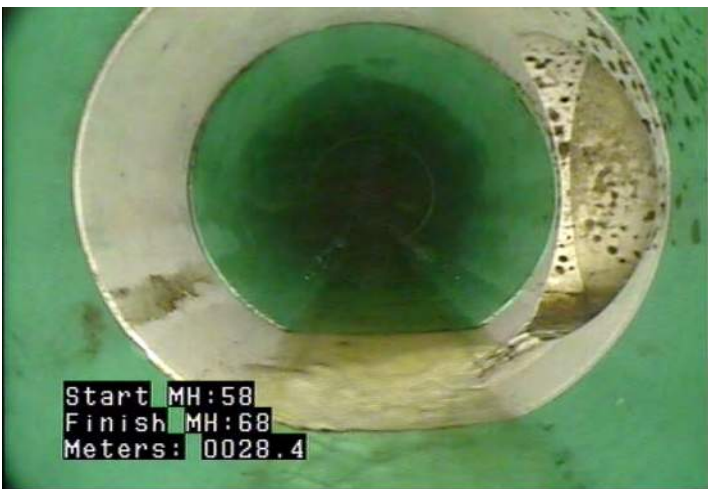
TFA - Tap, Factory Made: Active @ 28.4 m.
