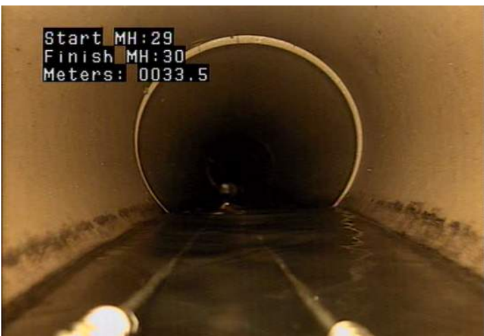
MWLS - Water Level: Sag @ 33.6 m.
