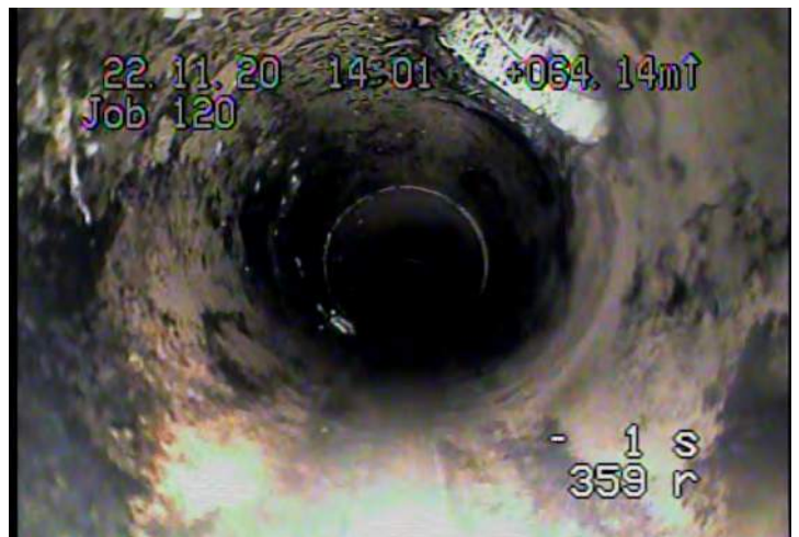
TB - Tap, Break-in / Hammer @ 64.1 m.
