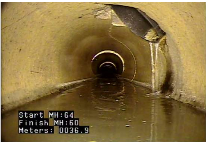
TBA - Tap, Break-in / Hammer: Active @ 36.9 m.
