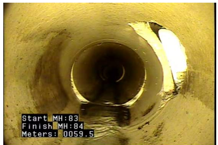
TBA - Tap, Break-in / Hammer: Active @ 59.5 m.
