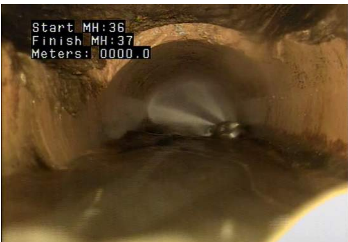
MGO - General Observation @ 0.0 m. Flusher on to reduce flow.
