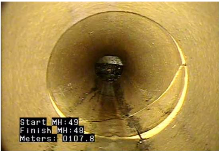
FM - Fracture Multiple @ 107.8 m.
