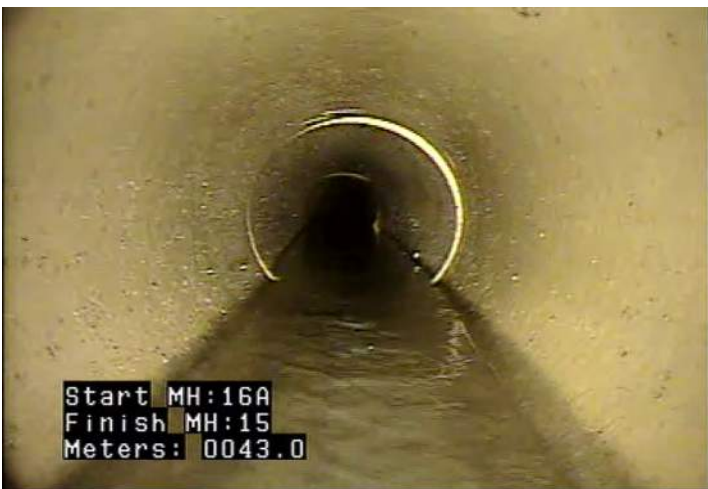
MWLS - Water Level: Sag @ 43.0 m.
