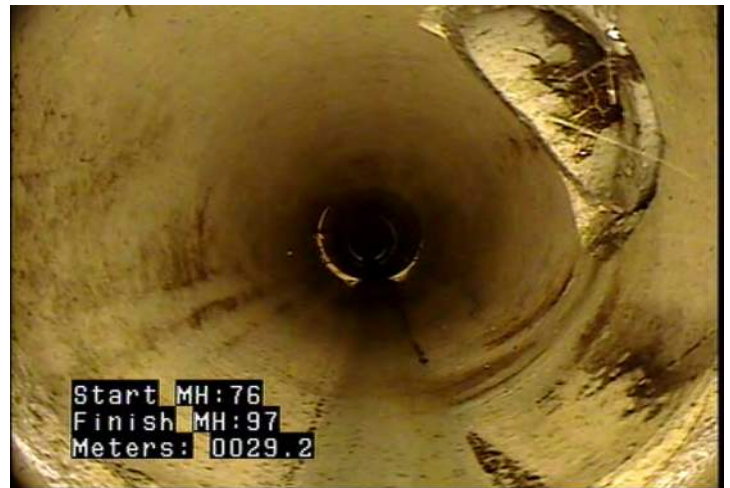
TBD - Tap, Break-in / Hammer: Defective @ 29.2 m. Roots in service
