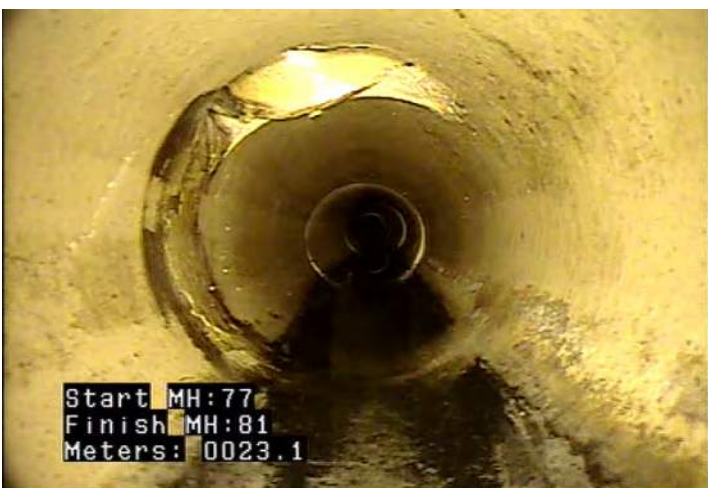
TB - Tap, Break-in / Hammer @ 23.1 m.
