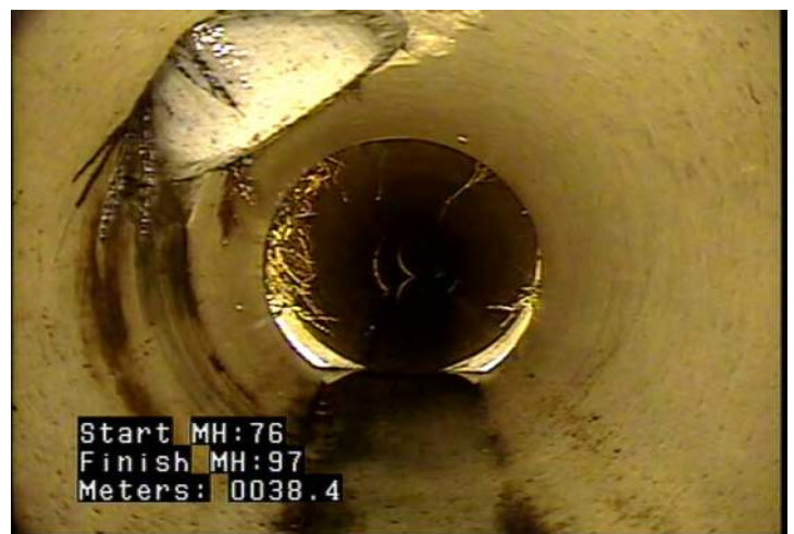
TB - Tap, Break-in / Hammer @ 38.4 m.
