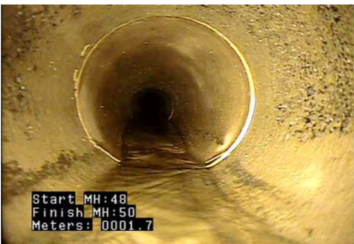
FS - Fracture Spiral @ 1.7 m.
