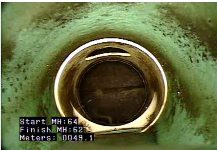
TF - Tap, Factory Made @ 49.1 m. Drop Structure
