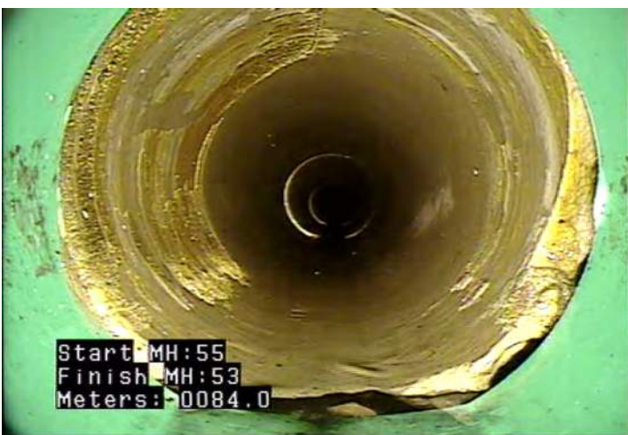
MMC - Material Change @ 84.0 m. PVC to Clay tile
