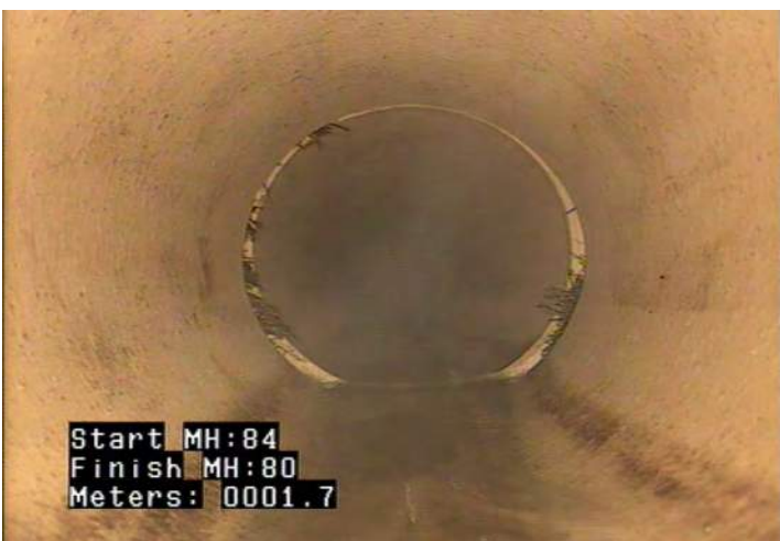
RFJ - Roots, Fine: Joint @ 1.0 m. Fine roots at most joints
