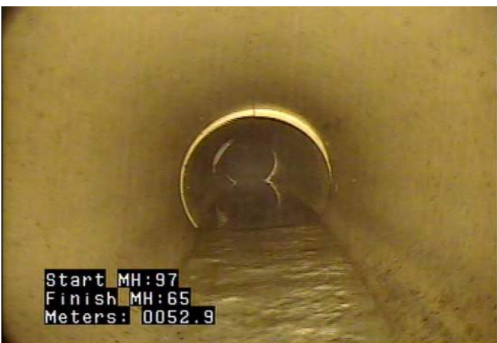
MWLS - Water Level: Sag @ 52.9 m.
