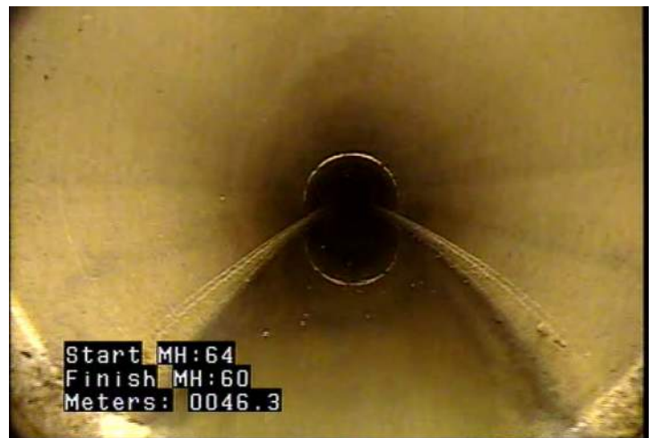
MWLS - Water Level: Sag @ 46.3 m.
