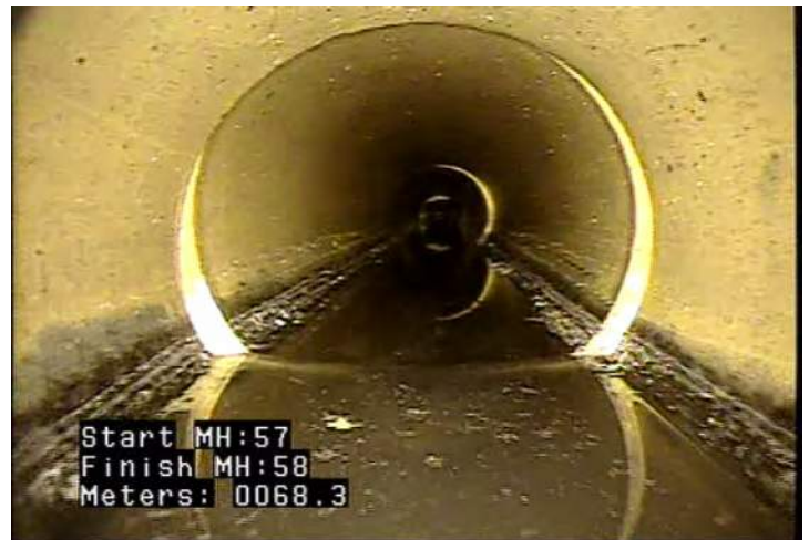
JOM - Joint Offset (displaced): Medium @ 68.3 m.
