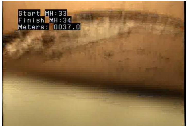
DAE - Deposits Attached: Encrustation @ 37.0 m.
