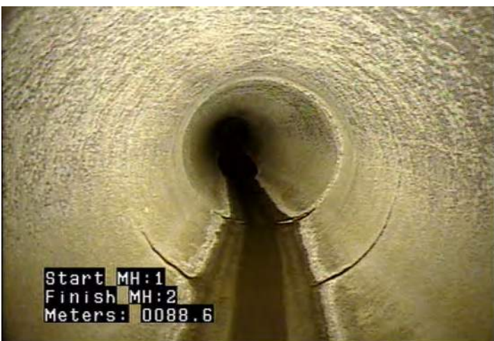
CC - Crack Circumferential @ 88.6 m.
