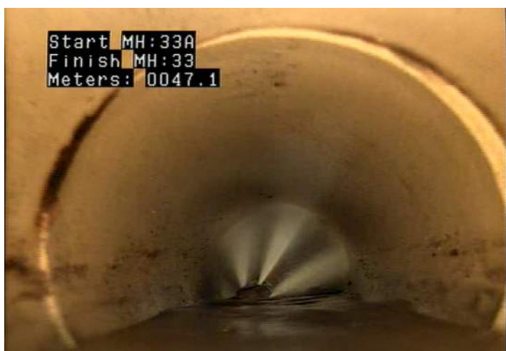
DAE - Deposits Attached: Encrustation @ 47.1 m.
