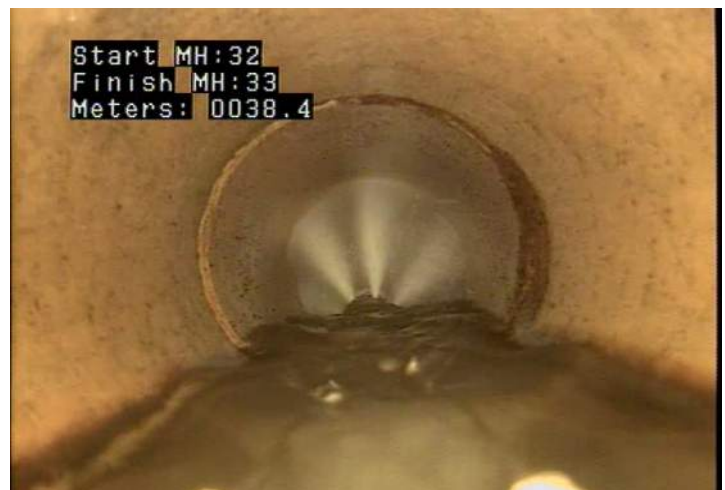
DAE - Deposits Attached: Encrustation @ 38.4 m.
