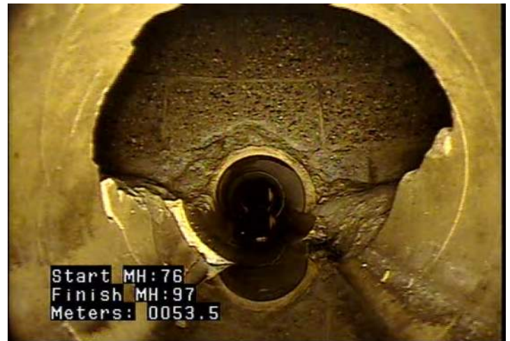
CC - Crack Circumferential @ 53.5 m.
