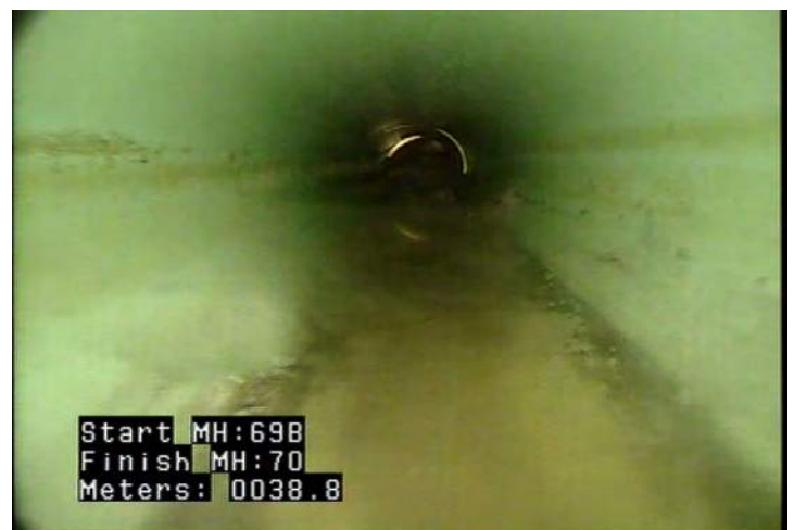
MWLS - Water Level: Sag @ 38.8 m.
