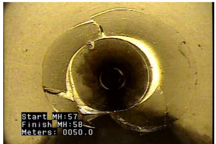
TB - Tap, Break-in / Hammer @ 51.9 m.
