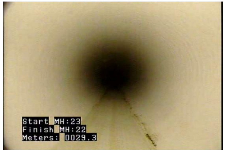
MWLS - Water Level: Sag @ 29.3 m.
