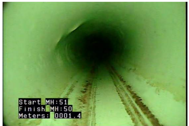
MWLS - Water Level: Sag @ 54.9 m.
