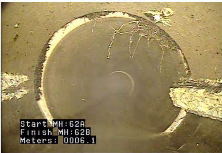
DAGS - Deposits Attached: Grease @ 6.1 m.
