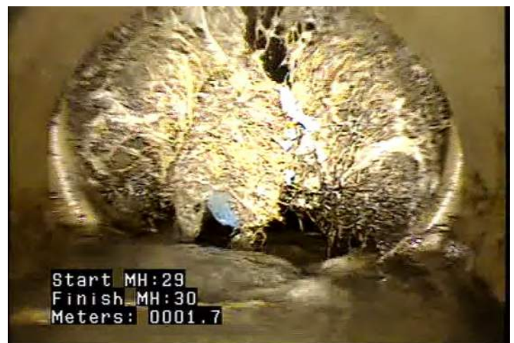
RBJ - Roots, Ball, Joint @ 1.7 m.
