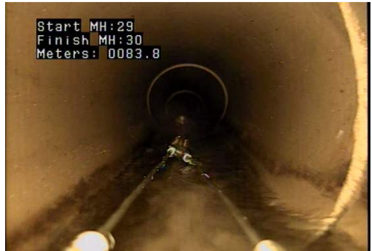
B - Pipe Broken @ 83.8 m.
