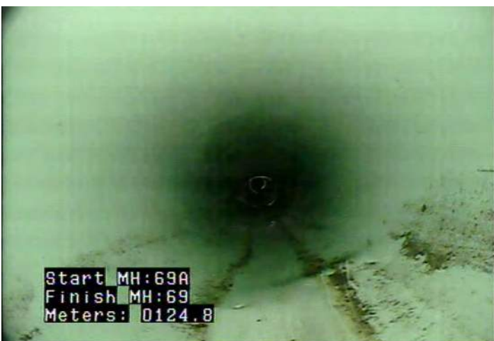
D - Pipe Deformed @ 124.8 m.
