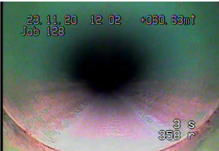
DSGV - Deposits Settled: Gravel @ 59.9 m.
