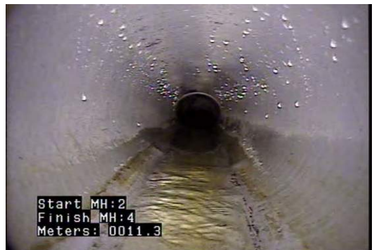
MWLS - Water Level: Sag @ 11.3 m.
