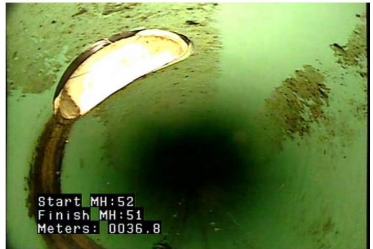
TSD - Tap, Saddle: Defective @ 36.8 m. Gasket visible around service.
