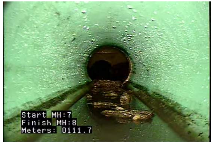
DSGV - Deposits Settled: Gravel @ 111.7 m.
