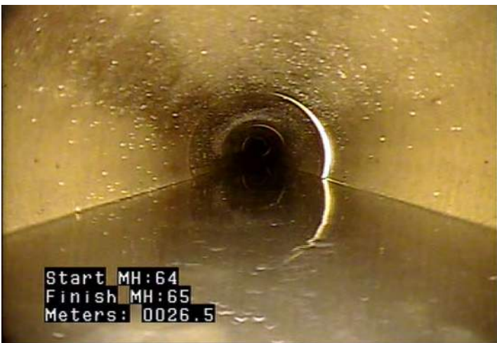
MGP - General Photograph @ 26.5 m. Deepest point of sag
