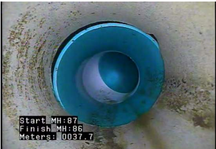
MLC - Lining Change @ 37.7 m. Clay tile to PVC
