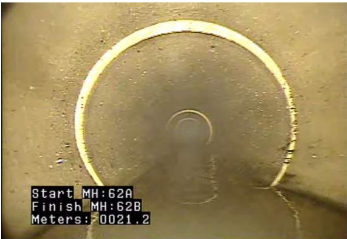
MWLS - Water Level: Sag @ 21.2 m.
