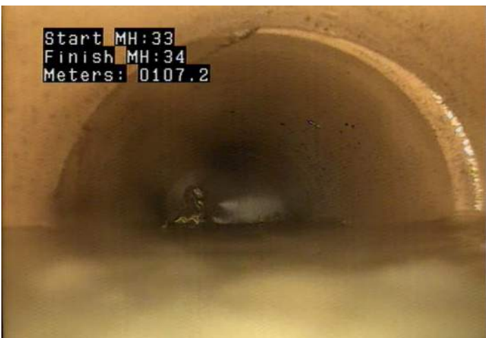
CC - Crack Circumferential @ 107.2 m.
