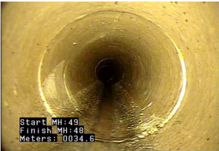
CS - Crack Spiral @ 34.8 m.
