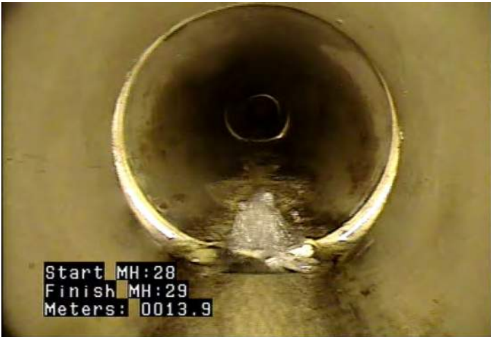
JOM - Joint Offset (displaced): Medium @ 13.9 m.
