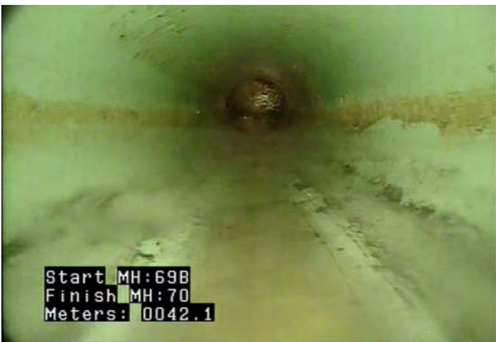
MWLS - Water Level: Sag @ 42.1 m.
