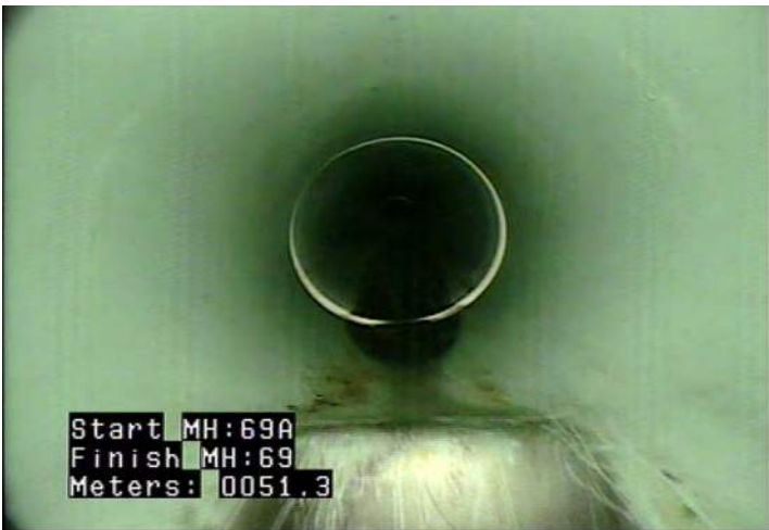
D - Pipe Deformed @ 51.3 m.
