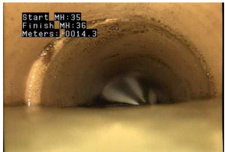
DAE - Deposits Attached: Encrustation @ 14.3 m.
