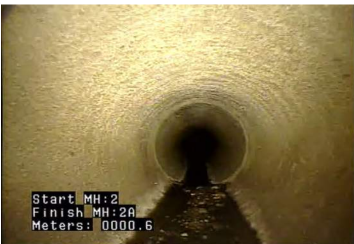
DSGV - Deposits Settled: Gravel @ 0.6 m.
