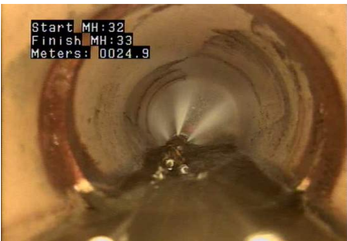
DAE - Deposits Attached: Encrustation @ 24.9 m.
