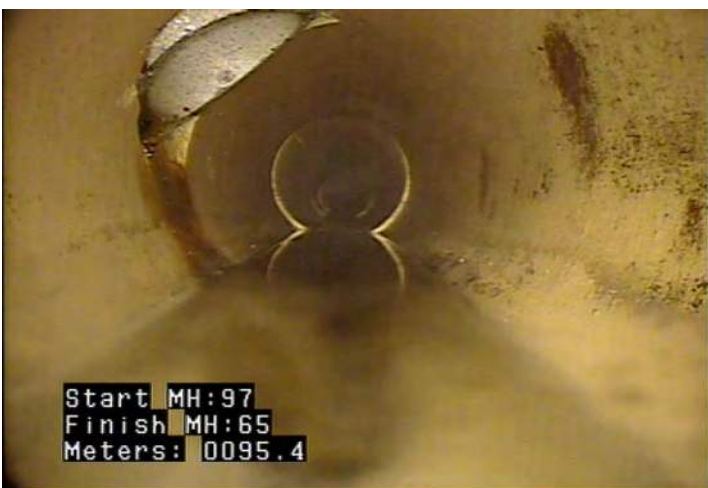
TB - Tap, Break-in / Hammer @ 95.4 m.
