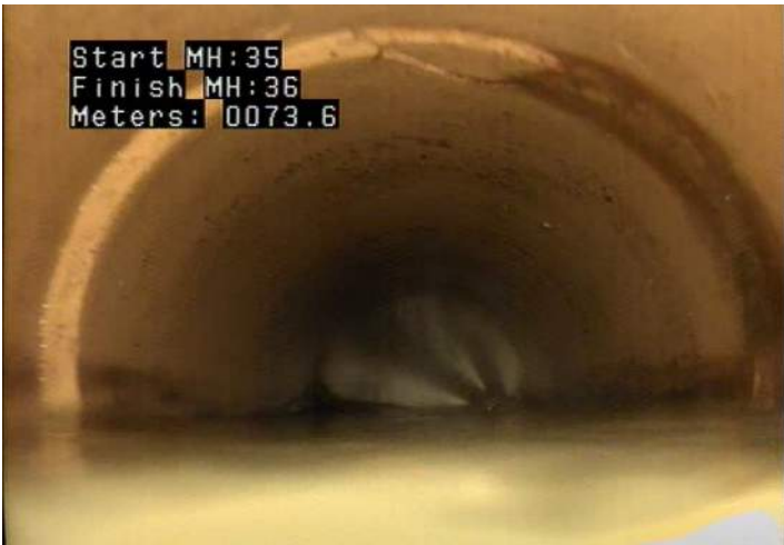
DAE - Deposits Attached: Encrustation @ 73.6 m.
