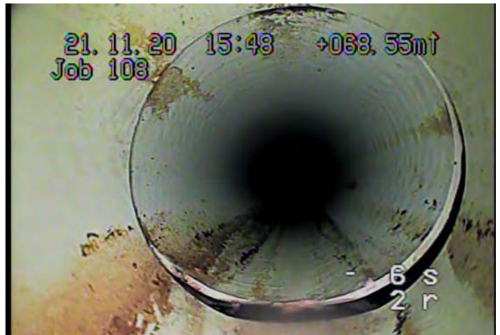
JOM - Joint Offset (displaced): Medium @ 68.4 m.
