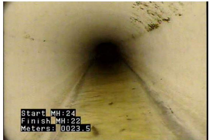
MWLS - Water Level: Sag @ 23.5 m.
