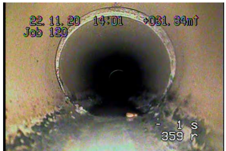
FS - Fracture Spiral @ 60.4 m.
