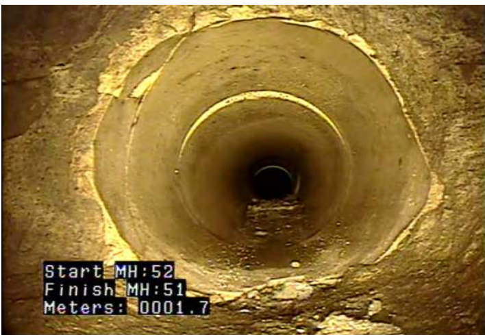
CC - Crack Circumferential @ 0.5 m. At MH opening
