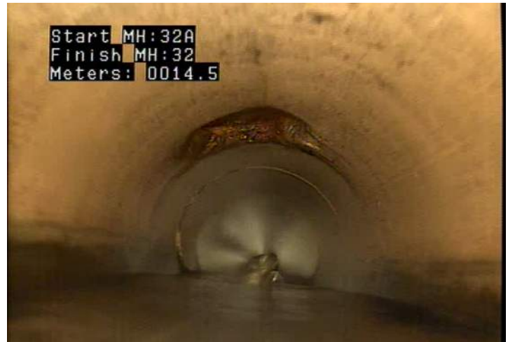
H - Hole in Pipe @ 14.5 m.
