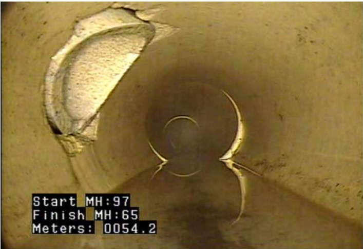
TB - Tap, Break-in / Hammer @ 54.2 m.
