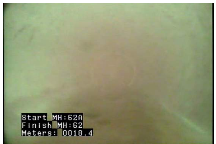
MWLS - Water Level: Sag @ 18.4 m.
