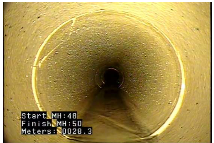
FM - Fracture Multiple @ 29.7 m.
