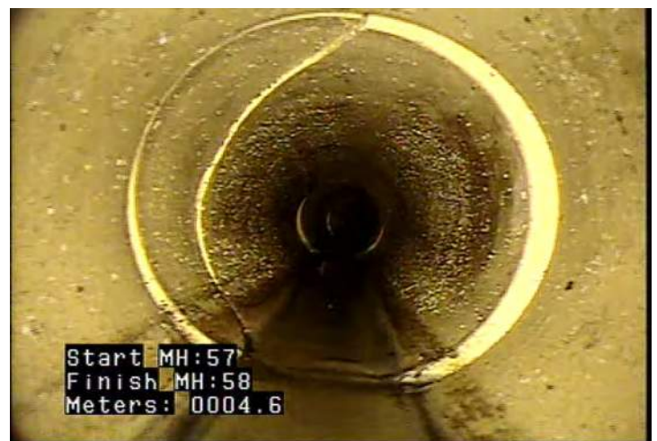
FS - Fracture Spiral @ 4.6 m.
