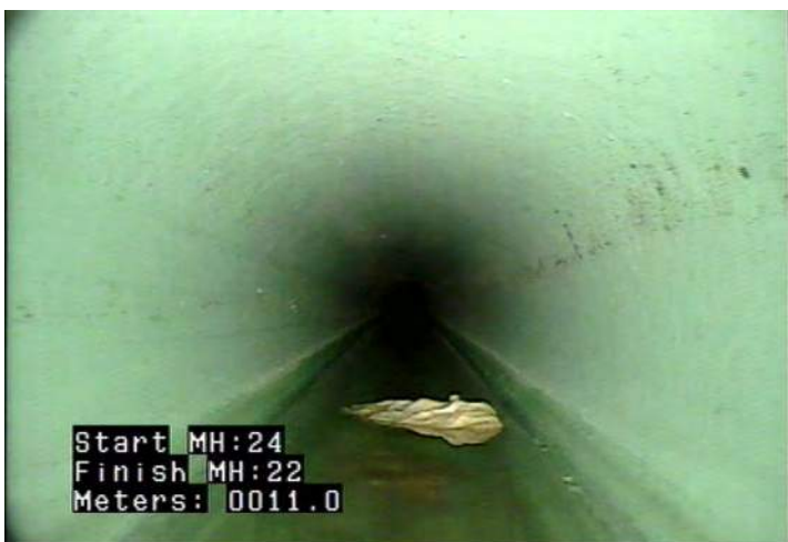
MWLS - Water Level: Sag @ 11.0 m.
