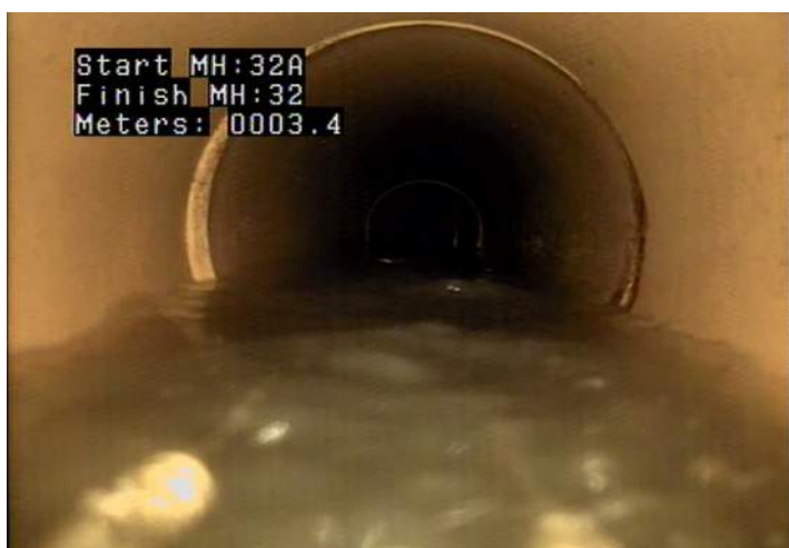
DAE - Deposits Attached: Encrustation @ 3.4 m.
