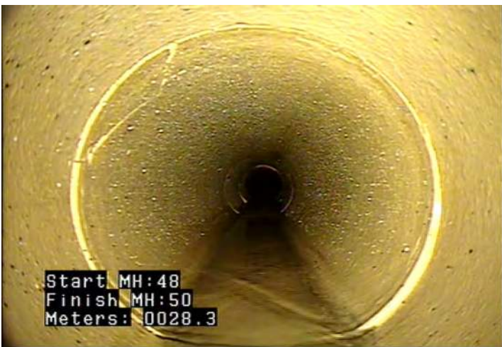
FS - Fracture Spiral @ 28.3 m.
