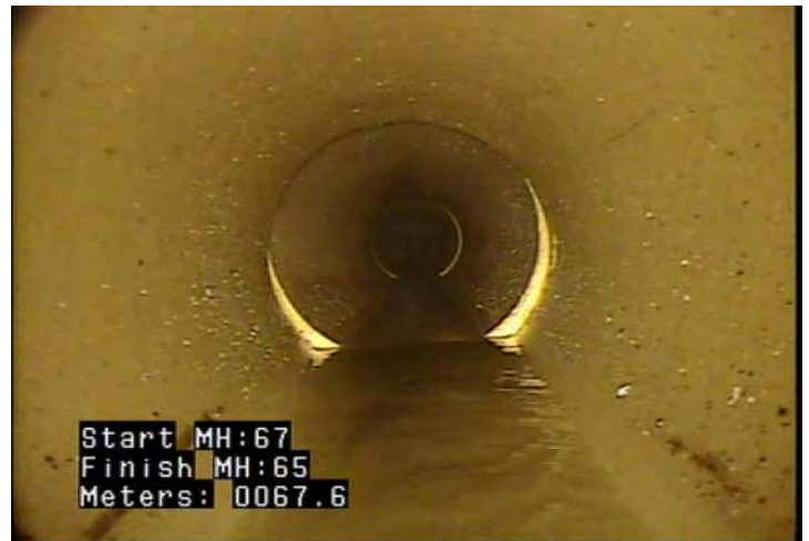
MWLS - Water Level: Sag @ 67.6 m.
