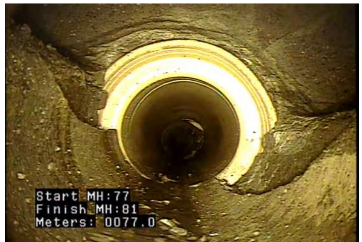
AMH - Access Point - Manhole @ 77.0 m. S MH 81
