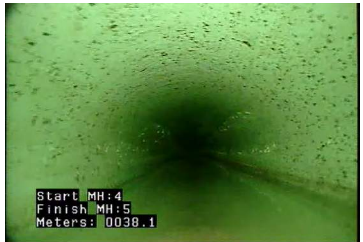
MWLS - Water Level: Sag @ 38.1 m.
