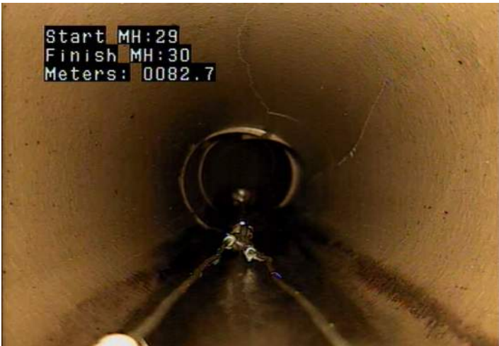
B - Pipe Broken @ 82.7 m.
