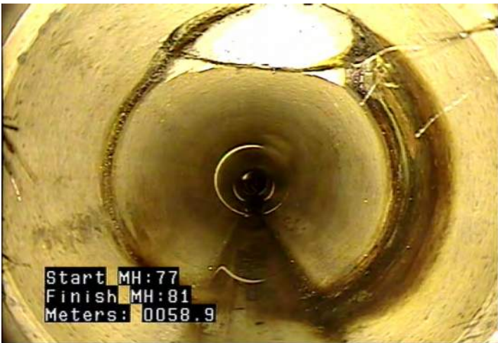
TB - Tap, Break-in / Hammer @ 58.9 m.
