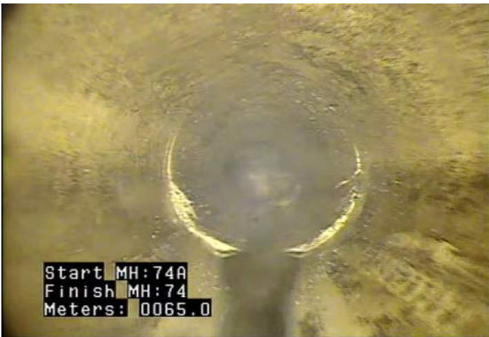
RMJ - Roots, Medium, Joint @ 65.0 m.
