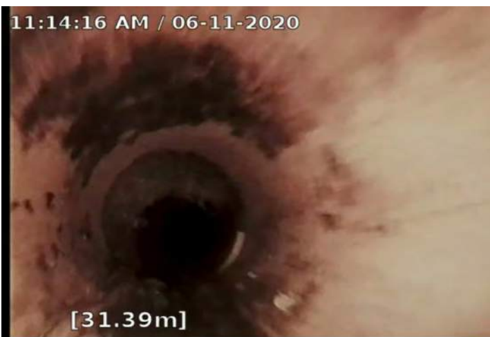
RMJ - Roots, Medium, Joint @ 31.3 m.
