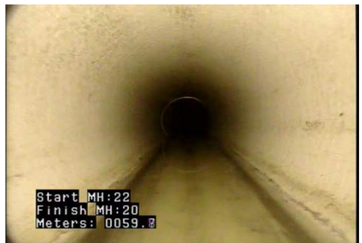
MWLS - Water Level: Sag @ 59.7 m.
