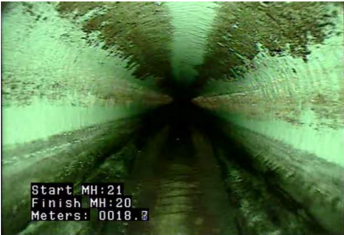
MWLS - Water Level: Sag @ 18.7 m.
