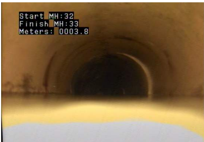
CM - Crack Multiple @ 3.8 m.
