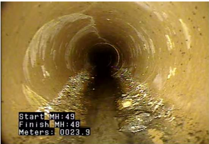
CS - Crack Spiral @ 23.9 m.
