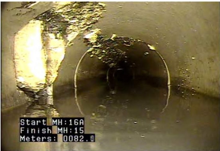
DAGS - Deposits Attached: Grease @ 82.0 m.
