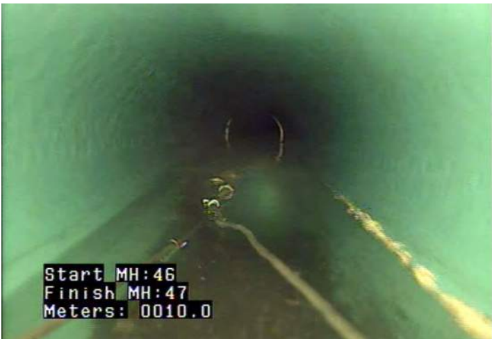
MWLS - Water Level: Sag @ 10.0 m.
