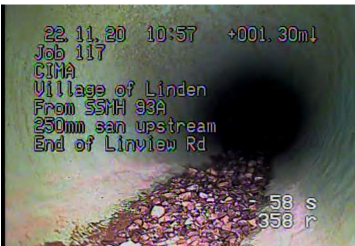
DSGV - Deposits Settled: Gravel @ 0.0 m.
