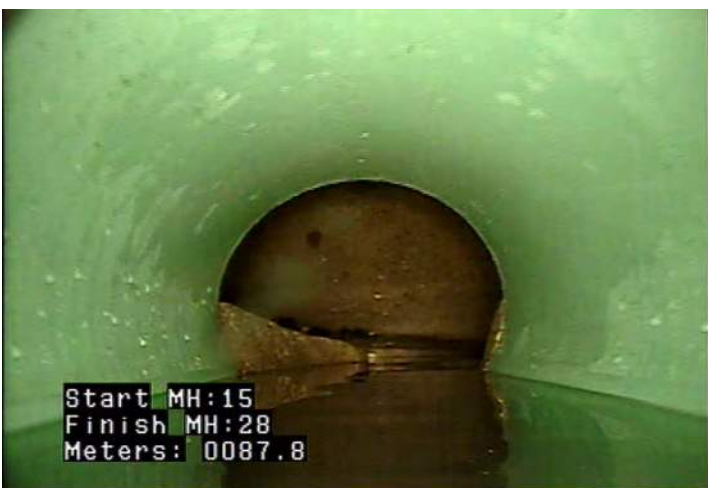
MWLS - Water Level: Sag @ 87.8 m.
