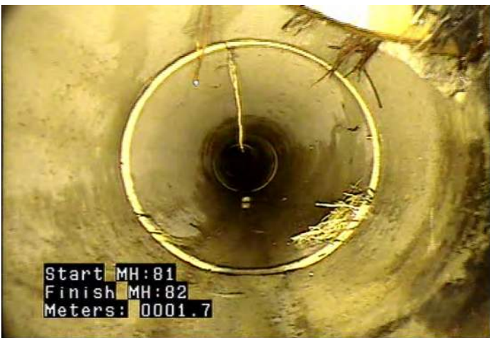
RFJ - Roots, Fine: Joint @ 1.8 m. Fine roots at most joints throughout pipe
