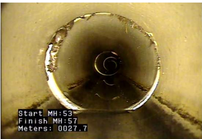
RTJ - Roots, Tap: Joint @ 27.7 m.
