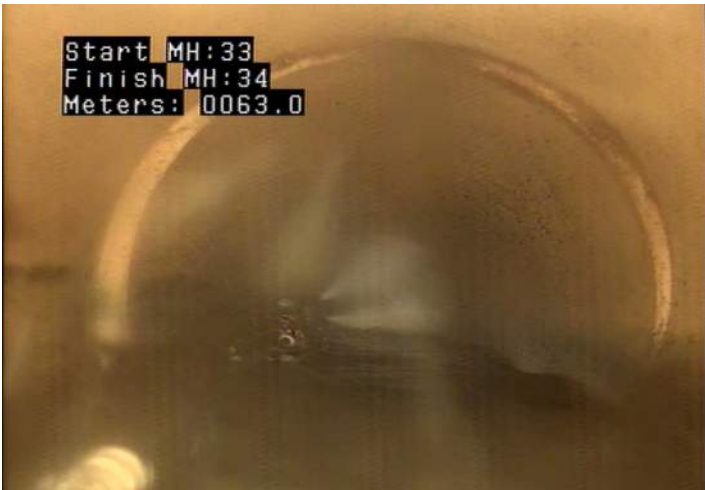
DAE - Deposits Attached: Encrustation @ 63.0 m.
