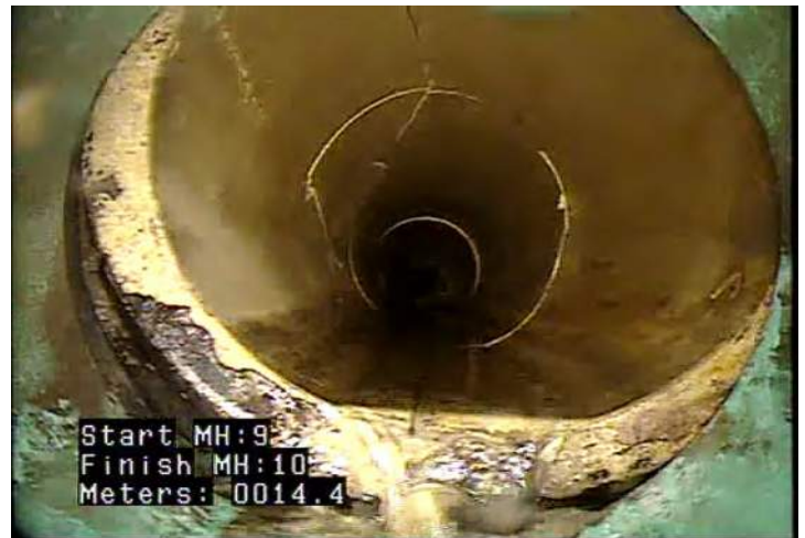
JOL - Joint Offset (displaced): Large @ 14.4 m.
