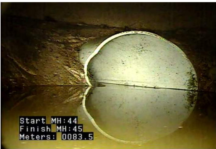
AMH - Access Point - Manhole @ 83.5 m. S MH 45
