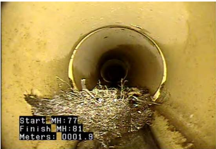
RMJ - Roots, Medium, Joint @ 1.8 m.
