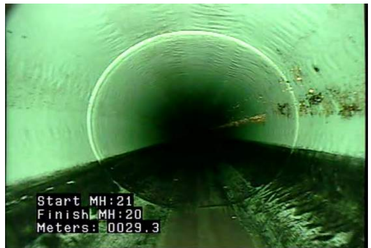
MWLS - Water Level: Sag @ 29.3 m.
