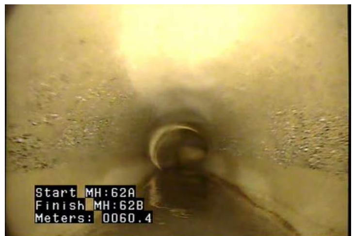
JOM - Joint Offset (displaced): Medium @ 61.4 m.
