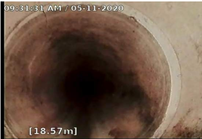
FS - Fracture Spiral @ 18.6 m.
