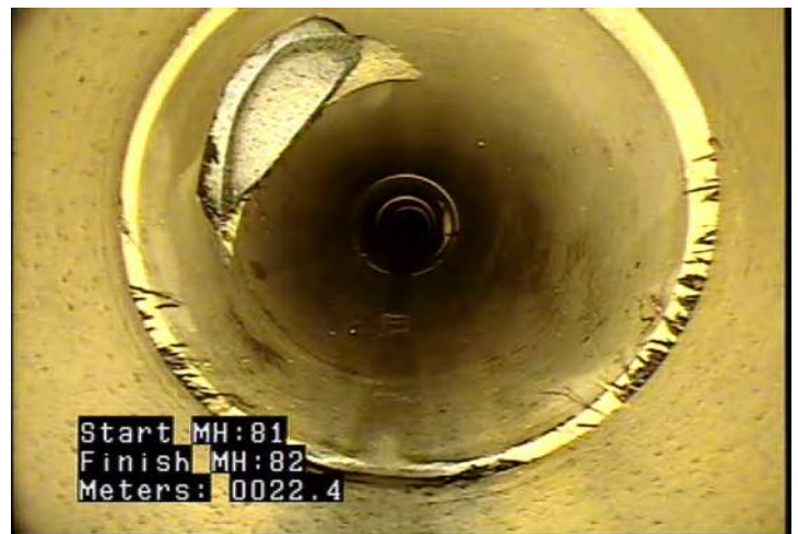
TB - Tap, Break-in / Hammer @ 22.4 m.
