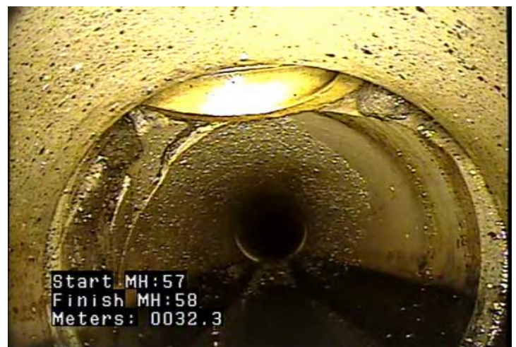
TB - Tap, Break-in / Hammer @ 32.3 m.
