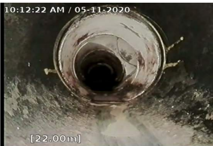
MGO - General Observation @ 22.0 m. Backflow Preventer
