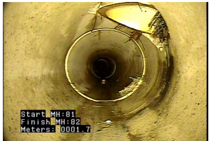
TB - Tap, Break-in / Hammer @ 1.7 m.
