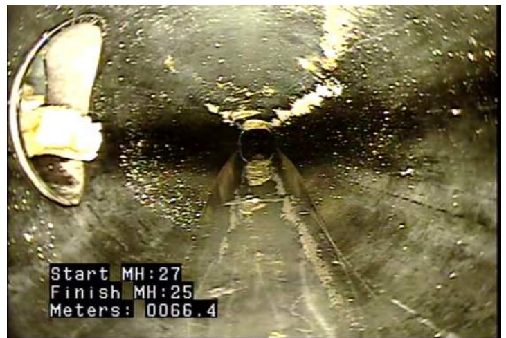
MWLS - Water Level: Sag @ 66.7 m.
