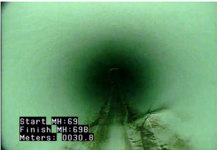
D - Pipe Deformed @ 30.8 m.
