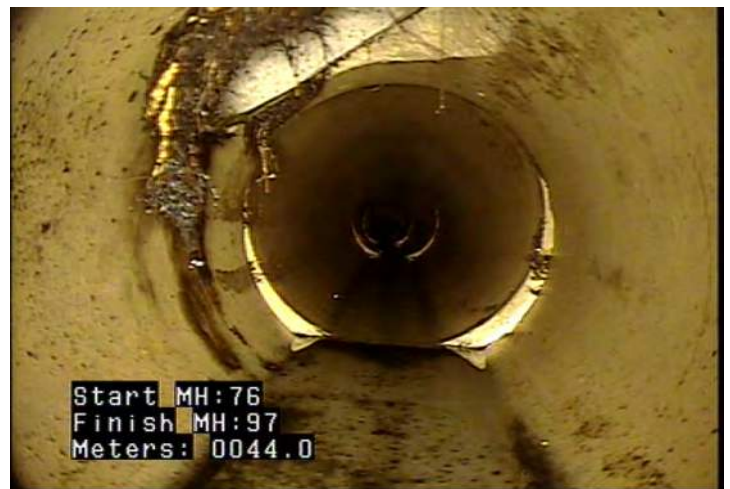
TBD - Tap, Break-in / Hammer: Defective @ 44.0 m. Roots around service
