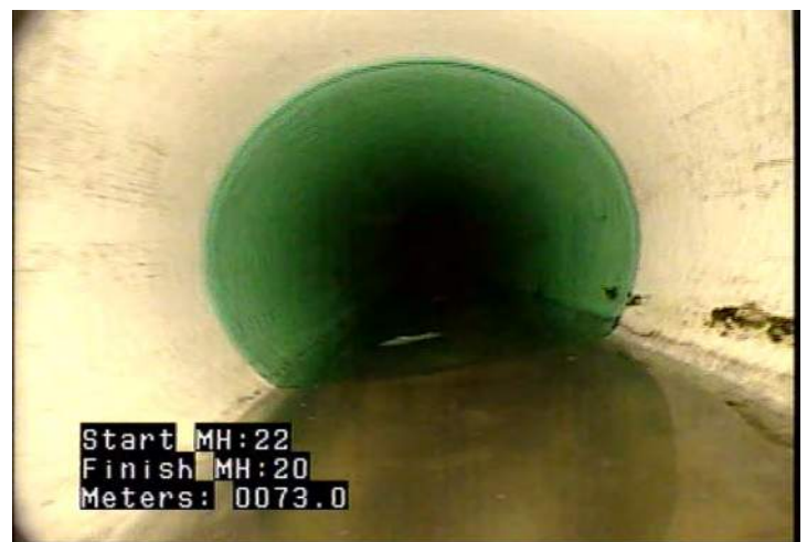
MMC - Material Change @ 73.0 m. White to Blue PVC
