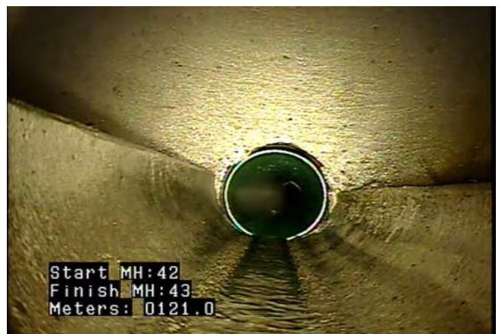
AMH - Access Point - Manhole @ 121.0 m. S MH 43
