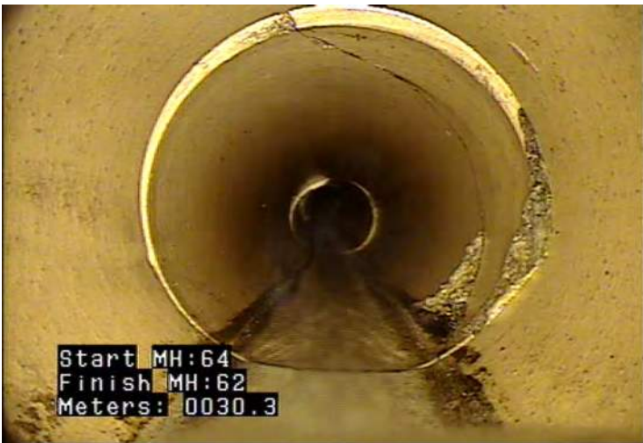
DAE - Deposits Attached: Encrustation @ 30.3 m.
