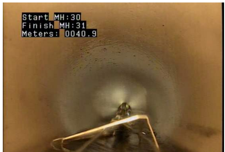
MWLS - Water Level: Sag @ 40.9 m.
