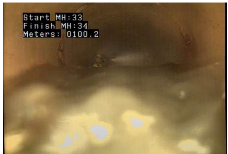
DAE - Deposits Attached: Encrustation @ 100.2 m.
