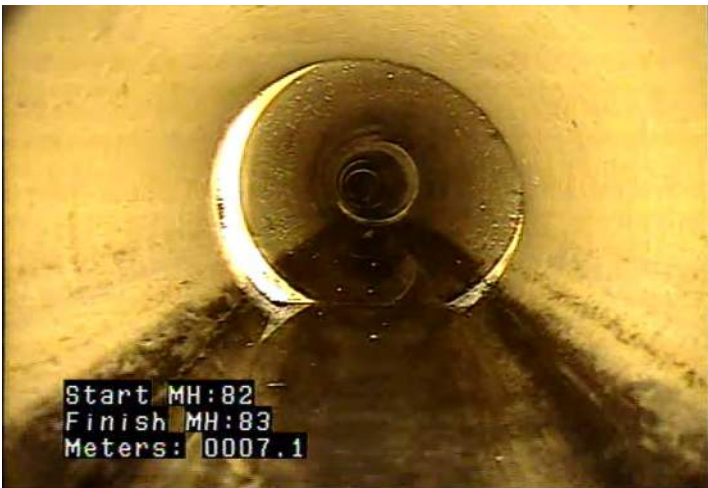
RFJ - Roots, Fine: Joint @ 7.1 m. Fine roots at most joints
