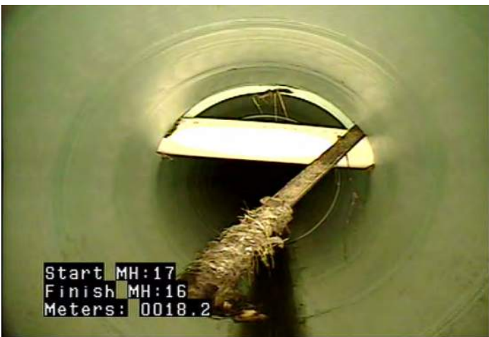
OBP - Obstacle - External Pipe or Cable in Sewer @ 18.2 m.
