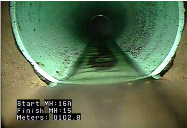
MMC - Material Change @ 102.8 m. Clay tile to PVC
