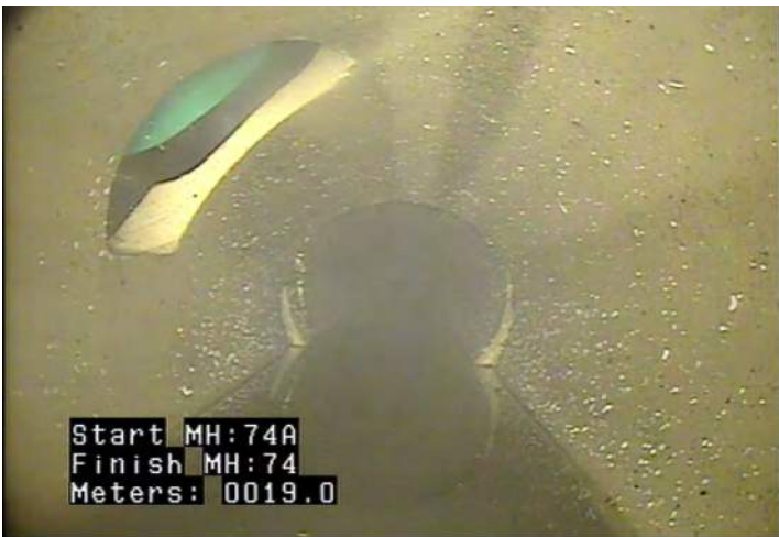
TB - Tap, Break-in / Hammer @ 19.0 m.
