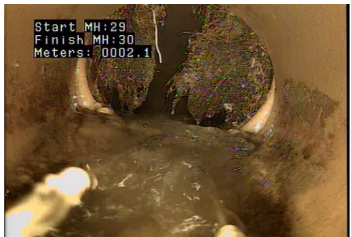
RBJ - Roots, Ball, Joint @ 2.1 m.
