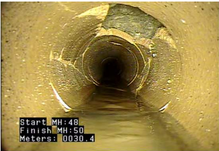
HVV - Hole in Pipe: Void Visible @ 30.6 m.
