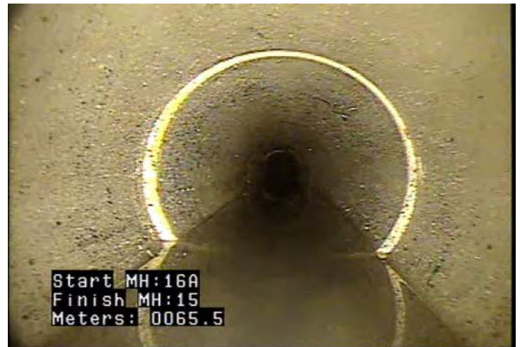
MWLS - Water Level: Sag @ 65.5 m.
