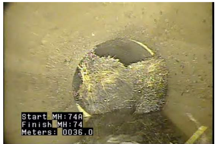
RBJ - Roots, Ball, Joint @ 36.0 m.
