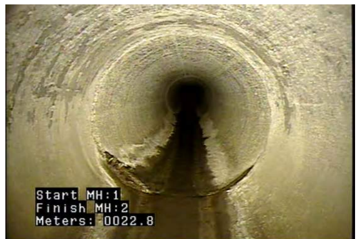
OBJ - Obstacle - Object Wedged in Joint @ 22.8 m. Branch
