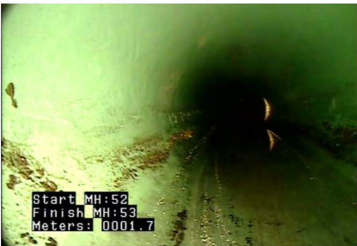
MWLS - Water Level: Sag @ 1.7 m.
