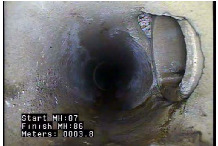
TB - Tap, Break-in / Hammer @ 3.8 m.
