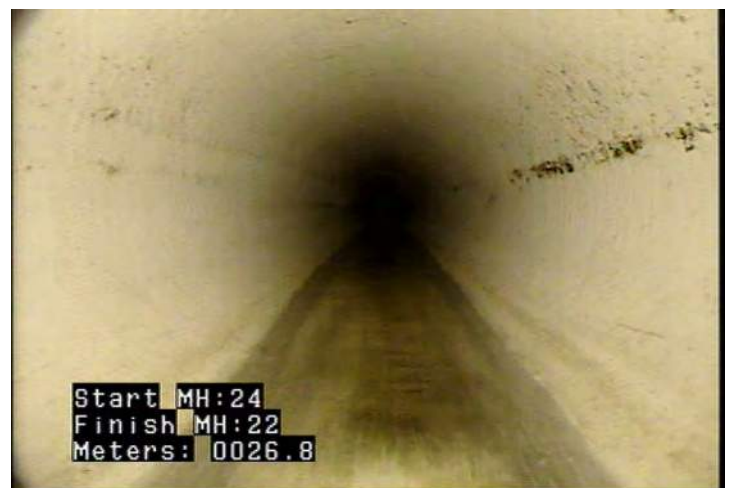
MWLS - Water Level: Sag @ 26.8 m.
