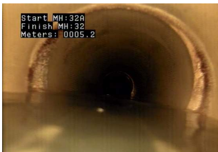
DAE - Deposits Attached: Encrustation @ 5.2 m.
