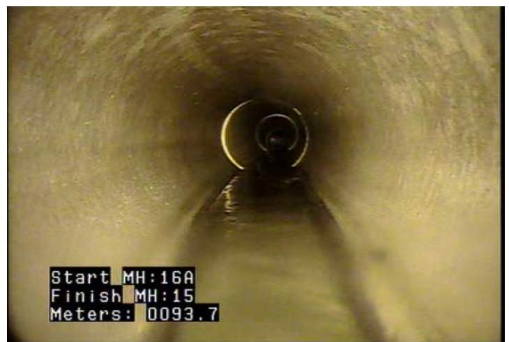
MWLS - Water Level: Sag @ 93.7 m.
