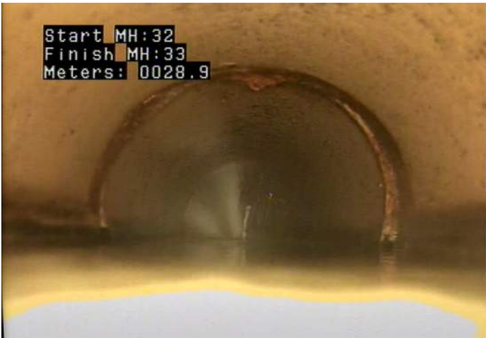
DAE - Deposits Attached: Encrustation @ 28.9 m.
