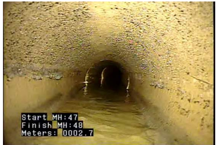
MWLS - Water Level: Sag @ 2.7 m.
