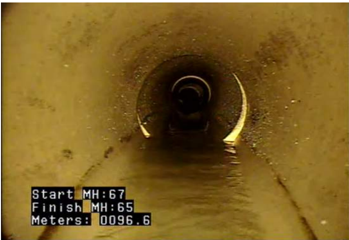
MWLS - Water Level: Sag @ 95.9 m.
