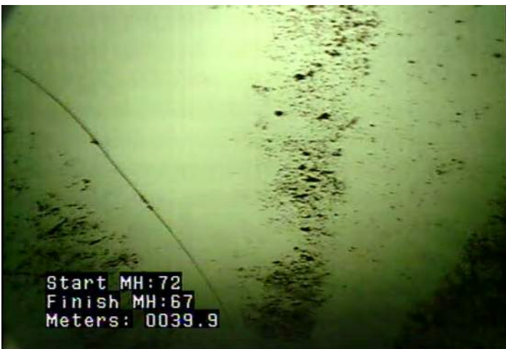
MGP - General Photograph @ 39.9 m. Closer view of crack
