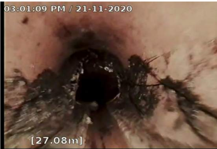
RMJ - Roots, Medium, Joint @ 27.5 m.
