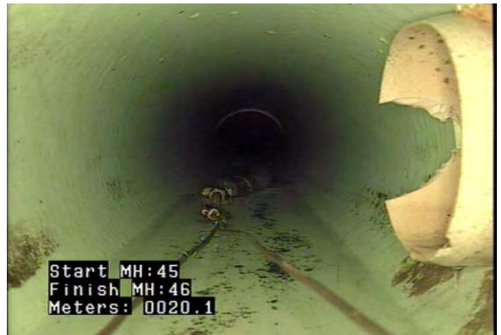
TSI - Tap, Saddle: Intruding @ 20.1 m. Connecting pipe broken
