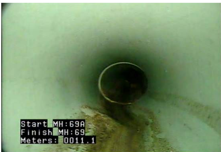
D - Pipe Deformed @ 11.1 m.
