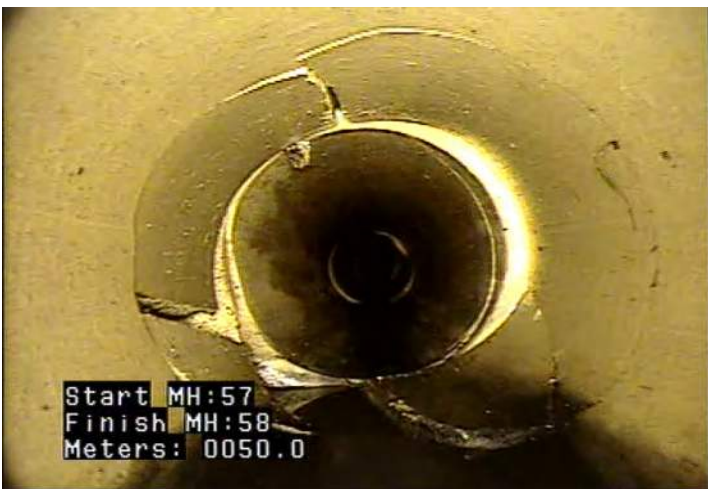
B - Pipe Broken @ 50.0 m.
