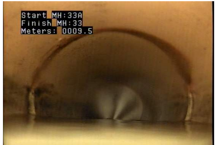
DAE - Deposits Attached: Encrustation @ 9.5 m.
