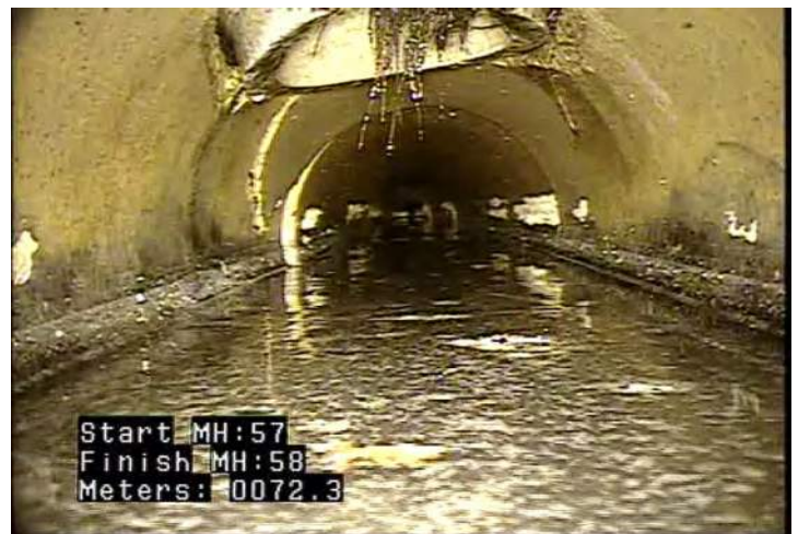
TBD - Tap, Break-in / Hammer: Defective @ 72.3 m. Roots in service
