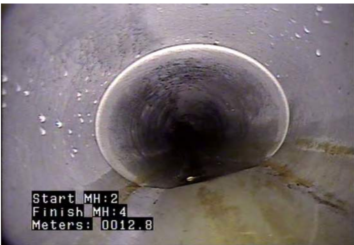
D - Pipe Deformed @ 12.8 m. Pipe ovalled (possible offset joint)
