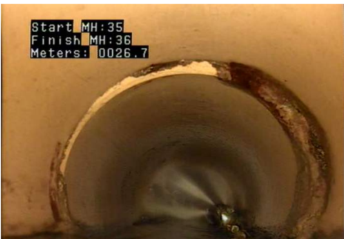
DAE - Deposits Attached: Encrustation @ 26.7 m.
