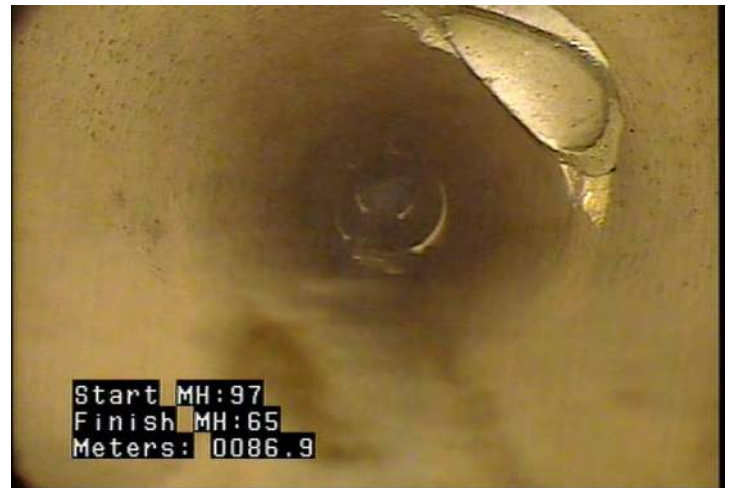
TB - Tap, Break-in / Hammer @ 86.9 m.
