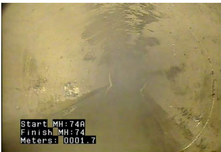
CC - Crack Circumferential @ 1.0 m.
