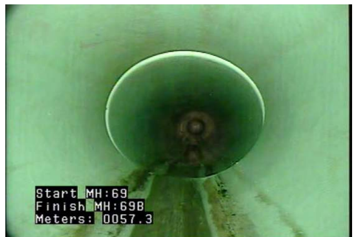
JAM - Joint Angular: Medium @ 57.3 m.
