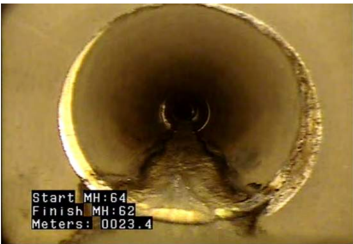
DAE - Deposits Attached: Encrustation @ 23.4 m.
