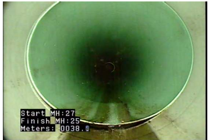
D - Pipe Deformed @ 38.0 m.
