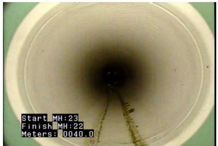
MMC - Material Change @ 40.0 m. Blue to White PVC
