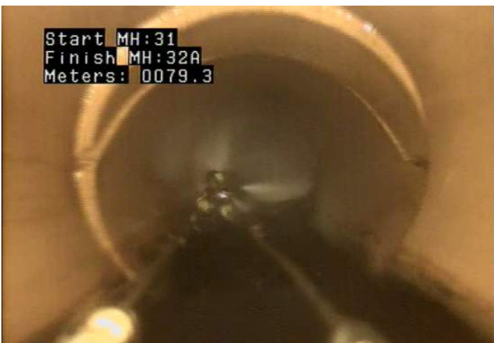
FC - Fracture Circumferential @ 79.3 m.
