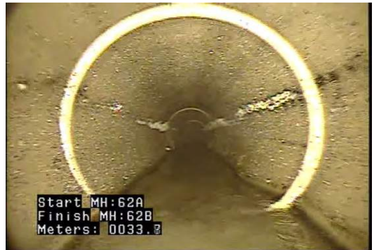
DAGS - Deposits Attached: Grease @ 33.8 m.
