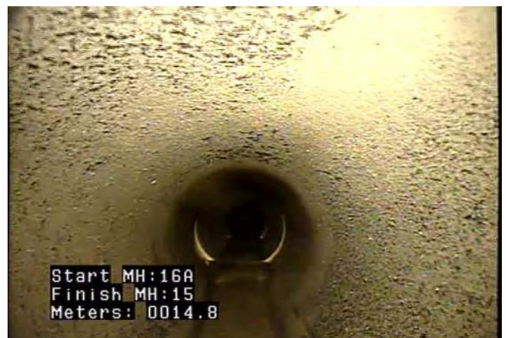
MWLS - Water Level: Sag @ 14.8 m.
