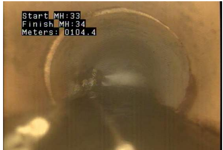
DAE - Deposits Attached: Encrustation @ 104.4 m.
