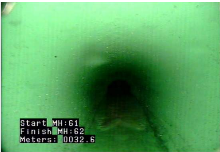
MWLS - Water Level: Sag @ 32.6 m.
