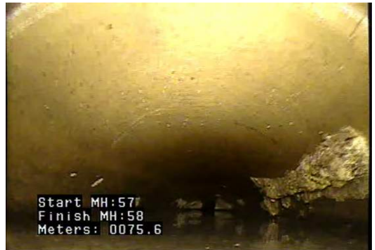
DAGS - Deposits Attached: Grease @ 75.6 m.
