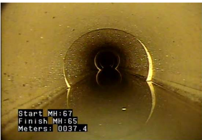
MGP - General Photograph @ 37.4 m. Deepest point of sag 30%
