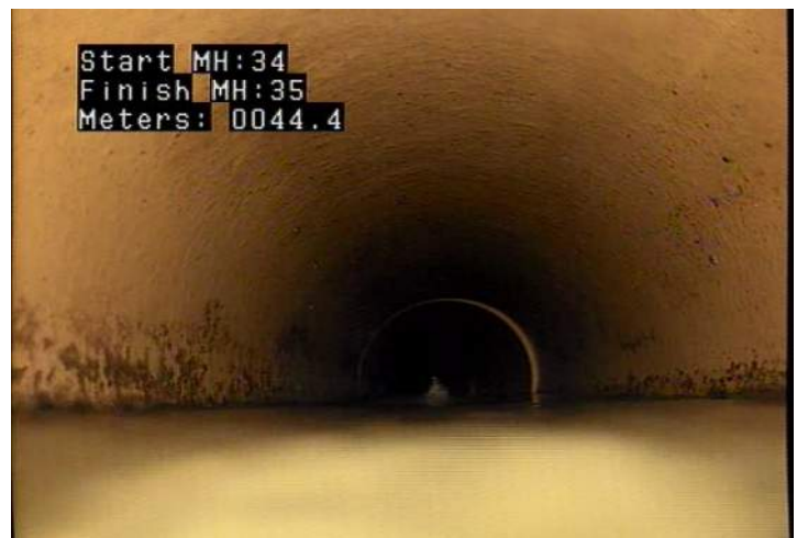
MGO - General Observation @ 44.4 m. Flusher on to reduce flow.
