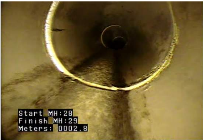
DAE - Deposits Attached: Encrustation @ 2.8 m.
