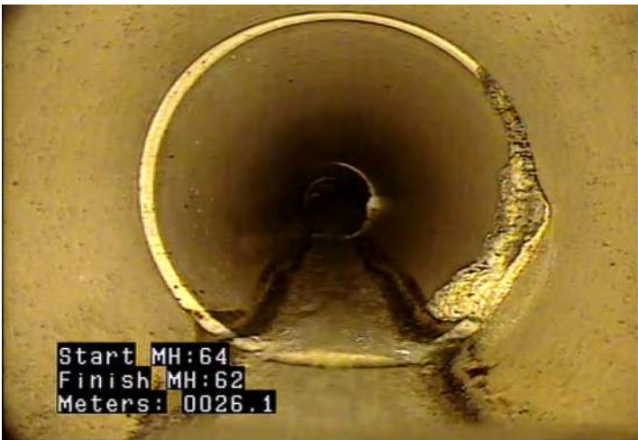
DAE - Deposits Attached: Encrustation @ 26.1 m.
