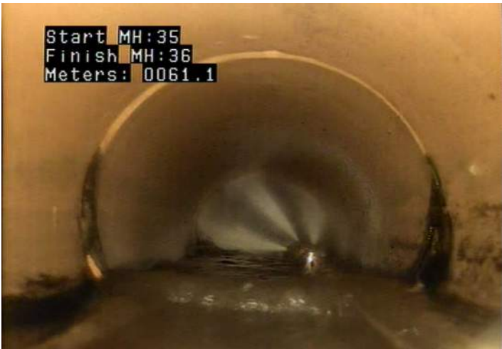
DAE - Deposits Attached: Encrustation @ 61.1 m.
