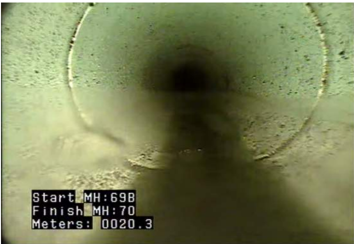
MWLS - Water Level: Sag @ 20.3 m.
