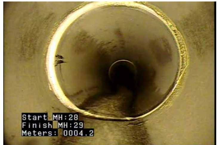
DAE - Deposits Attached: Encrustation @ 4.2 m.
