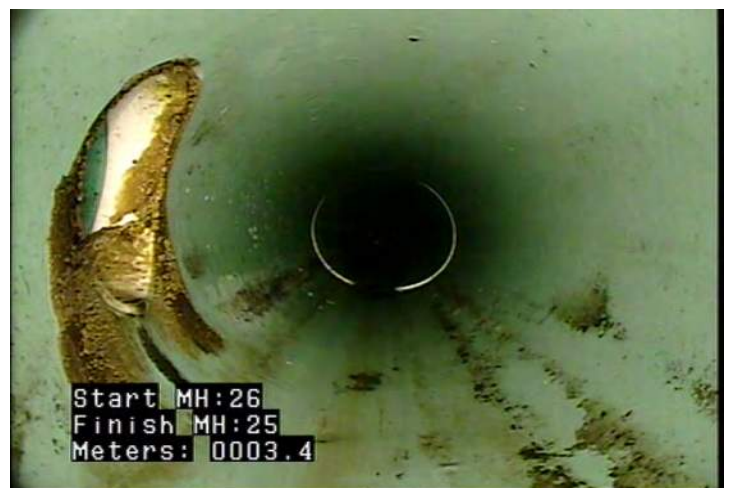
DAE - Deposits Attached: Encrustation @ 3.4 m. Around service.
