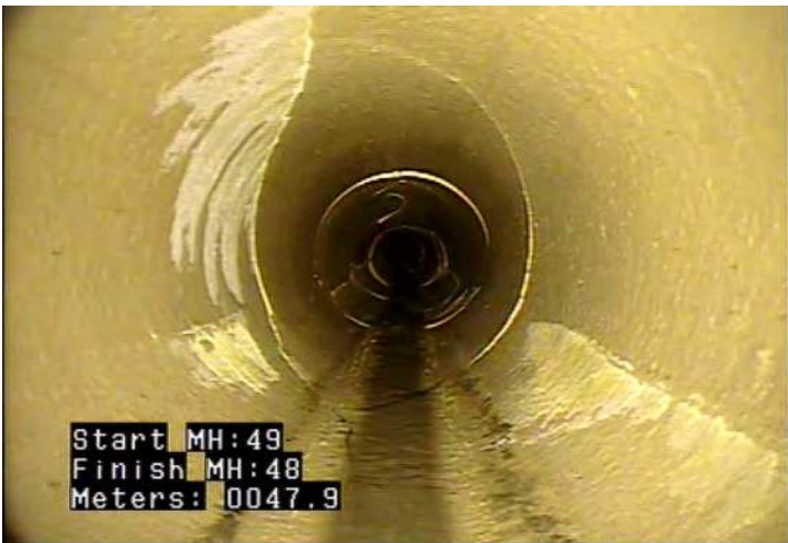
FM - Fracture Multiple @ 47.9 m.
