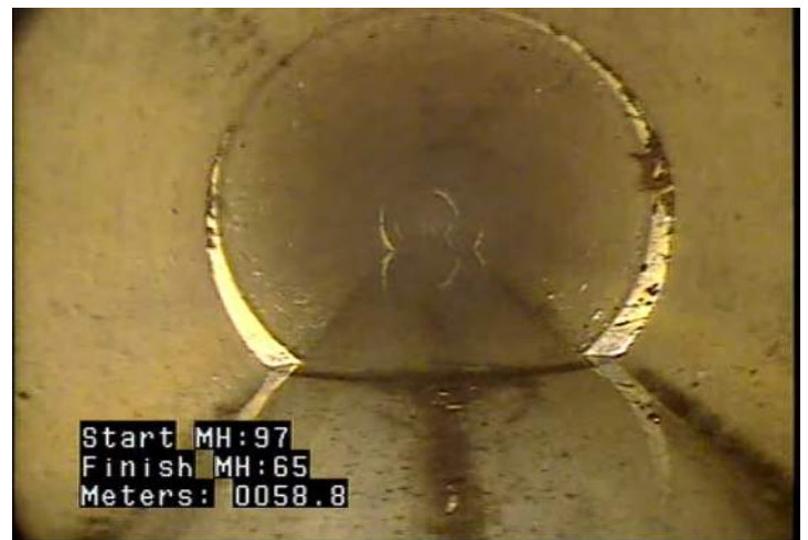
MWLS - Water Level: Sag @ 58.8 m.
