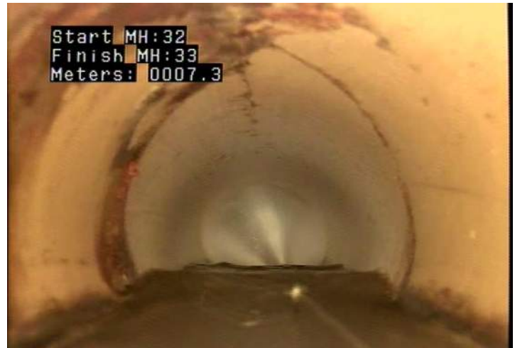
CC - Crack Circumferential @ 7.3 m.
