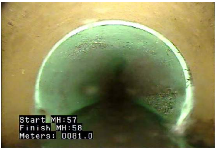
MMC - Material Change @ 81.0 m. Clay tile to PVC
