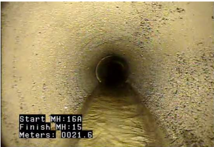
MWLS - Water Level: Sag @ 21.6 m.
