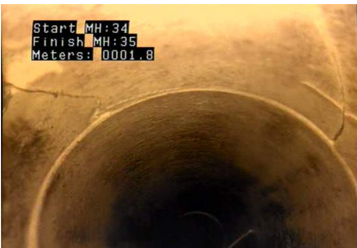
FM - Fracture Multiple @ 1.0 m.
