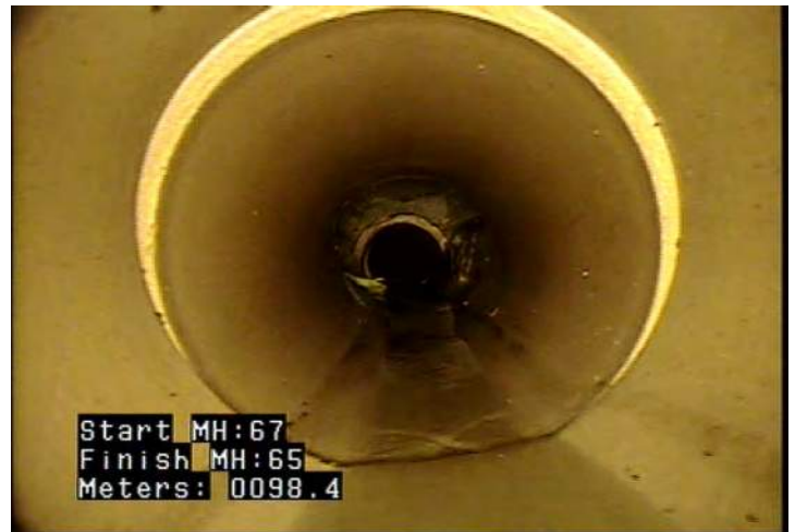
MWLS - Water Level: Sag @ 98.4 m.
