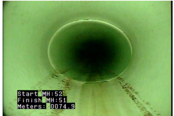
D - Pipe Deformed @ 74.9 m.
