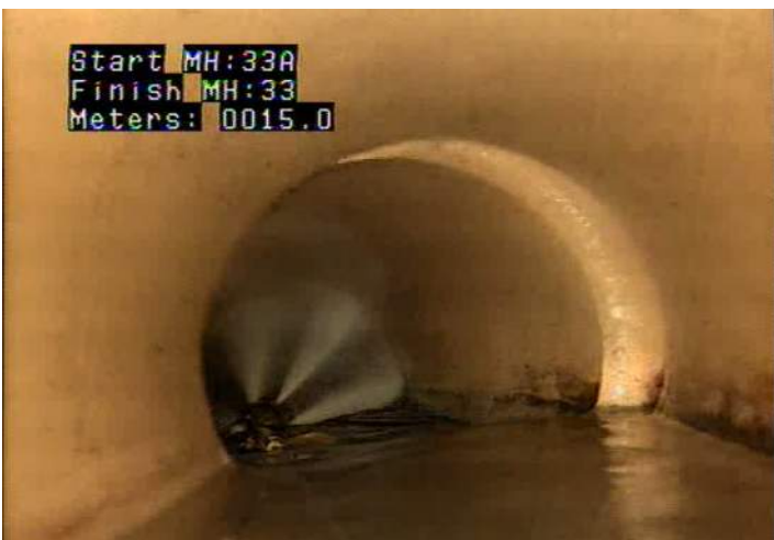
JAL - Joint Angular: Large @ 15.0 m.
