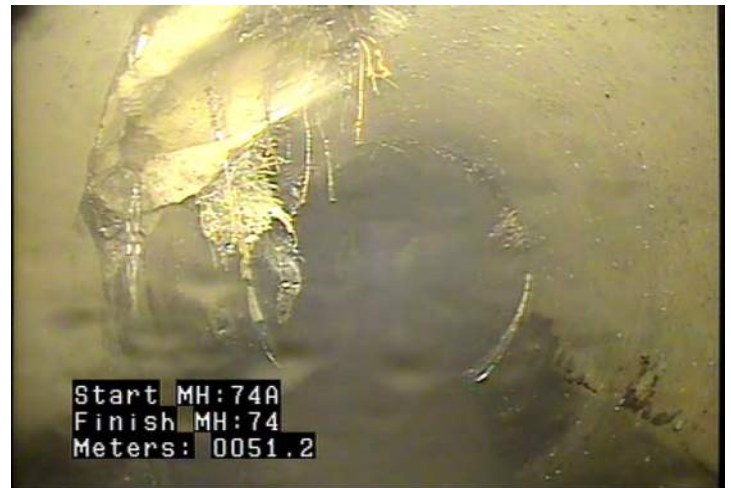
FL - Fracture Longitudinal @ 51.2 m.
