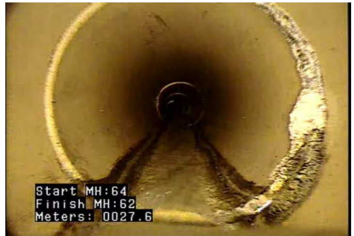
DAE - Deposits Attached: Encrustation @ 27.6 m.
