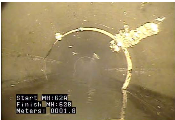
DAGS - Deposits Attached: Grease @ 1.8 m.
