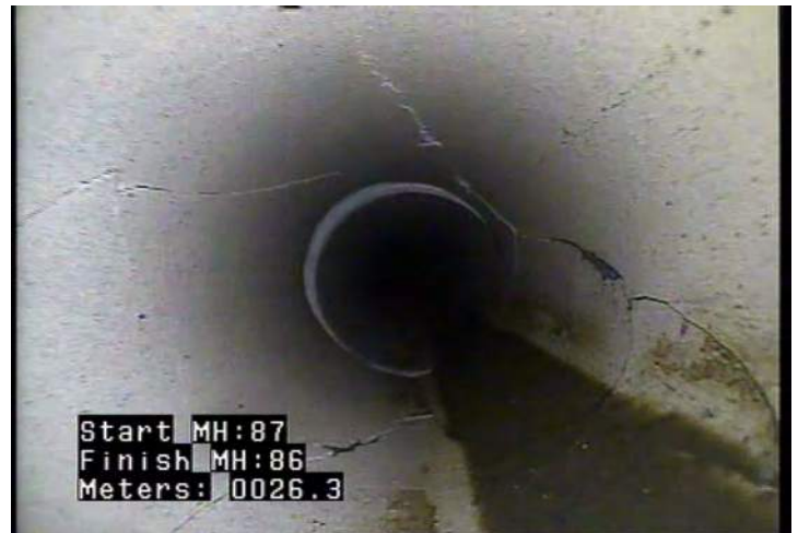
MGP - General Photograph @ 26.3 m. Additional view of multiple fracture
