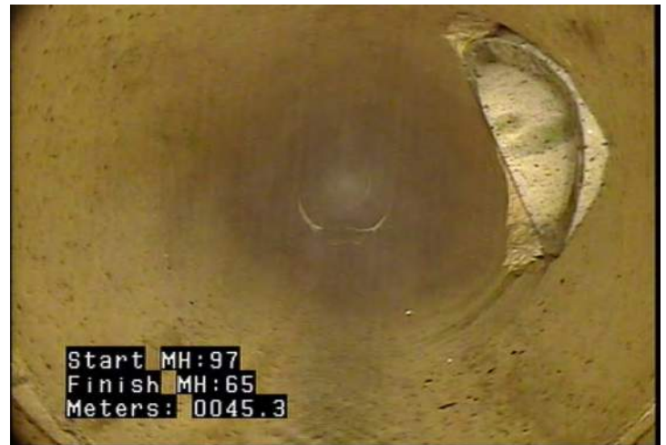
TB - Tap, Break-in / Hammer @ 45.3 m.
