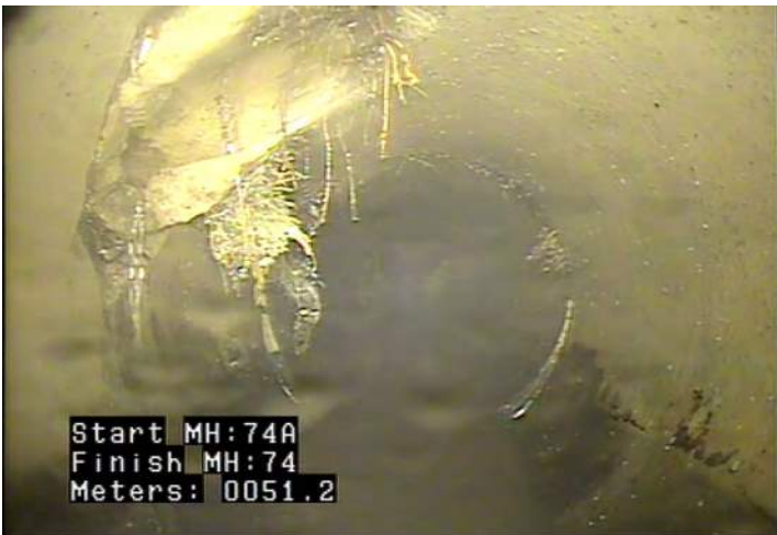
TB - Tap, Break-in / Hammer @ 51.0 m.
