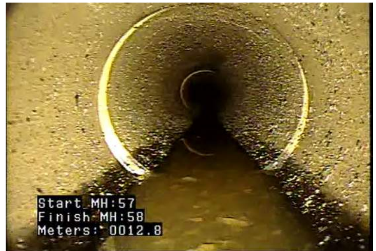
CM - Crack Multiple @ 12.8 m.
