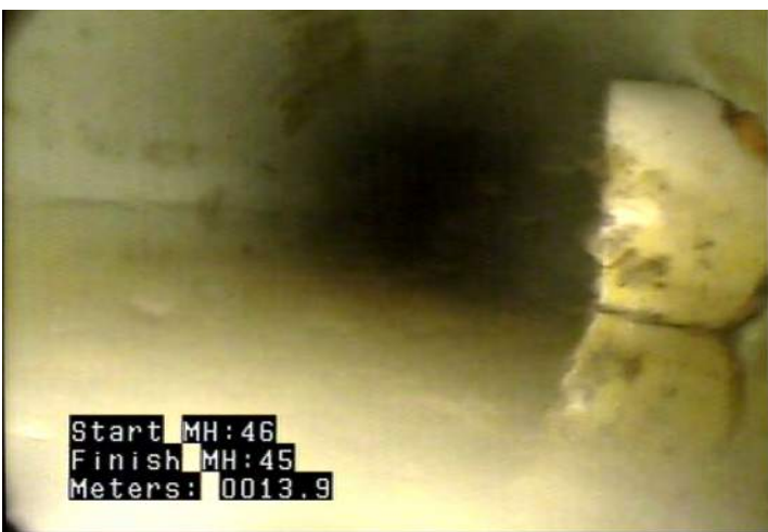
MSA - Survey Abandoned @ 13.9 m. Unable to pass intruding service.
