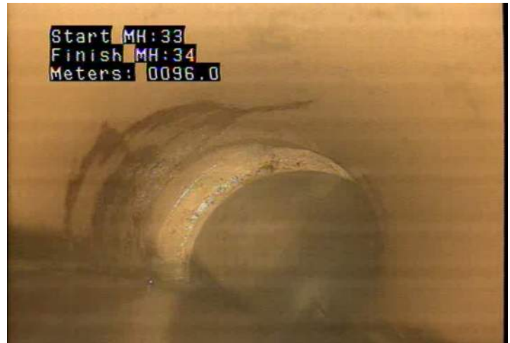
JAM - Joint Angular: Medium @ 96.0 m.
