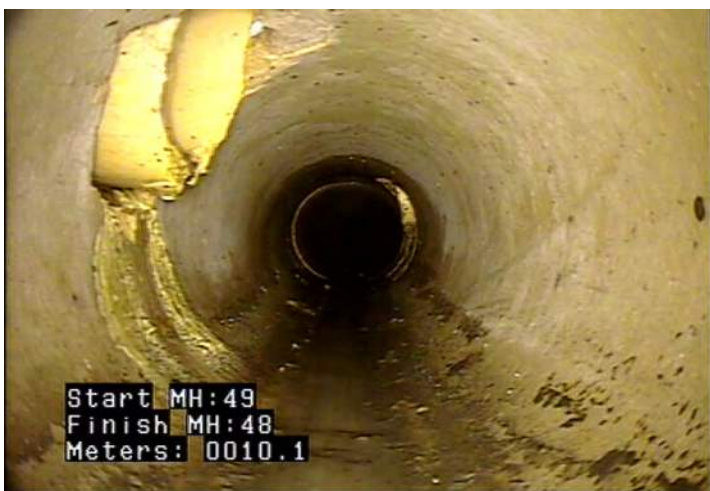
TBI - Tap, Break-in / Hammer: Intruding @ 10.1 m.
