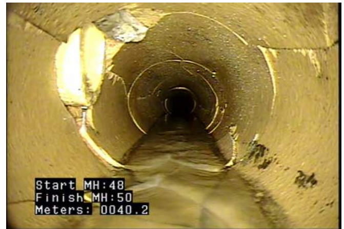
TBD - Tap, Break-in / Hammer: Defective @ 40.2 m. Plastic intruding from top of service.
