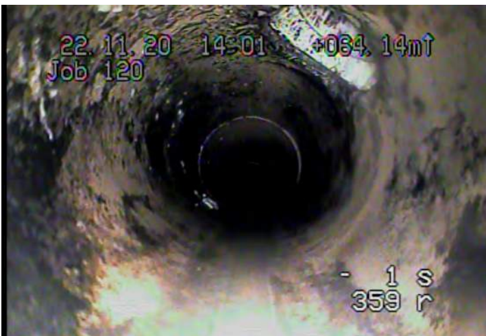
TB - Tap, Break-in / Hammer @ 63.5 m.
