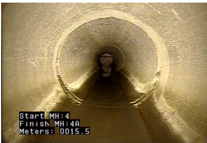
FC - Fracture Circumferential @ 15.5 m.
