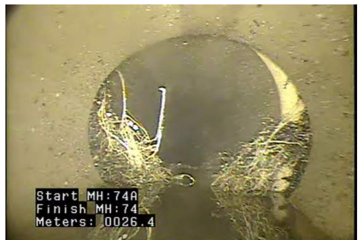
JOL - Joint Offset (displaced): Large @ 26.5 m.
