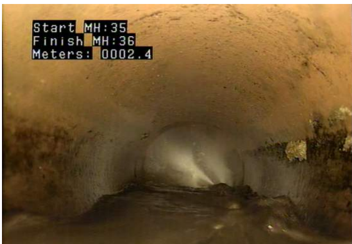
MGO - General Observation @ 2.4 m. Flusher on to reduce flow
