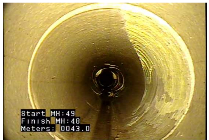
DAE - Deposits Attached: Encrustation @ 43.0 m. Possible hairline crack at 12-1:00
