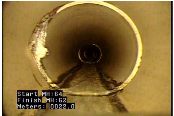
DAE - Deposits Attached: Encrustation @ 22.0 m.
