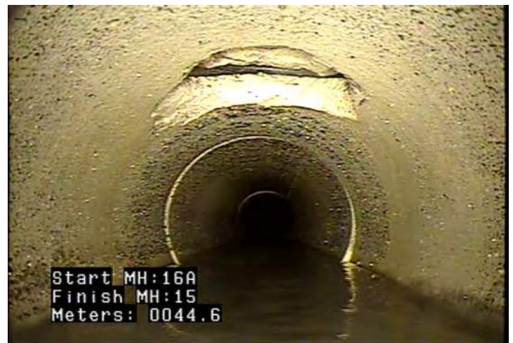
TB - Tap, Break-in / Hammer @ 44.6 m.
