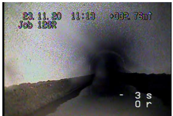
ISGT - Intruding Seal Material - Grout @ 2.3 m.
