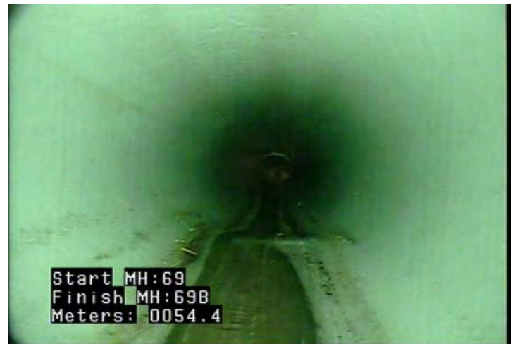
D - Pipe Deformed @ 54.5 m.
