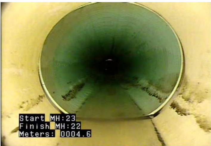
MMC - Material Change @ 4.6 m. White to Blue PVC
