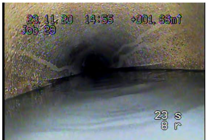
MSA - Survey Abandoned @ 1.6 m. Unable to pass debris in water.
