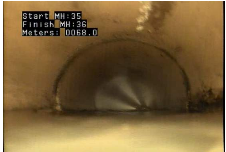
DAE - Deposits Attached: Encrustation @ 68.0 m.
