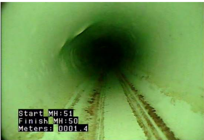
KD - Buckling Dimpling @ 1.4 m.
