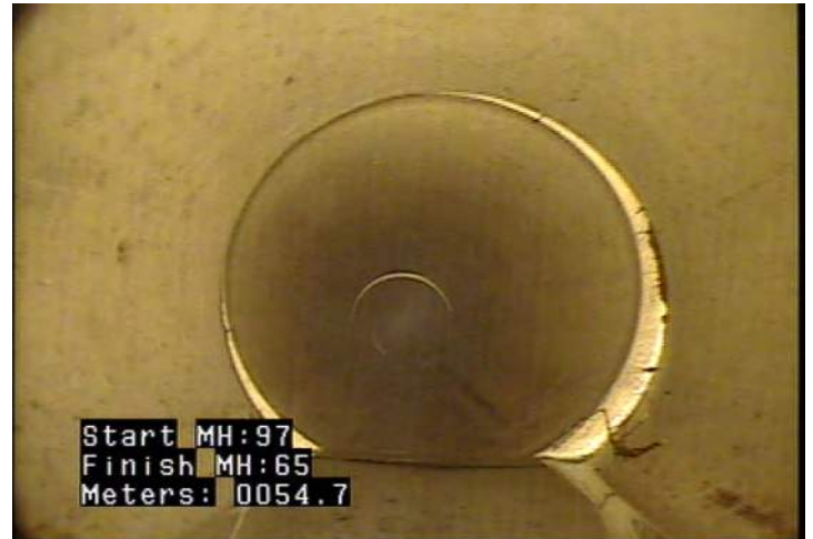
MWLS - Water Level: Sag @ 54.7 m.
