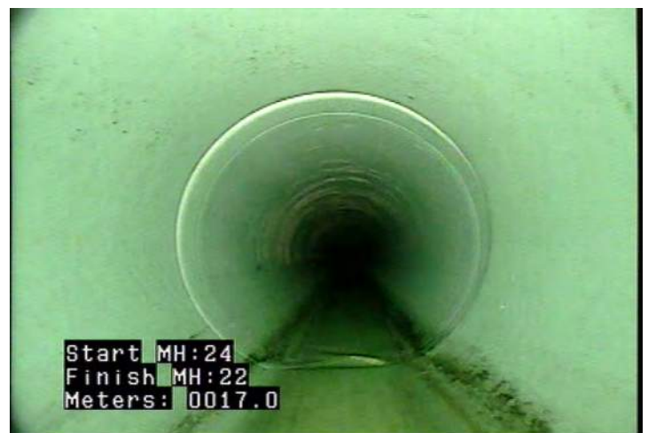
MWLS - Water Level: Sag @ 17.0 m.
