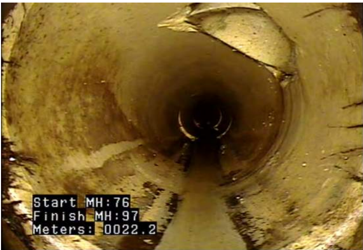
TB - Tap, Break-in / Hammer @ 22.2 m.
