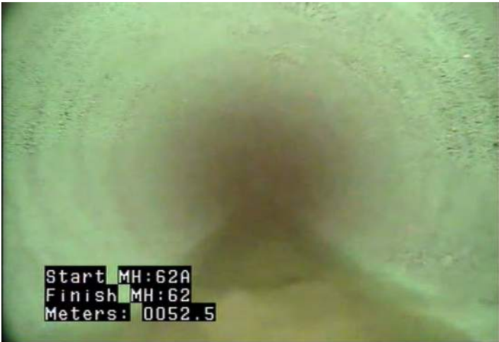
MWLS - Water Level: Sag @ 52.5 m.
