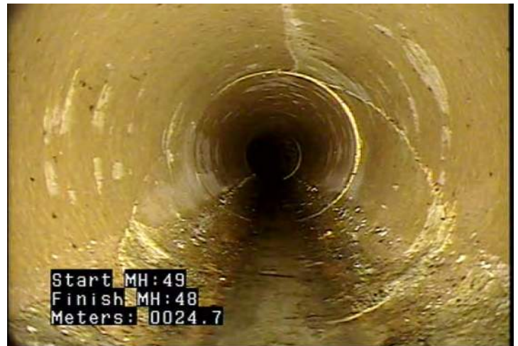
FS - Fracture Spiral @ 24.7 m.
