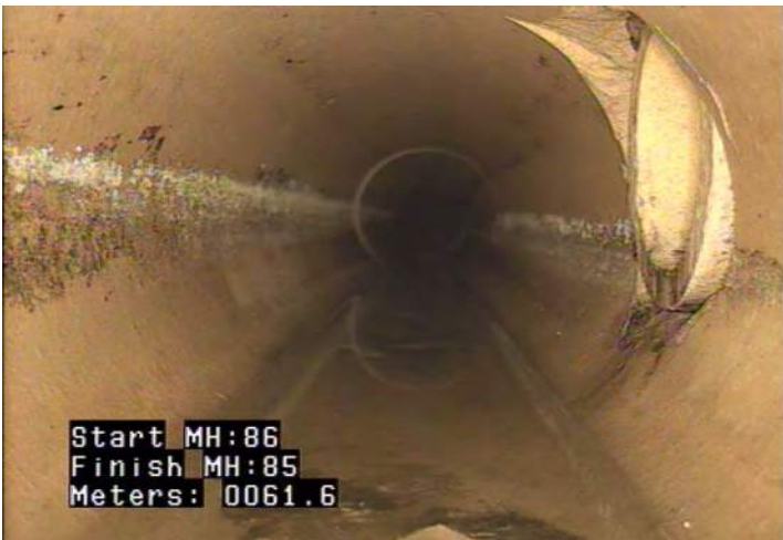
TB - Tap, Break-in / Hammer @ 61.6 m.
