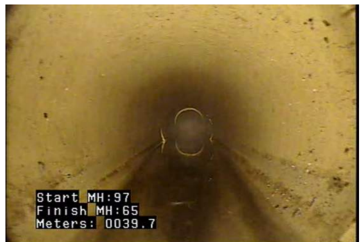
MWLS - Water Level: Sag @ 39.7 m.
