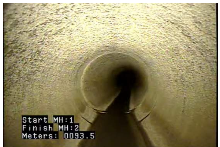
CC - Crack Circumferential @ 93.5 m.
