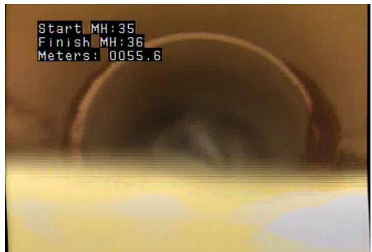
DAE - Deposits Attached: Encrustation @ 55.6 m.
