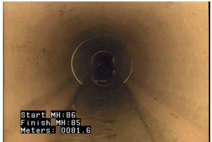
MWLS - Water Level: Sag @ 81.6 m.
