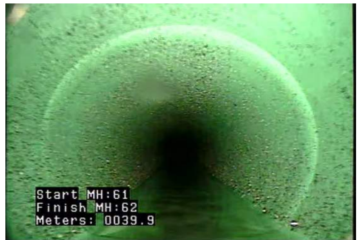
MWLS - Water Level: Sag @ 39.9 m.
