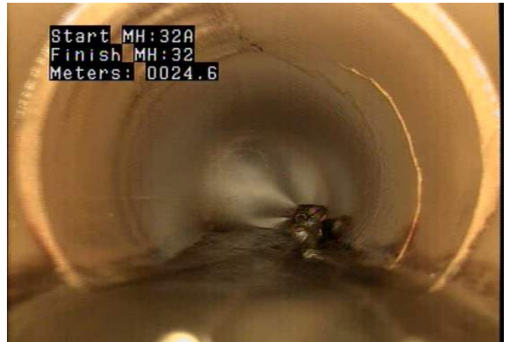
CM - Crack Multiple @ 24.6 m.
