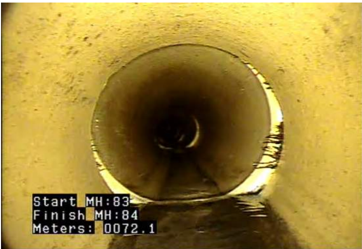
JOM - Joint Offset (displaced): Medium @ 72.1 m.
