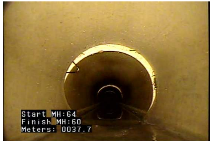
JOM - Joint Offset (displaced): Medium @ 37.7 m.
