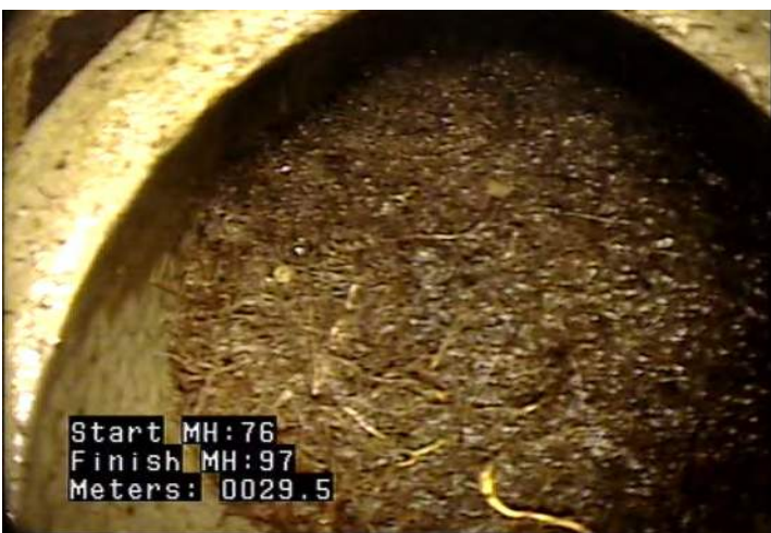
MGP - General Photograph @ 29.2 m. View of root ball inside service
