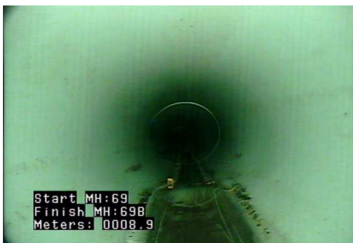
D - Pipe Deformed @ 8.9 m.
