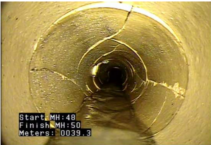
B - Pipe Broken @ 39.3 m.
