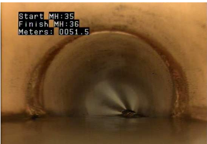
DAE - Deposits Attached: Encrustation @ 51.5 m.
