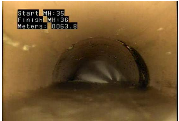
DAE - Deposits Attached: Encrustation @ 63.8 m.
