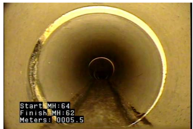
DAE - Deposits Attached: Encrustation @ 5.6 m. Deposits/Encrustation at most joints throughout pipe
