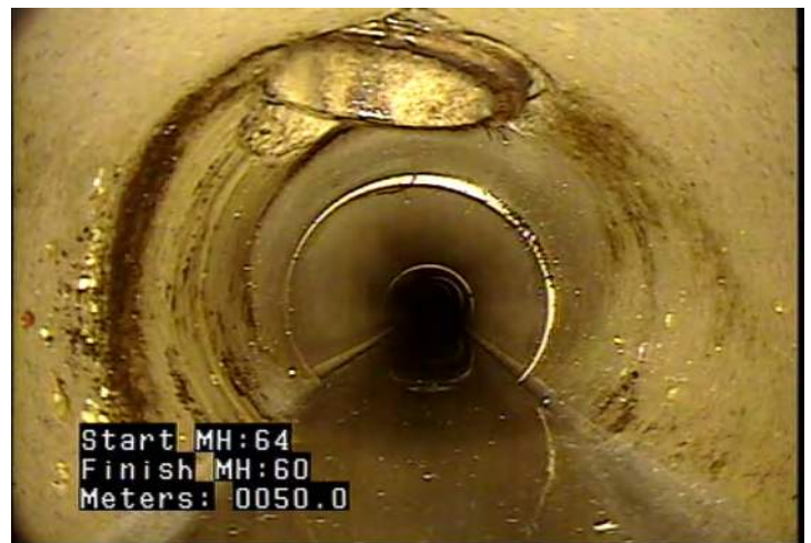
TB - Tap, Break-in / Hammer @ 50.0 m.
