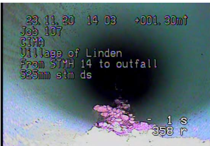
DSGV - Deposits Settled: Gravel @ 0.0 m.
