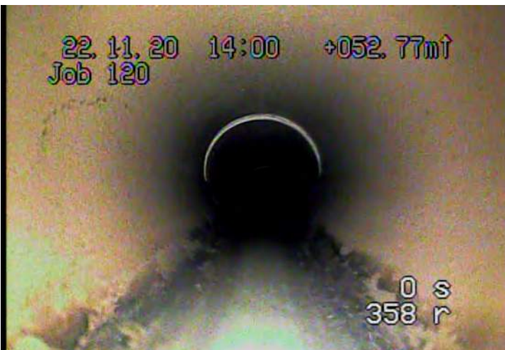
RMJ - Roots, Medium, Joint @ 51.7 m.
