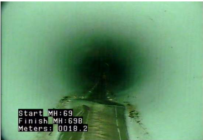
D - Pipe Deformed @ 18.2 m.
