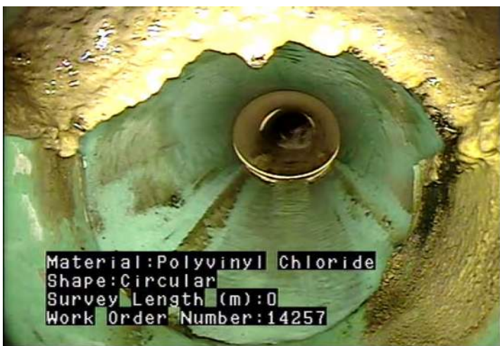
DAE - Deposits Attached: Encrustation @ 0.0 m. At pipe opening
