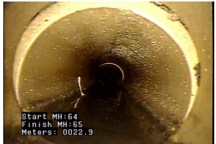
MWLS - Water Level: Sag @ 22.9 m.
