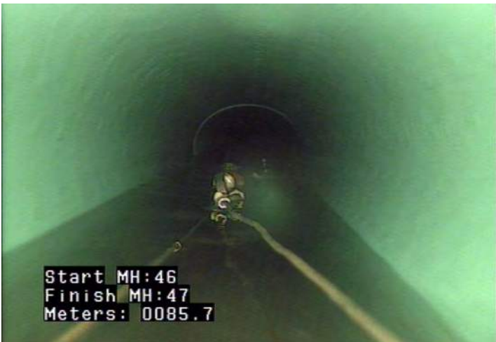
MWLS - Water Level: Sag @ 85.7 m.
