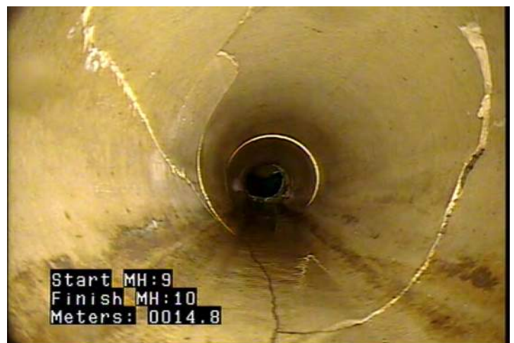
MSA - Survey Abandoned @ 14.8 m. Unable to go over joint with crawler.
