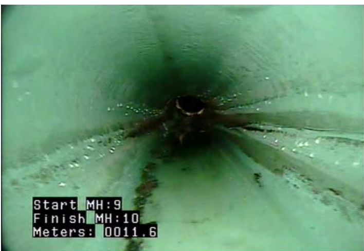
MWLS - Water Level: Sag @ 11.6 m.
