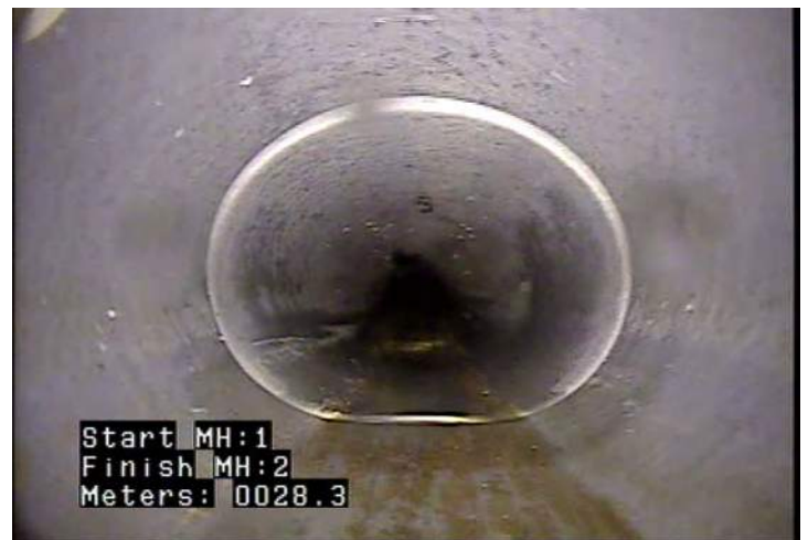
D - Pipe Deformed @ 28.3 m. Pipe oval (visible at joint)
