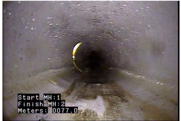
D - Pipe Deformed @ 77.0 m.
