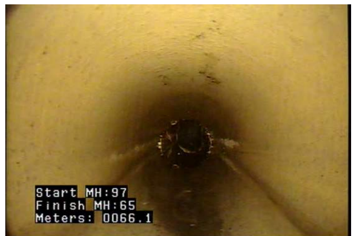
MWLS - Water Level: Sag @ 66.1 m.
