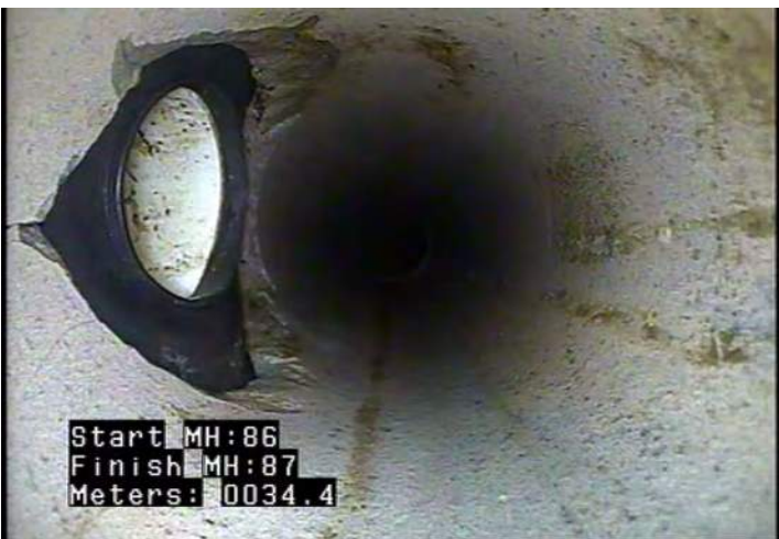
TBD - Tap, Break-in / Hammer: Defective @ 34.4 m. Hole overcut
