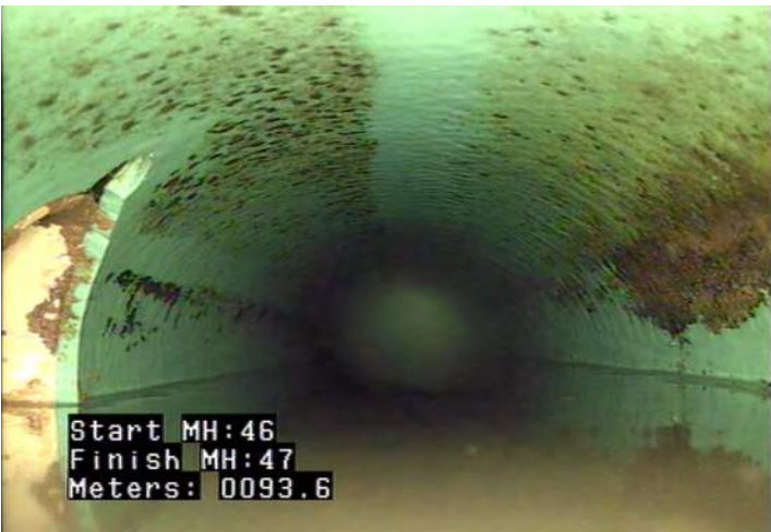
TSD - Tap, Saddle: Defective @ 93.6 m. Pipe chipped above service.
