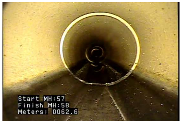
FS - Fracture Spiral @ 66.9 m.
