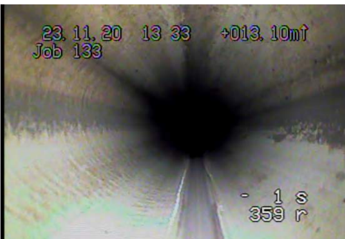
JOL - Joint Offset (displaced): Large @ 10.8 m.
