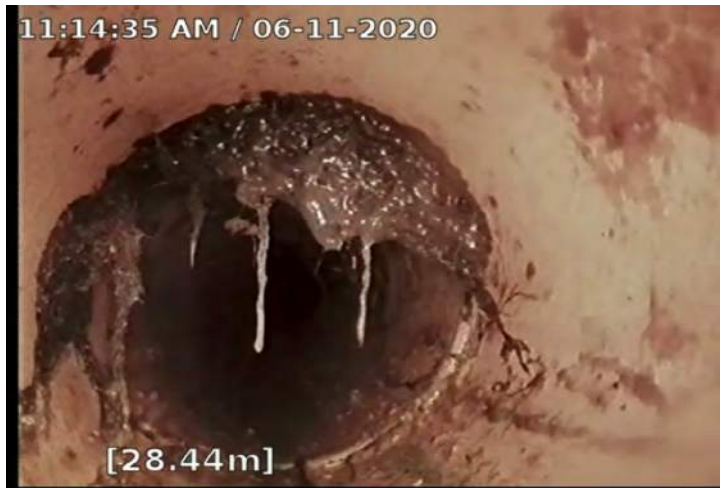
RMJ - Roots, Medium, Joint @ 28.4 m.
