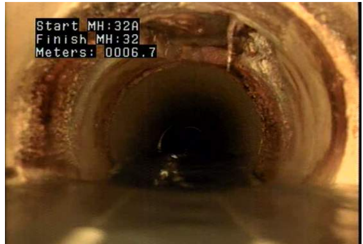
RPPD - Point Repair - Patch Repair: Defective @ 6.7 m. Leaking
