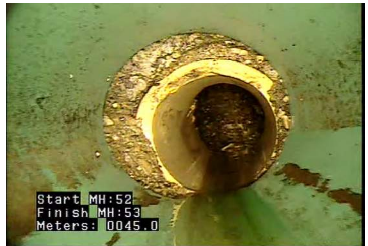
MGO - General Observation @ 0.0 m. Concrete patch repair
