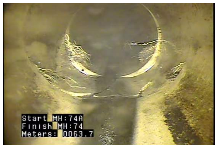
MGP - General Photograph @ 63.7 m. Additional view of break
