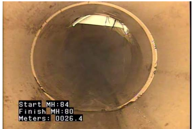
RFC - Roots, Fine: Connection @ 26.4 m.
