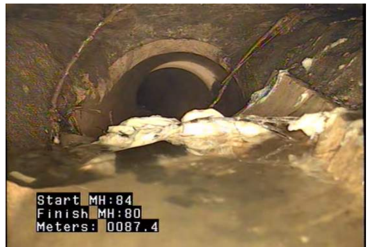
AMH - Access Point - Manhole @ 87.4 m. S MH 80
