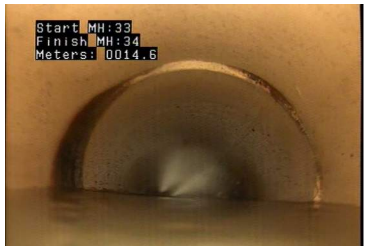
DAE - Deposits Attached: Encrustation @ 14.6 m.
