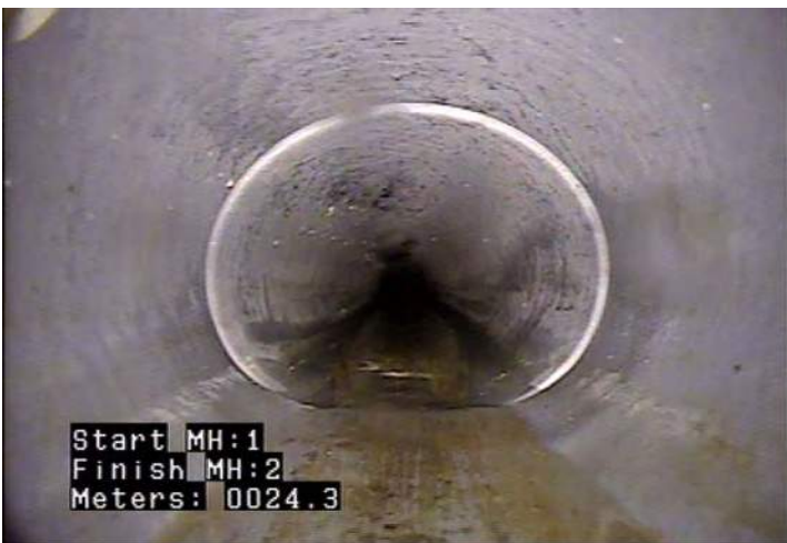
D - Pipe Deformed @ 24.3 m. Pipe oval (visible at joint)
