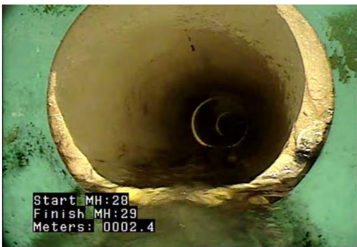
JOM - Joint Offset (displaced): Medium @ 2.4 m.
