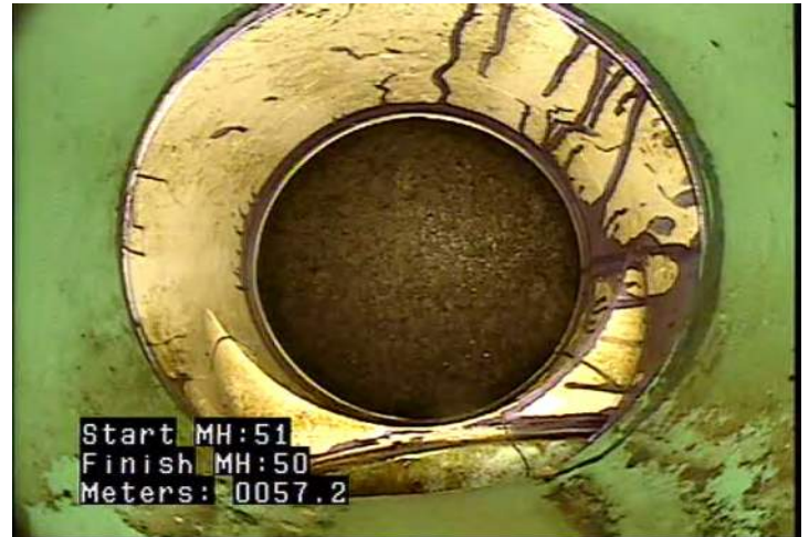
TF - Tap, Factory Made @ 57.2 m. Drop structure
