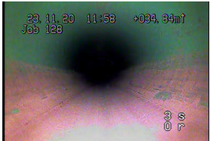
DSGV - Deposits Settled: Gravel @ 33.3 m.
