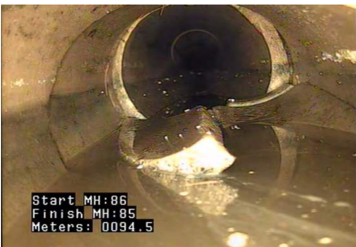
MSA - Survey Abandoned @ 94.5 m. Unable to pass broken pipe
