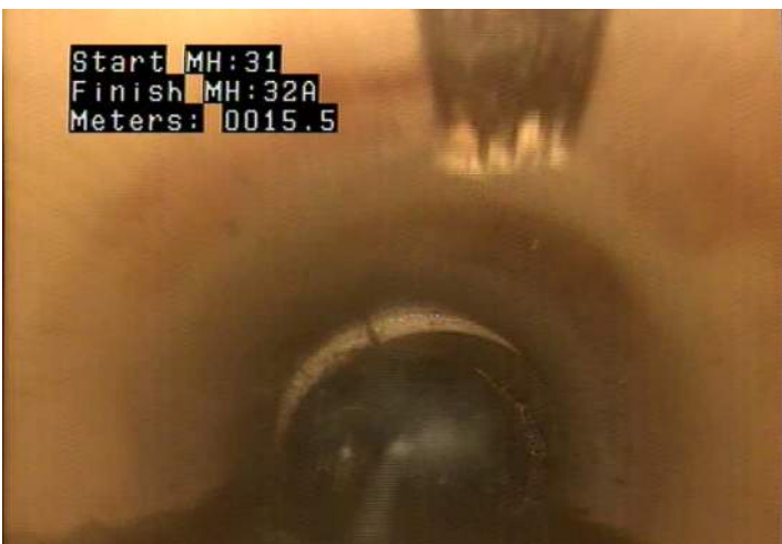
H - Hole in Pipe @ 15.5 m. Hole cut
