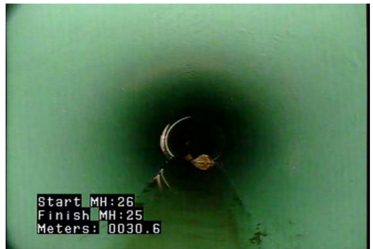
MWLS - Water Level: Sag @ 30.6 m.
