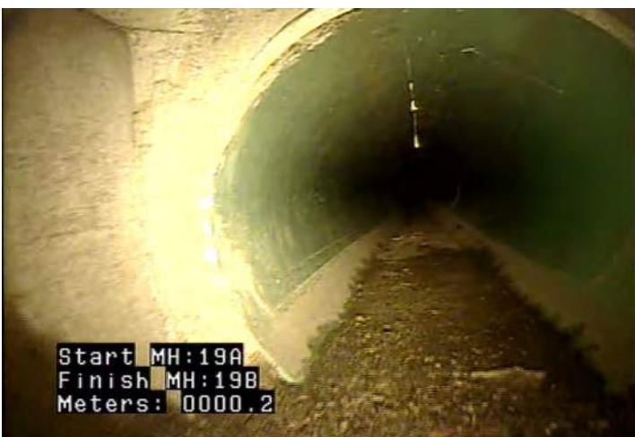
DSGV - Deposits Settled: Gravel @ 0.2 m.
