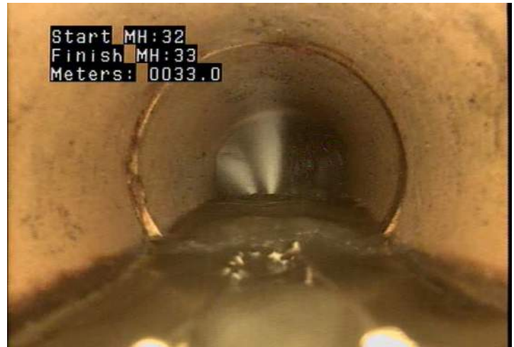
DAE - Deposits Attached: Encrustation @ 33.0 m.
