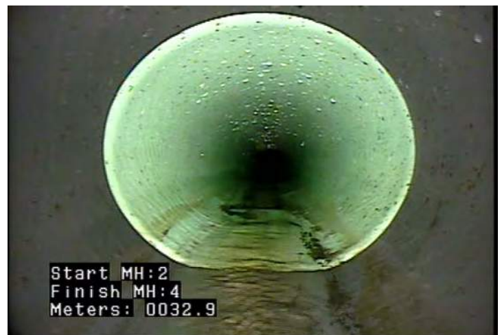
MMC - Material Change @ 32.9 m. Grey PVC to Blue PVC
