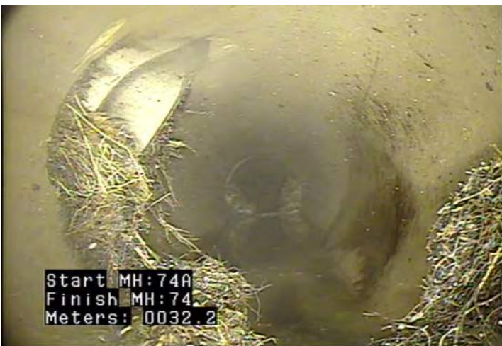
TB - Tap, Break-in / Hammer @ 32.2 m.
