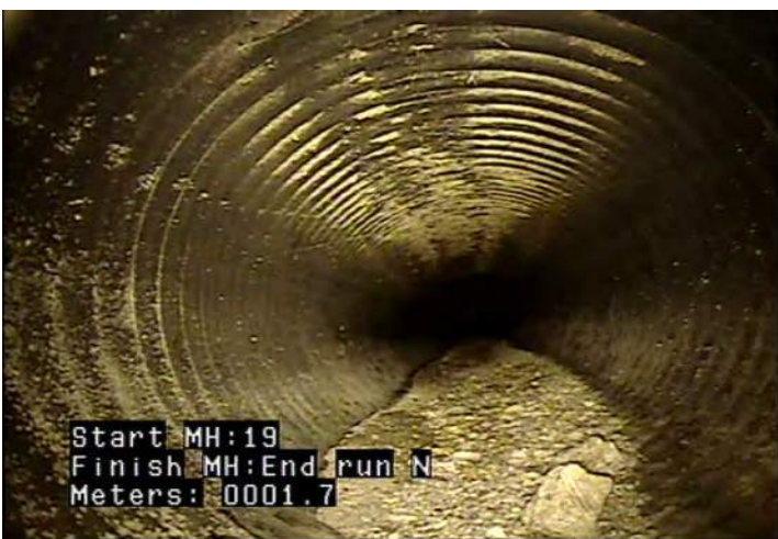
DSGV - Deposits Settled: Gravel @ 0.5 m.
