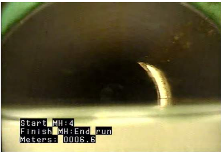
MMC - Material Change @ 6.6 m. Blue PVC to Grey PVC
