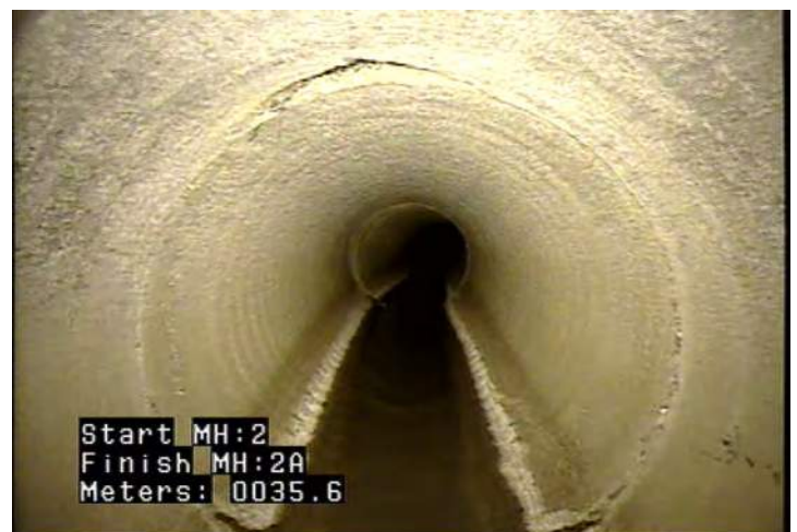
MGO - General Observation @ 35.6 m. Chipped joint
