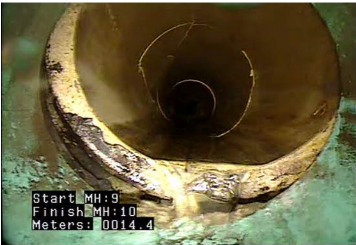
MMC - Material Change @ 14.4 m. PVC to Clay tile
