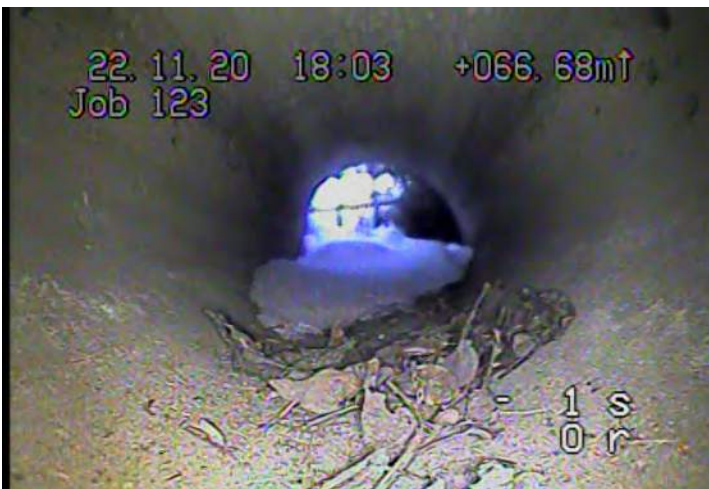
MMC - Material Change @ 66.4 m. PVC to Concrete
